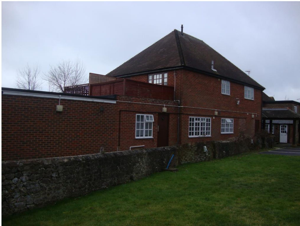
2.2 North elevation to hotel access drive. Site is in foreground.
