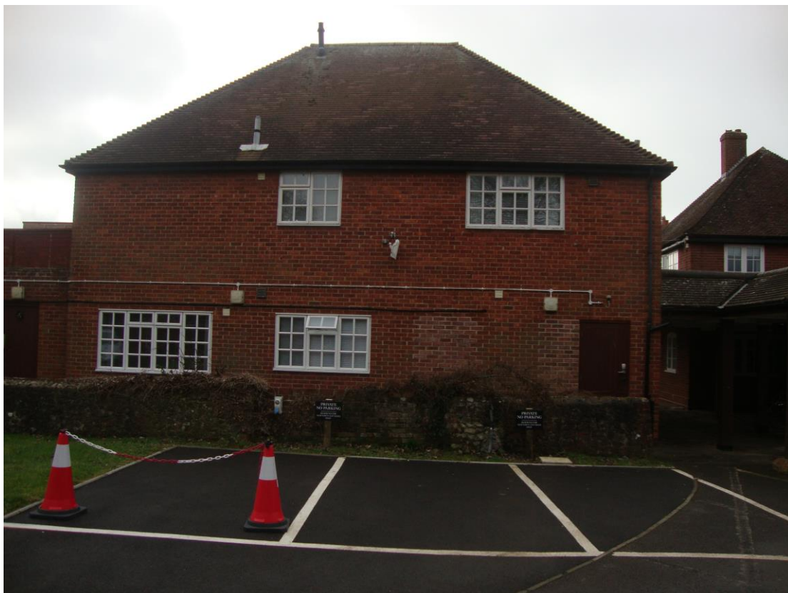
2.3 North elevation viewed from hotel access drive.
