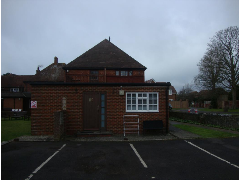
2.1 East elevation showing existing building with flat roof and terrace accessible from first floor guest rooms.
