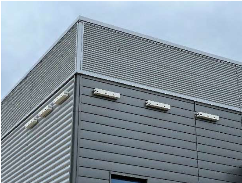
Genesis swift nest boxes attached to a new industrial unit in Cambridgeshire
