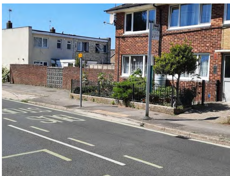
Photograph 6.3: Raised Kerbs at Wakefords Way Bus Stop
