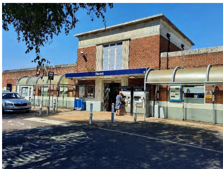
Photograph 4.8: Havant Railway Station
