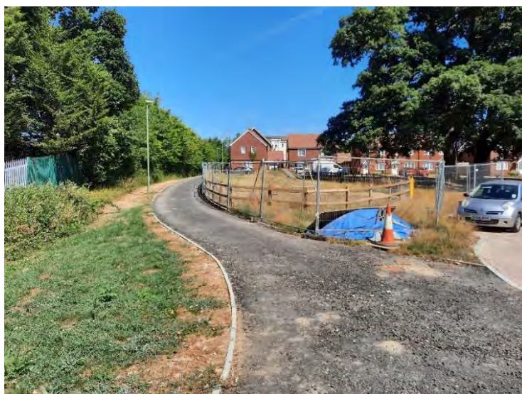
Photograph 6.1: Footpath that runs along the western and north-western edge of Brookvale
