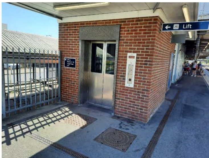
Photograph 6.6: Lifts Located on each Platform of Havant Railway Station
