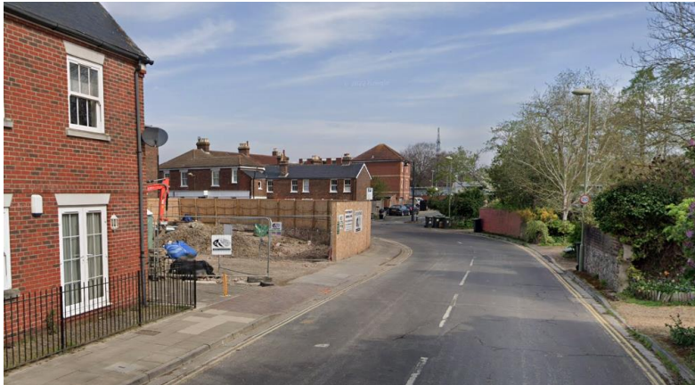
Fig 4: Residential construction within the area (Prince George Street) adjoining to North Street.
