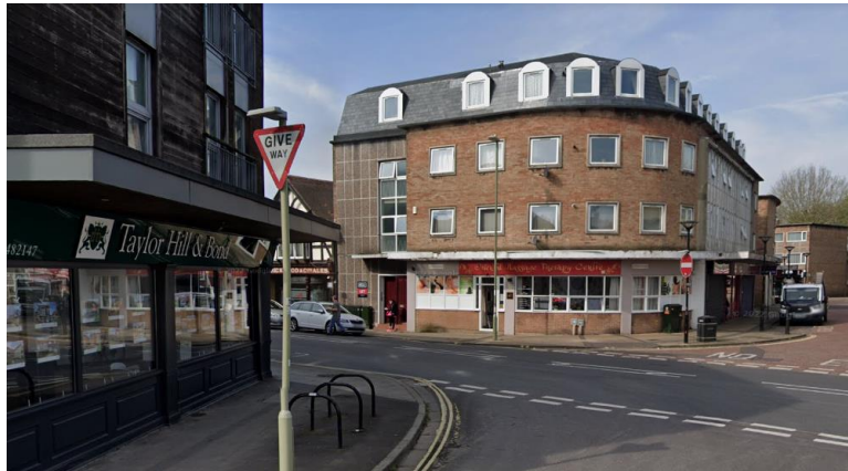
Fig 5 Adjacent 4 storey building
