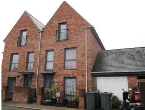
Fig 1 – View of the front of the property.
