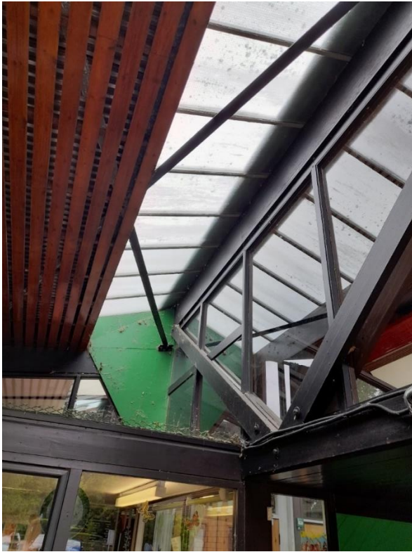
Fig 6. Interior view of the school showing the feature glulam beams and rooflights.
