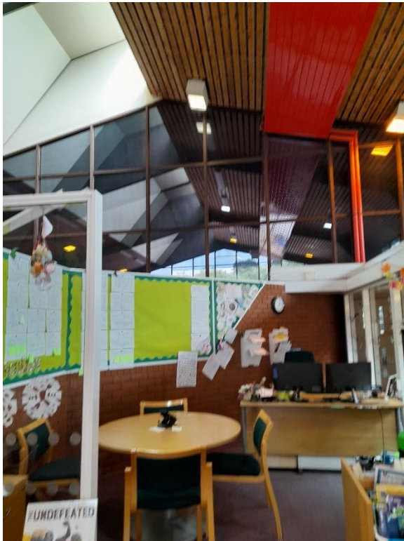
Fig 7. Interior view of the school showing the feature timber soffit ceiling with feature red ceiling radiant panel.
