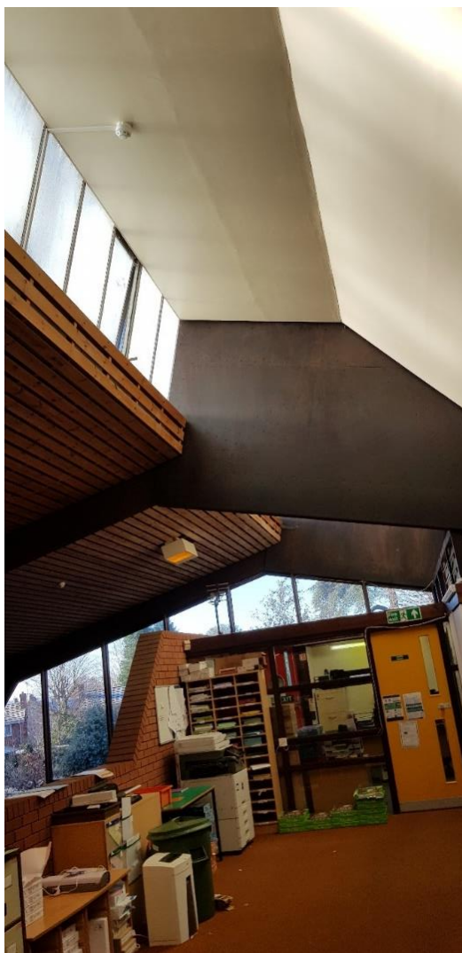
Fig.5 Interior view of the school showing the feature glulam beams and timber slat ceiling
