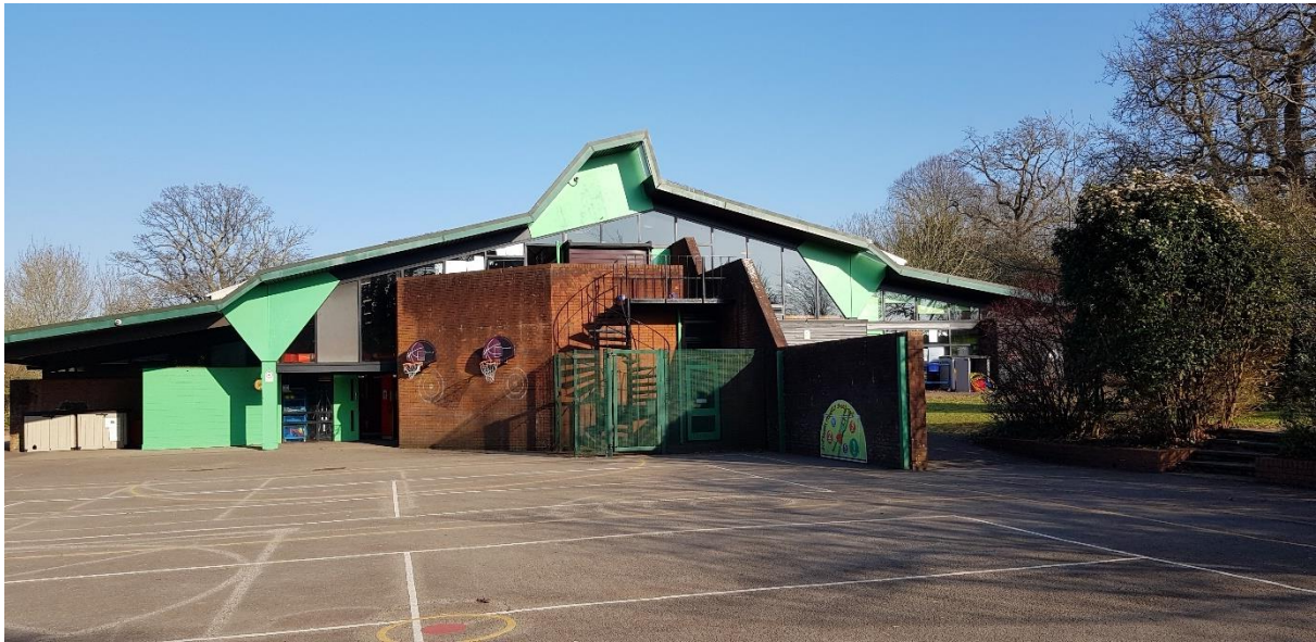
Fig 3. West Elevation showing the feature 'floppy hat' roof.
