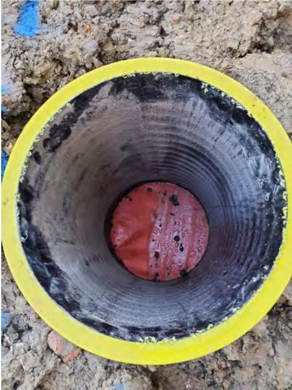
Plate 13 – View of high visibility membrane installed beneath subsoil
