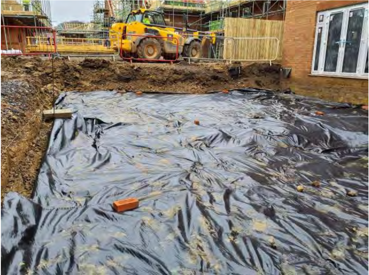
Plate 6 – View of reduced dig and black geotextile in Plots 111-112
