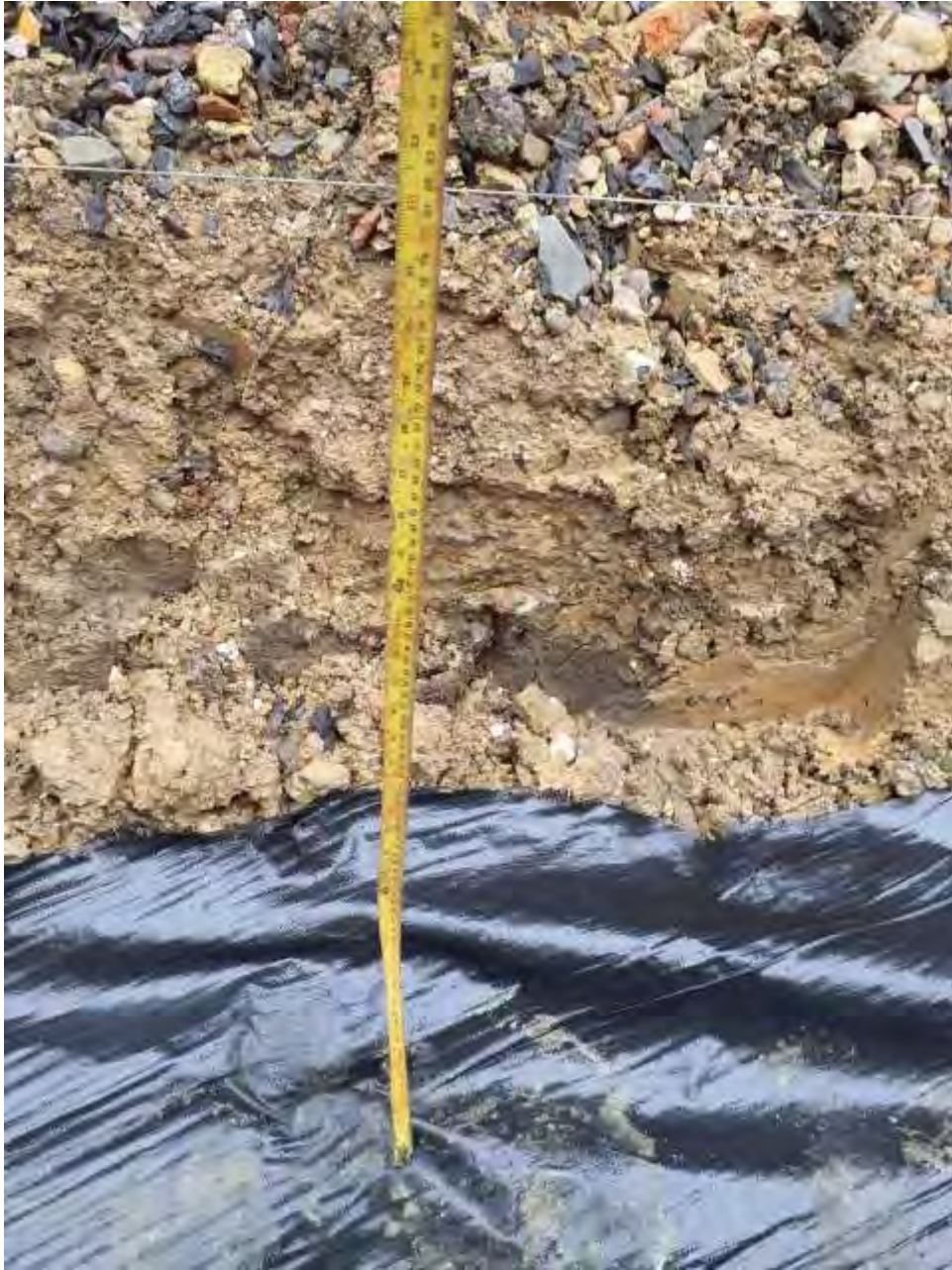
Plate 8 – Depth of reduced dig
