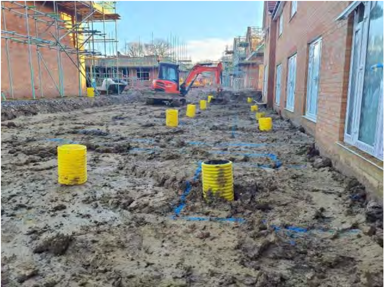
Plate 10 – View of subsoil installed across Plots 108-112
