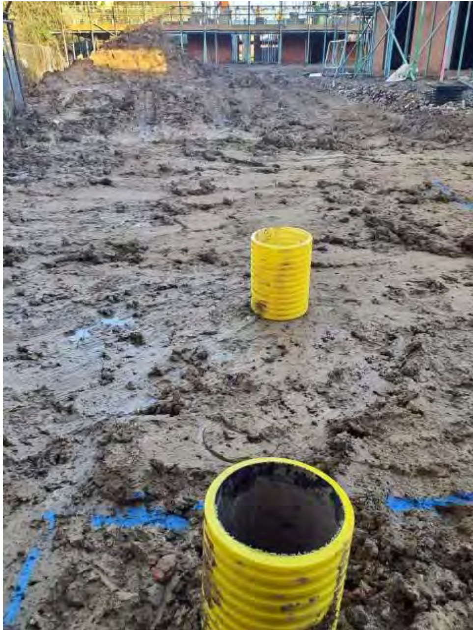
Plate 12 – View of subsoil installed in Plot 108
