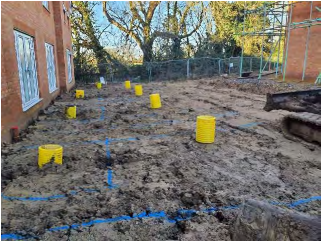
Plate 9 – View of subsoil installed across Plots 108-112
