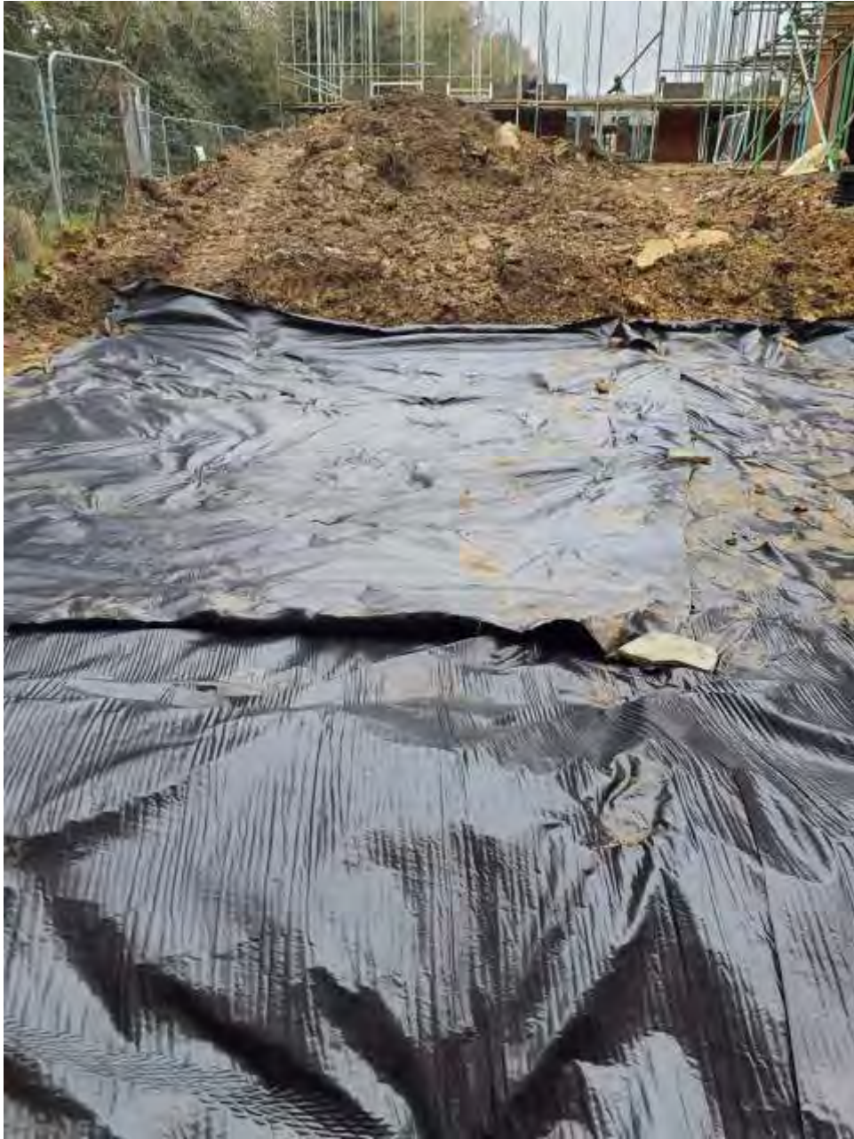
Plate 3 – Reduced dig and black geotextile in Plot 108
