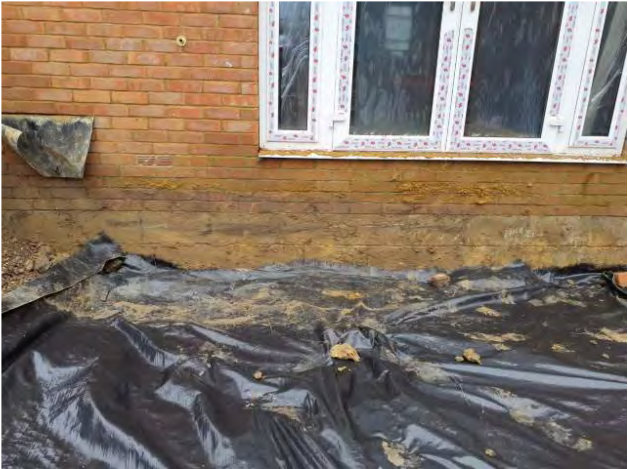
Plate 7 – View of reduced dig and black geotextile in Plot 112
