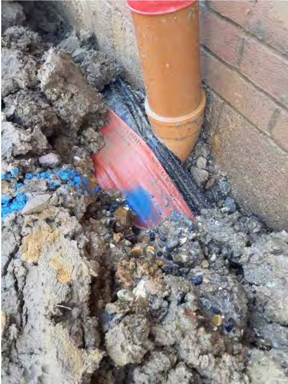
Plate 11 – View of black geotextile and high visibility geotextile beneath subsoil
