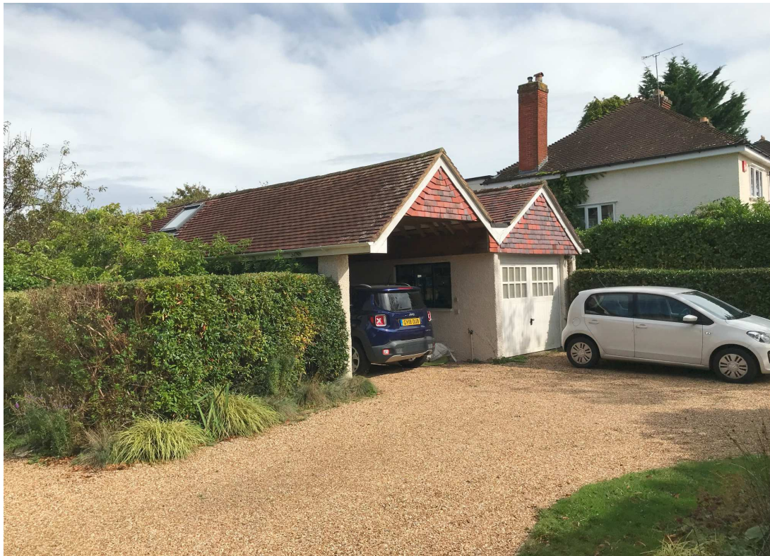
View from the front looking east existing garage / studio block
