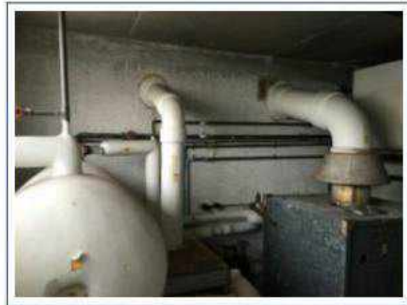
View of ACM lagging and pipework in M&Co. Boiler room
