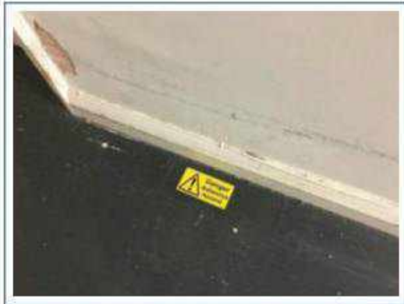
View of vinyl floor tiles in M&Co.
