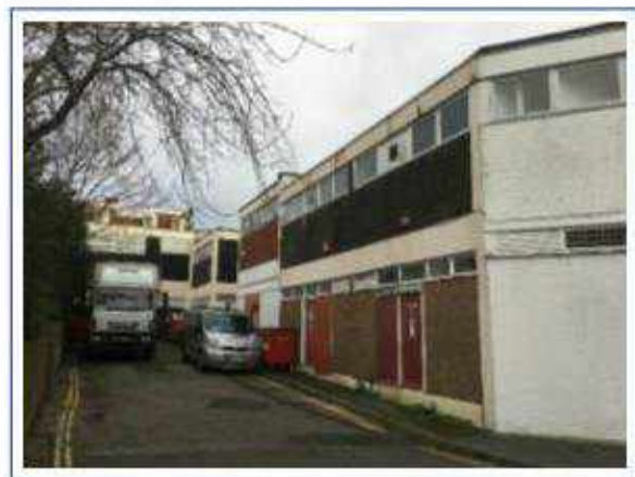
Tradesman entrance behind north western block
