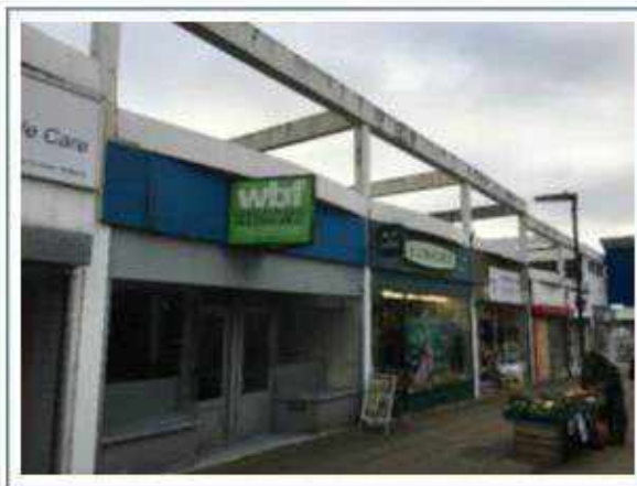
Retail units and view of concrete frame
