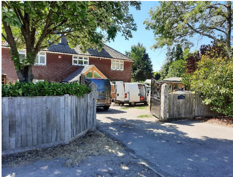
Photograph 2.4: The Laurels, located to the north of the proposed development
