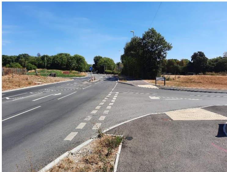
Photograph 2.1: Bartons Road looking east at the junction with Normandy Way
