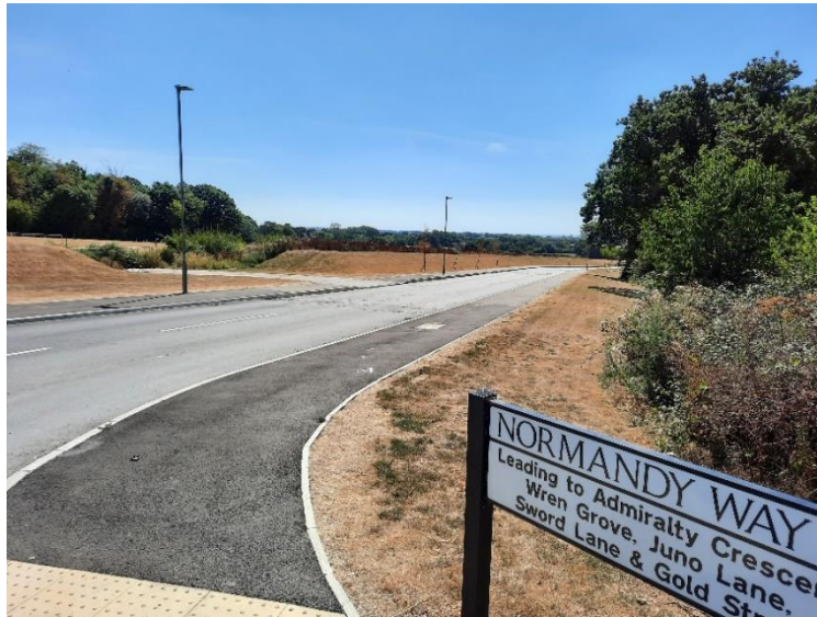
Photograph 2.2: Normandy Way looking south from Bartons Road towards the proposed site access
