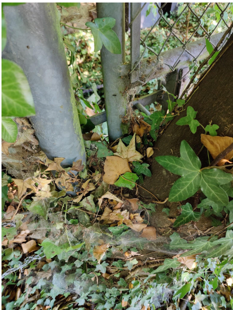
T017: Tree has grown around gate and gate post - unable to be removed and or opened
