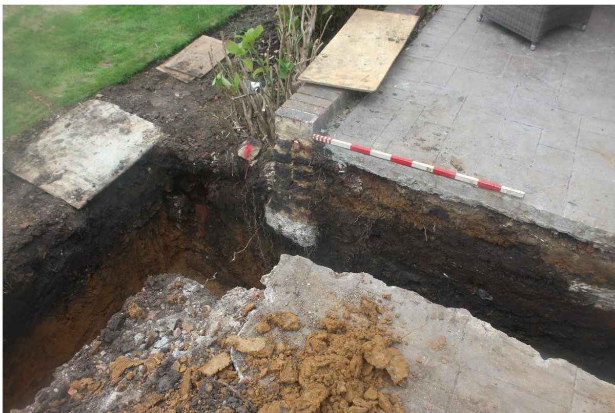
Plate 4. North facing section of southern trench, showing patio wall and rubble soakaway (left), looking southeast. 1m scale.
