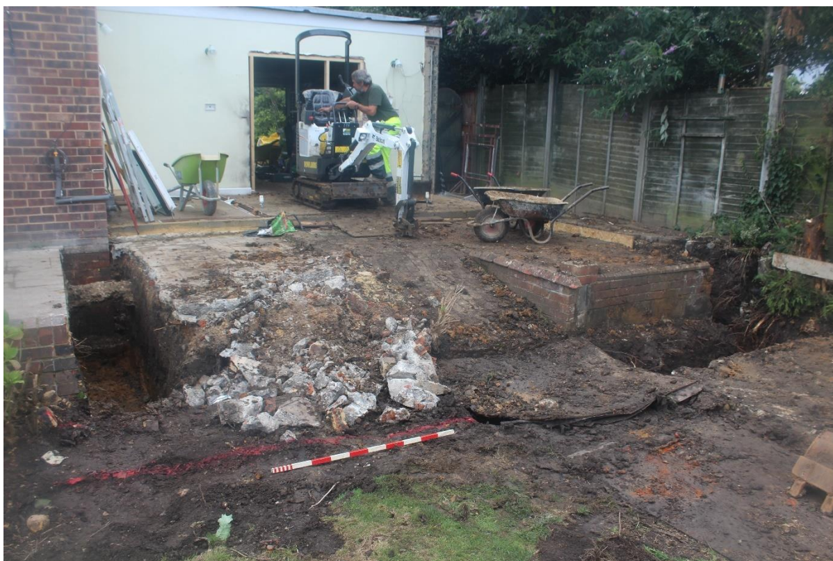
Plate 5. Site shot taken partway through the works, Looking northwest. 1m scale.
