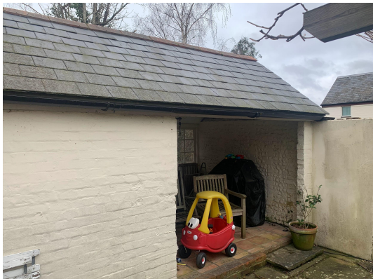
Another view showing the outdoor store area. This opening would be infilled with glazed doors to form an entrance to the office.
