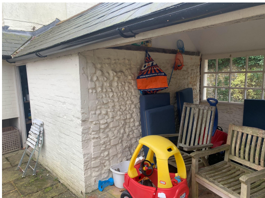
View of the outdoor store area. This is the open back half of the storage area currently used for garden storage.
