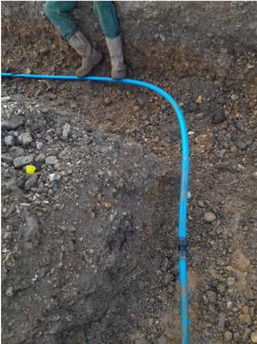
Figure 21 – Main Water (Barrier Pipe).
