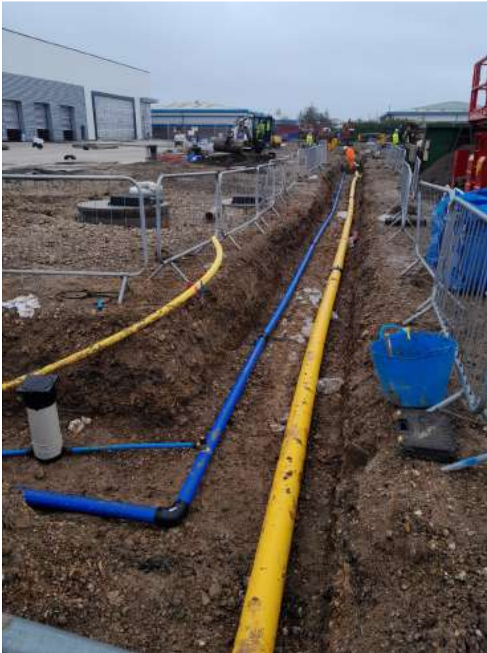
Figure 22 – Main Water (Barrier Pipe).
