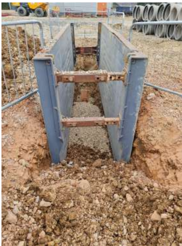
Figure 14 – Ongoing drainage works
