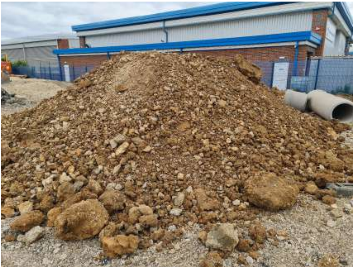
Figure 13 – Stockpiled drainage arisings
