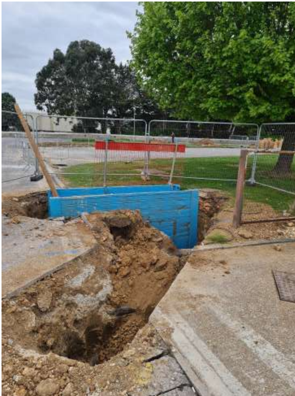
Figure 16 – Drainage work in and around WS2
