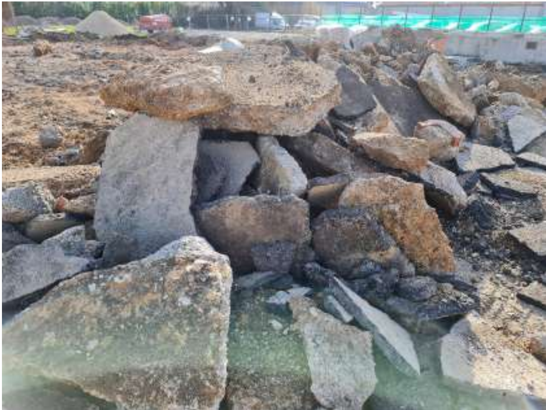
Figure 10 – Oversize and concrete for crushing (NE)
