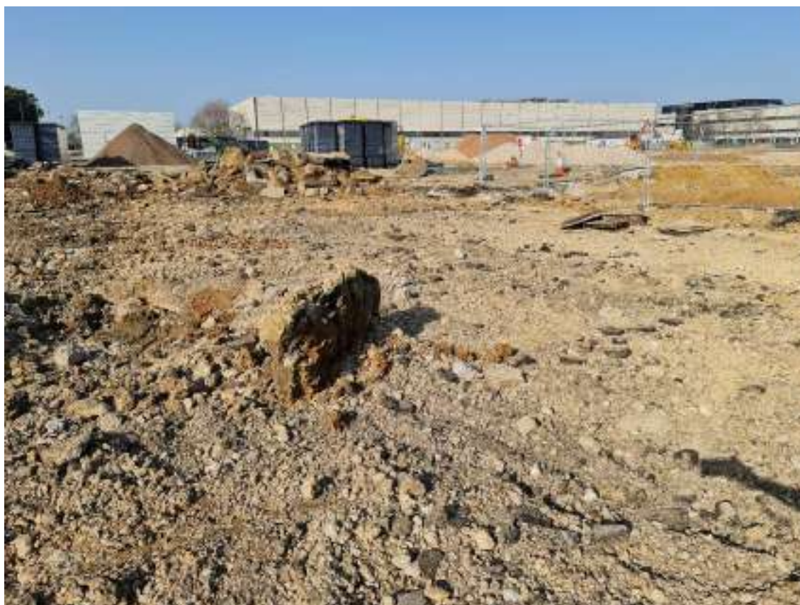
Figure 7 – Southwest development platform - Hardstanding and topsoil removed
