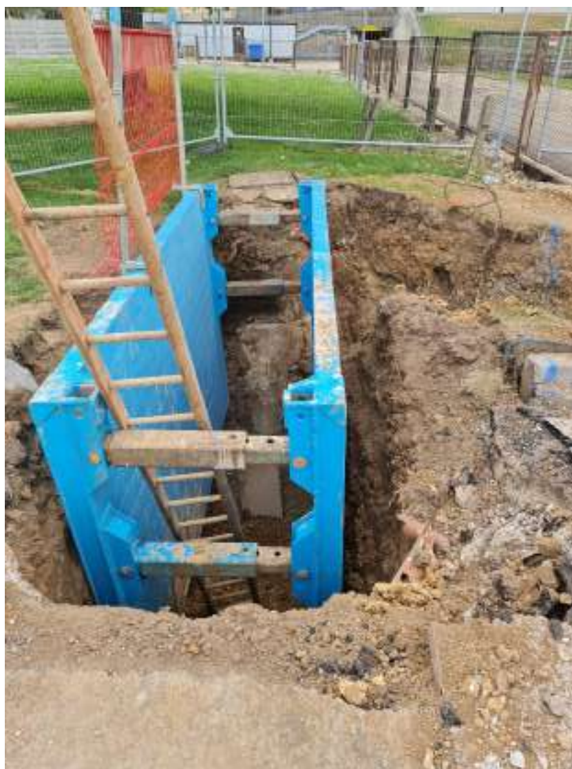
Figure 15 – Drainage work in and around WS2
