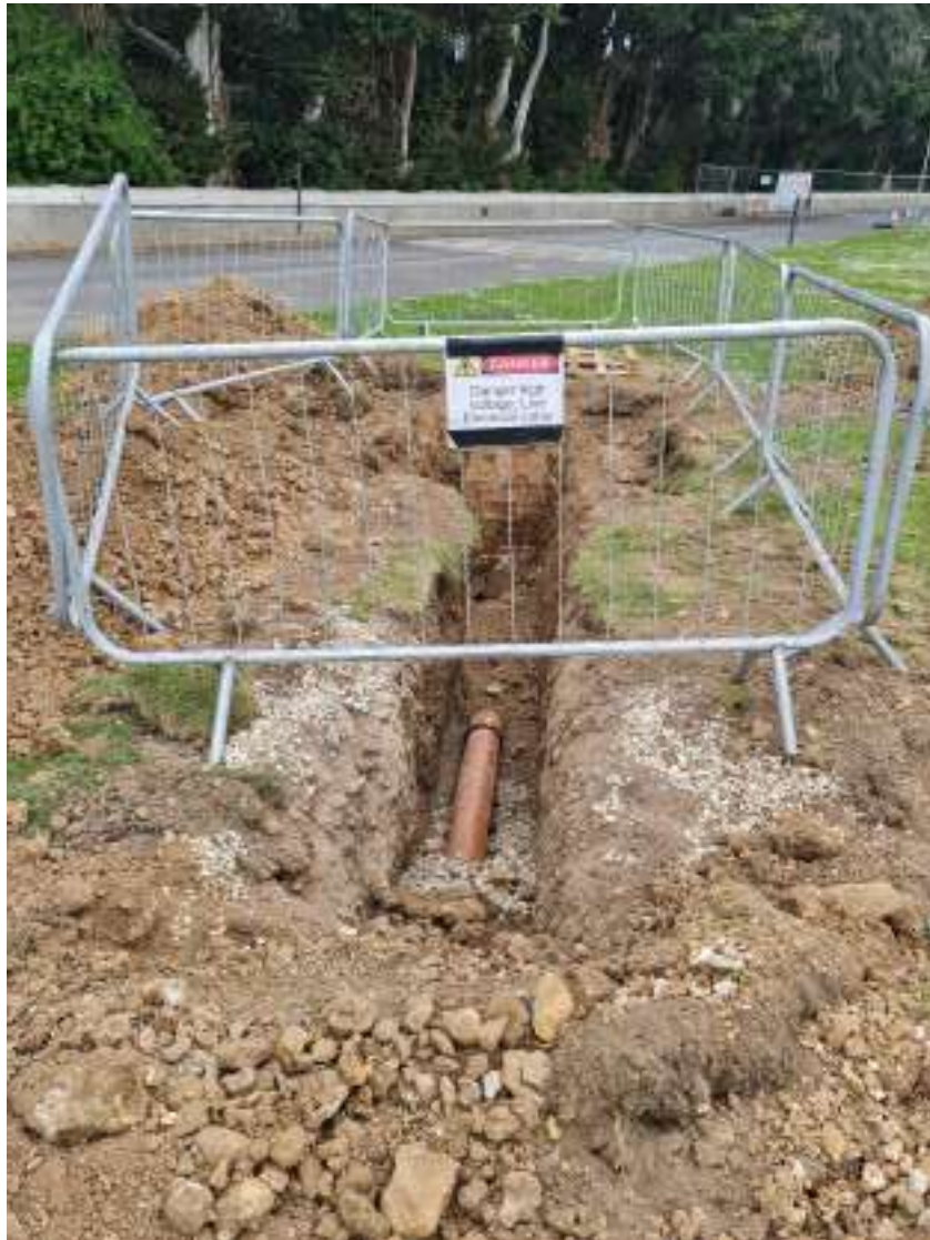
Figure 19 – Drainage work in and around WS2
