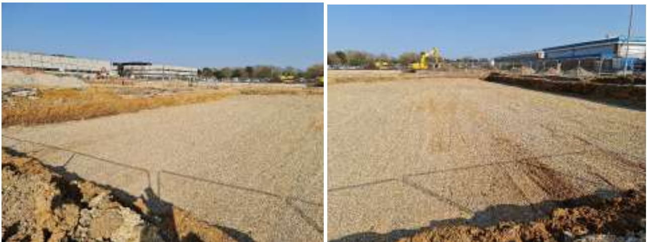
Figure 9 – Attenuation tanks (resulting in mostly natural soils)
