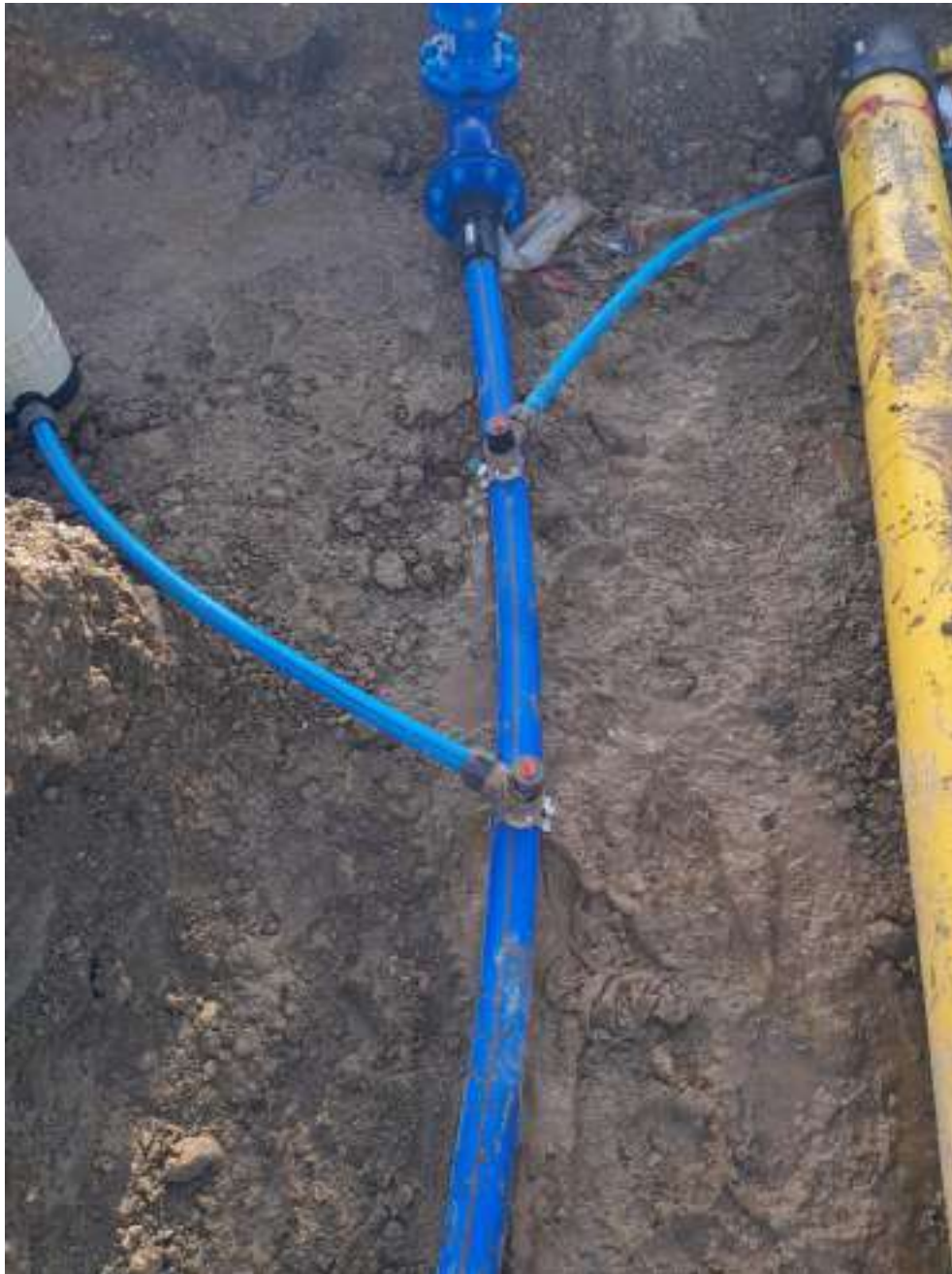
Figure 20 – Main Water (Barrier Pipe).
