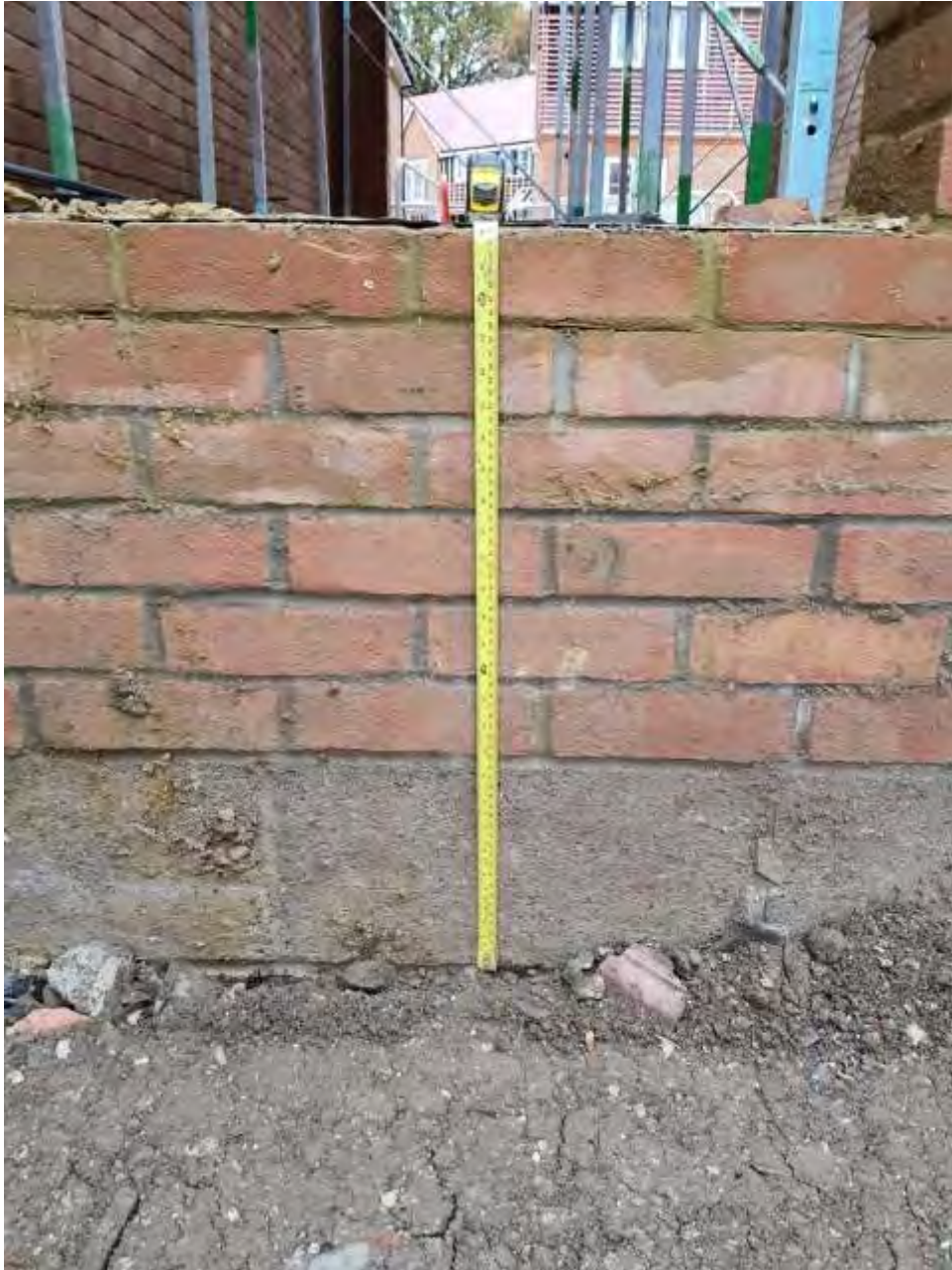
Plate 16 – Depth to crushed concrete layer
