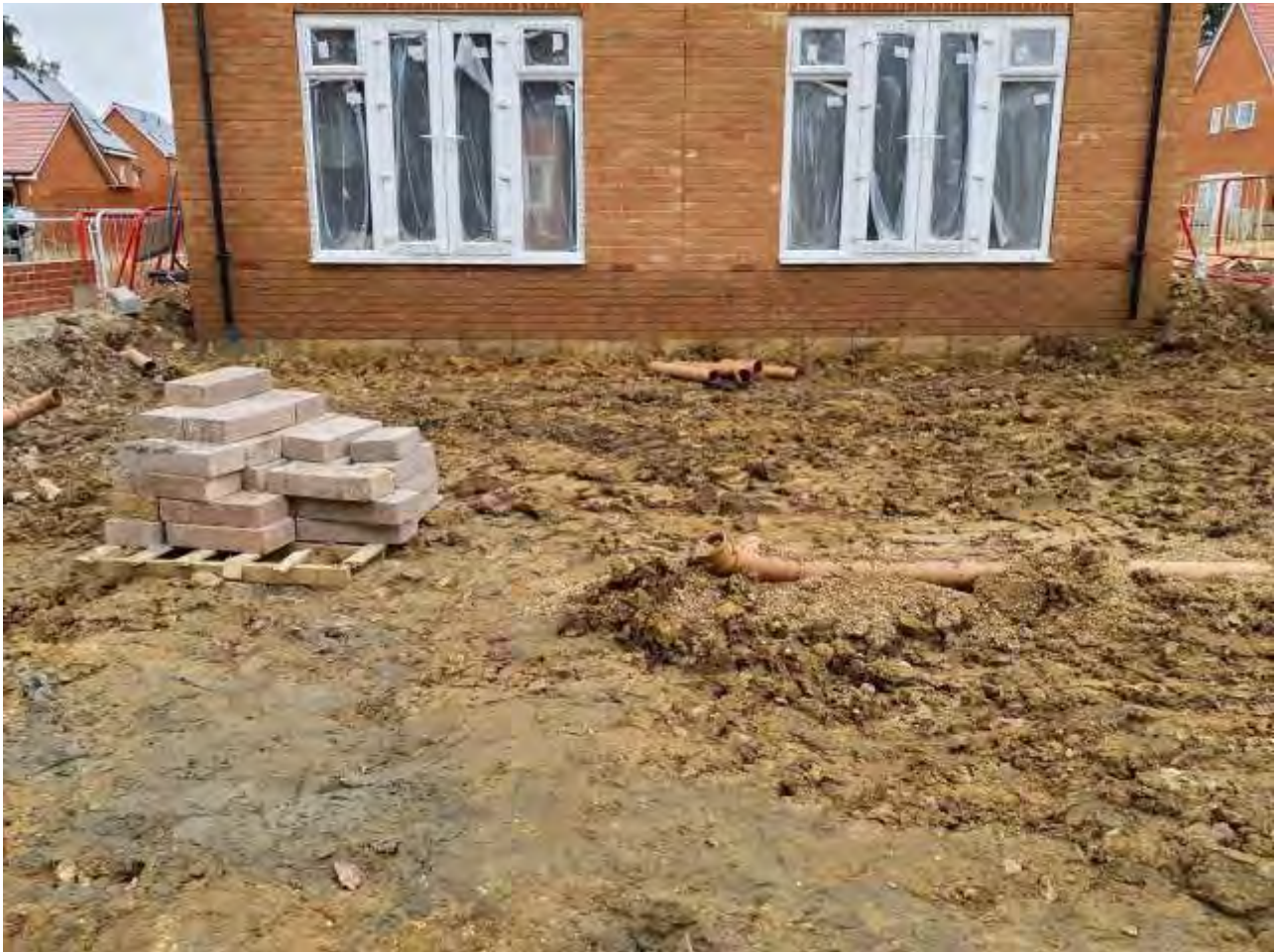
Plate 9 – View of reduced dig in Plots 121-122
