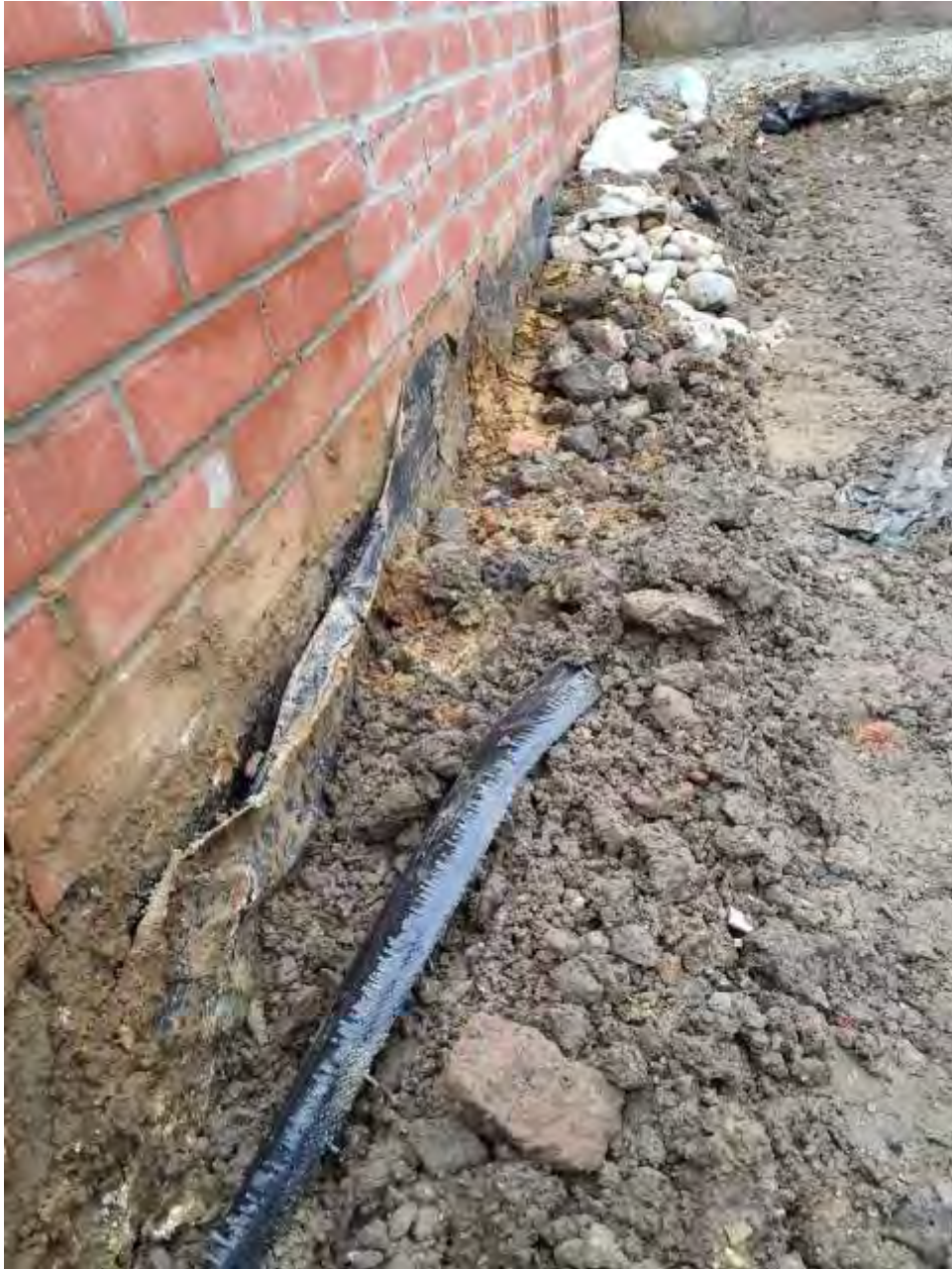
Plate 22 – View of membrane edge assumed to be installed beneath crushed concrete
