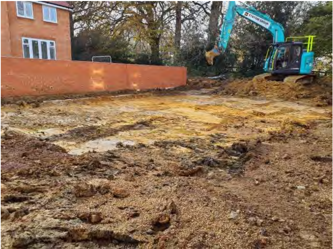
Plate 27 – View of reduced dig in progress in Plots 104-105
