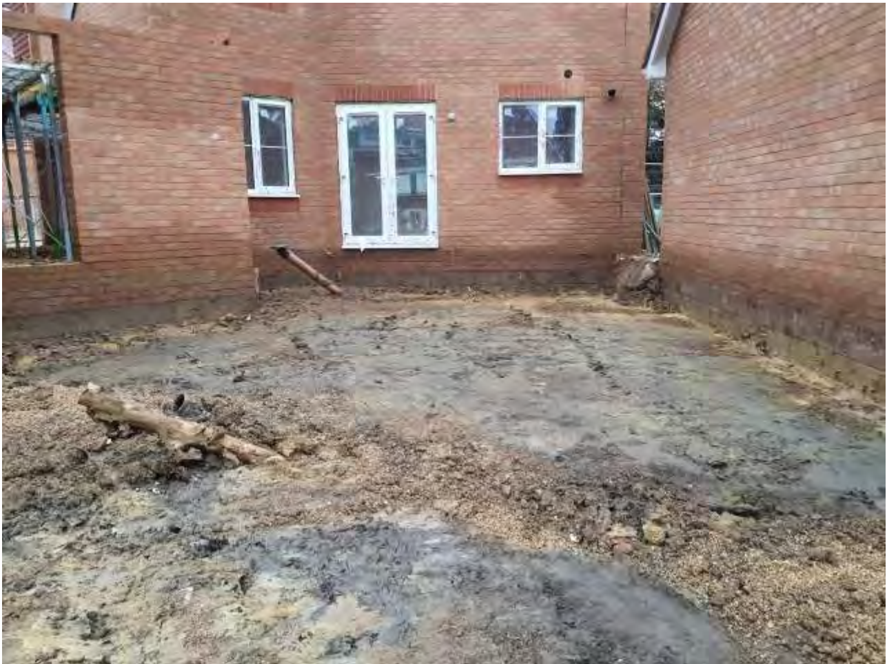
Plate 2 – View of reduced dig in Plot 102
