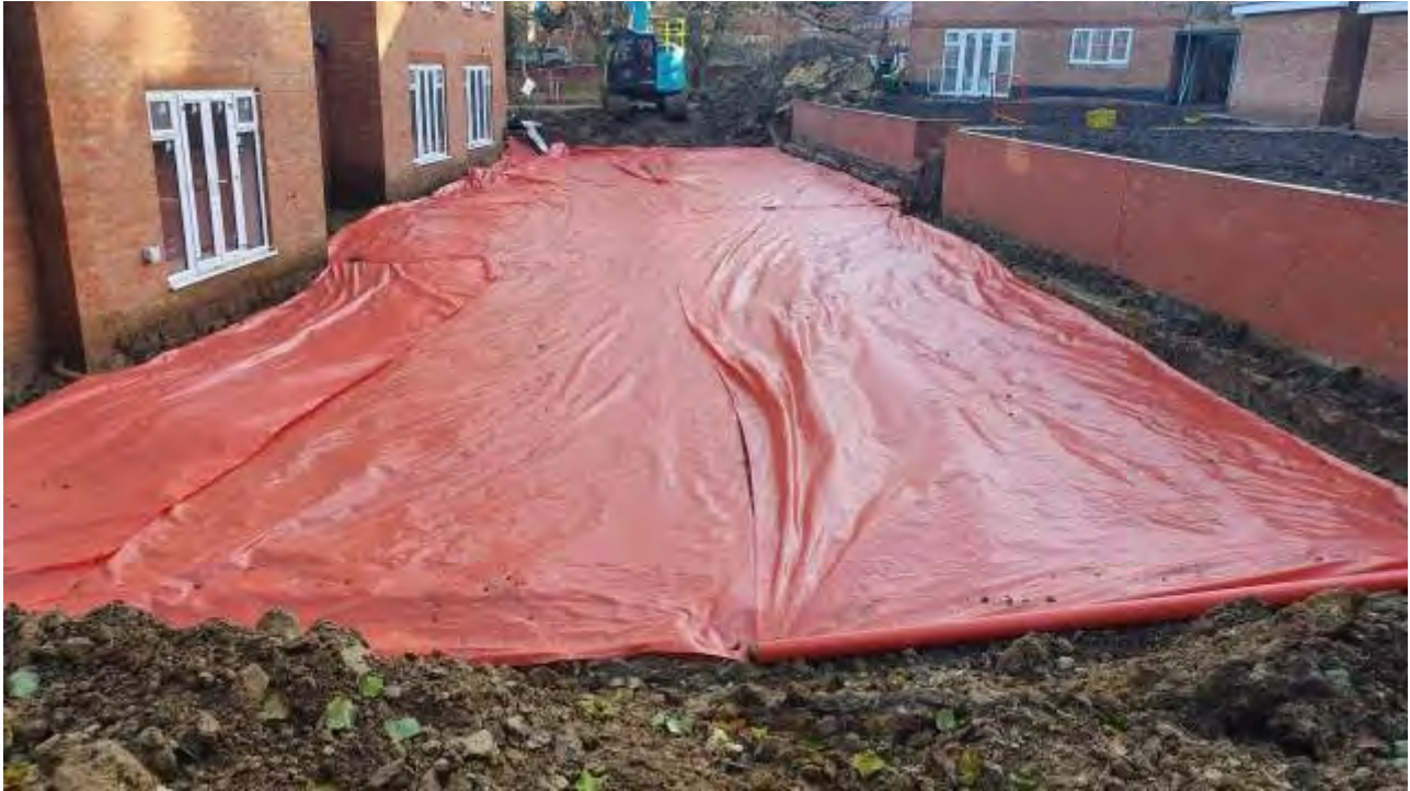
Plate 35 –View of the high visibility membrane installed above crushed concrete layer in Plots 104-107
