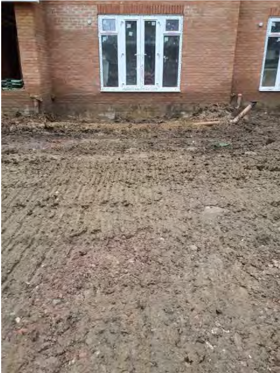
Plate 7 – View of reduced dig in Plot 101
