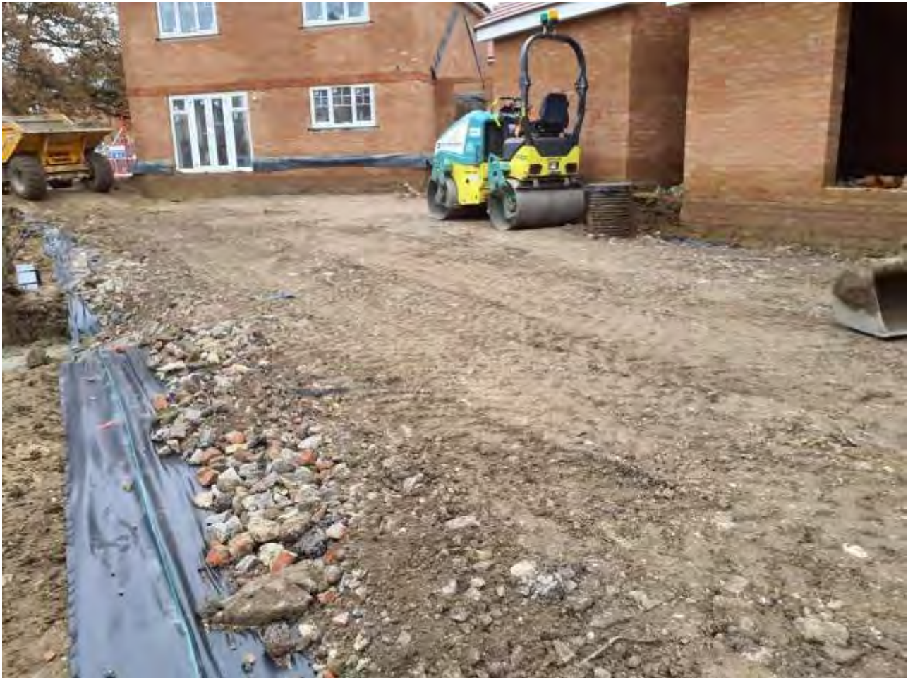
Plate 15 – View of crushed concrete installed across Plots 100-103
