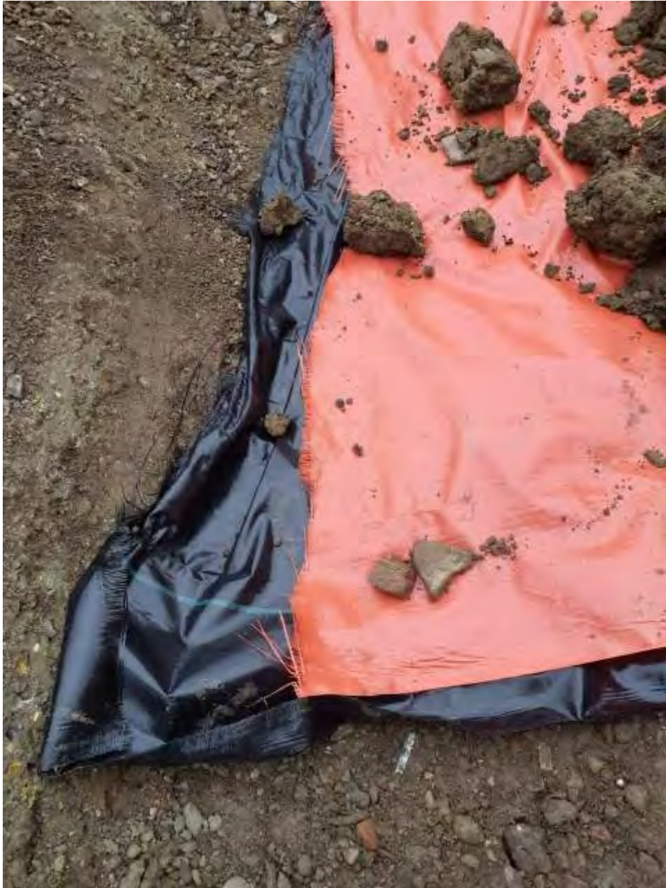
Plate 26 – View of black geotextile with high visibility geotextile installed above
