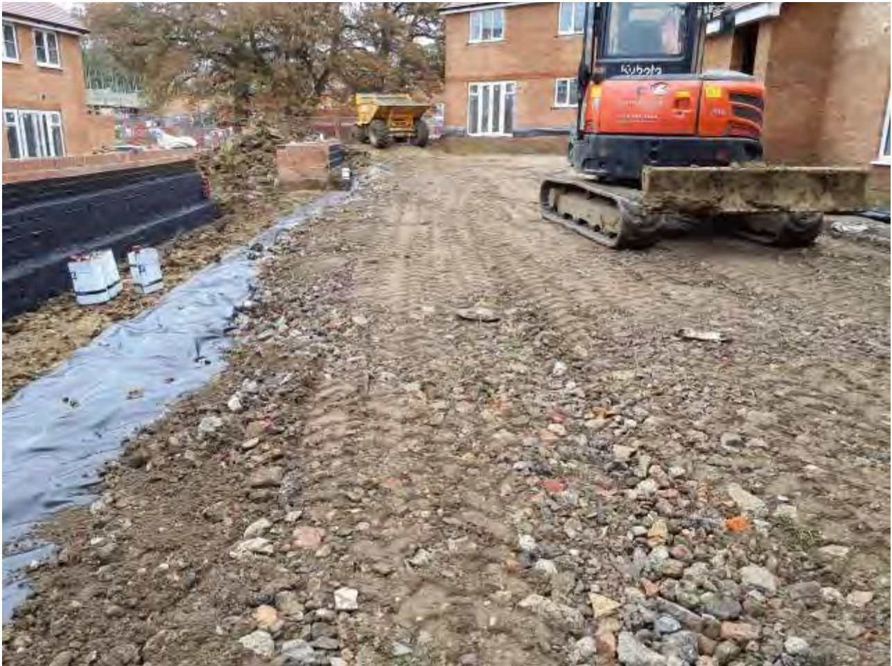
Plate 10 – View of crushed concrete layer in Plots 100-103
