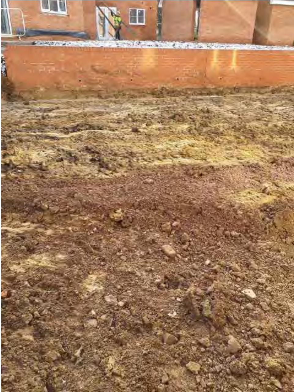
Plate 29 – View of the reduced dig in progress in Plot 107
