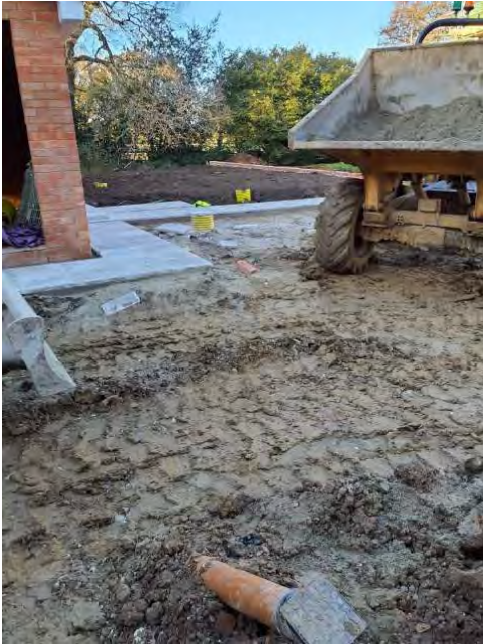
Plate 21 – View of subsoil installed in Plot 102
