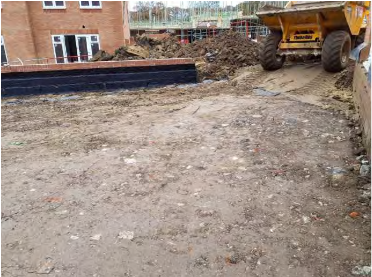
Plate 12 – View of crushed concrete layer installed in Plot 103
