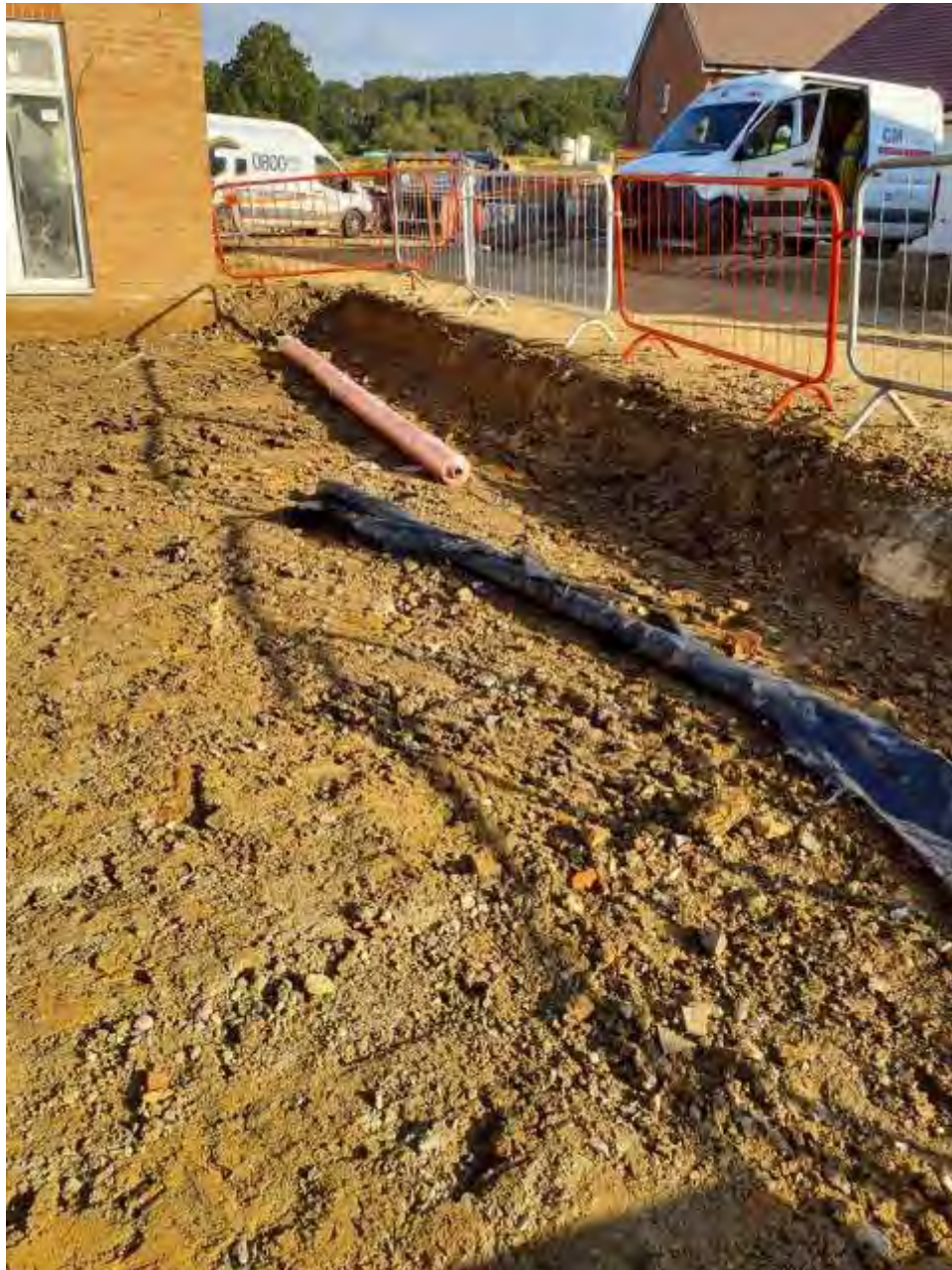
Plate 4 – View across the edge of reduced dig in Plot 119 with membrane rolls
