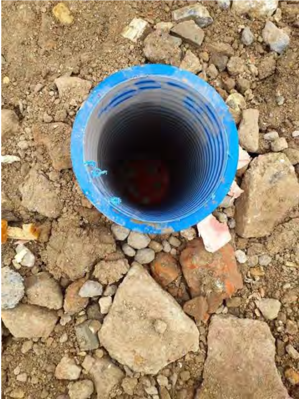
Plate 18 – View down inspection pipe installed in soft landscaping area showing membrane beneath crushed concrete
