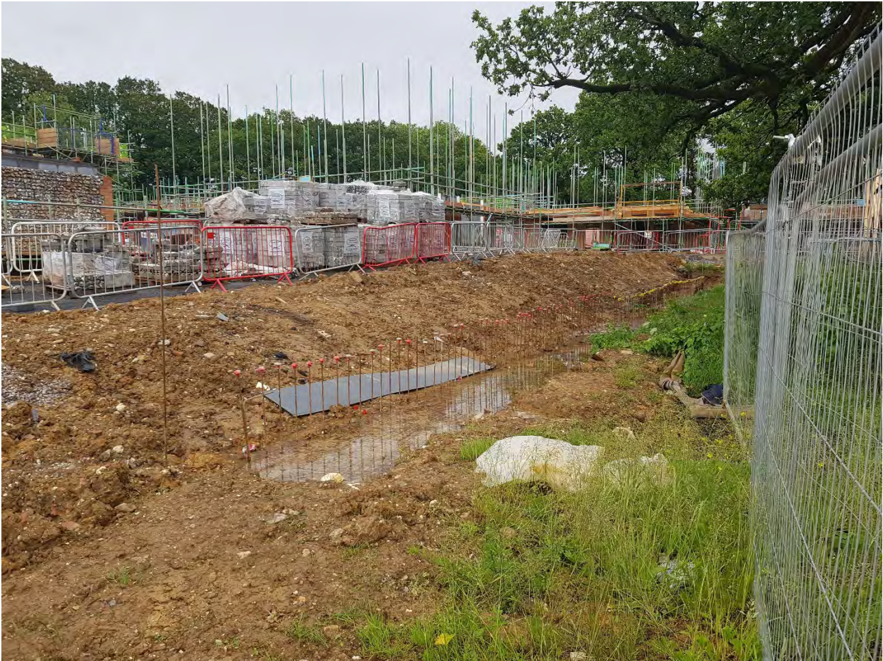
Plate 1 – View south towards Plots 121-122 during construction
