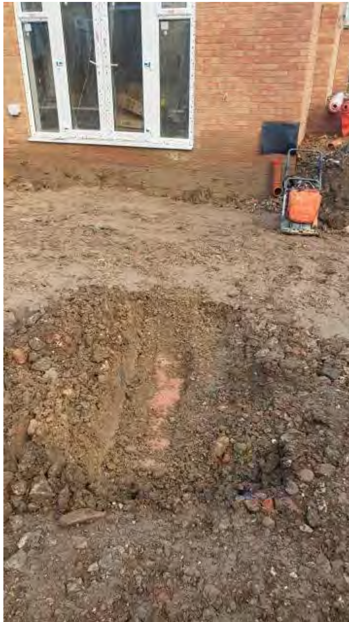
Plate 31 – View of the high visibility membrane installed beneath the crushed concrete layer in Plots 104-107
