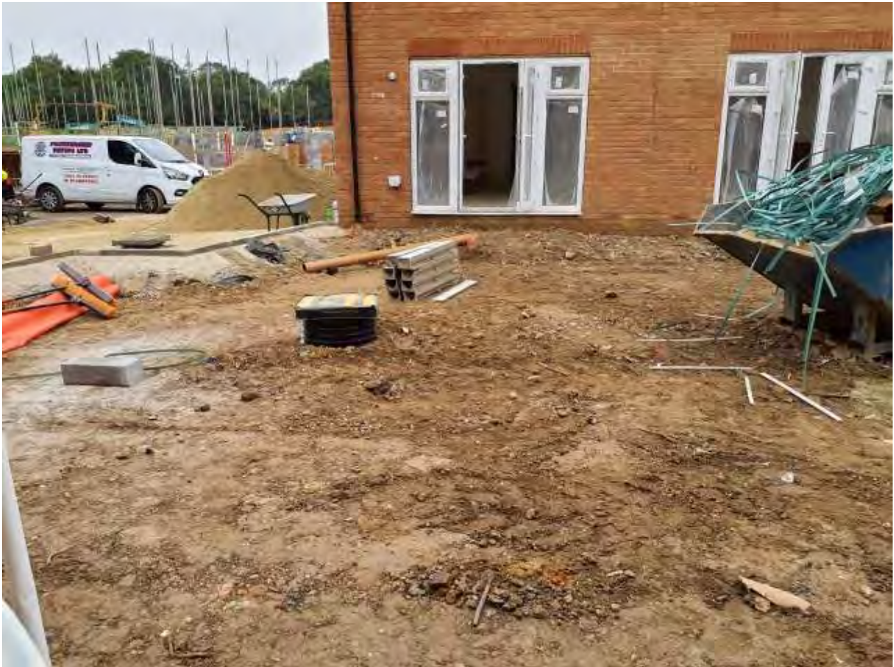
Plate 15 – View of crushed concrete installed in Plot 120
