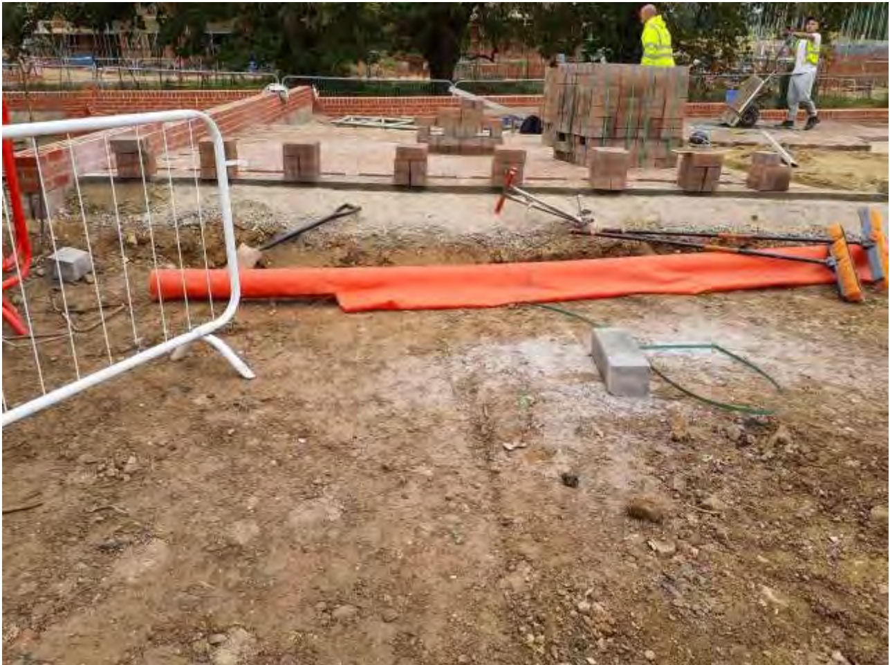
Plate 16 – View of crushed concrete with high visibility membrane for installation
