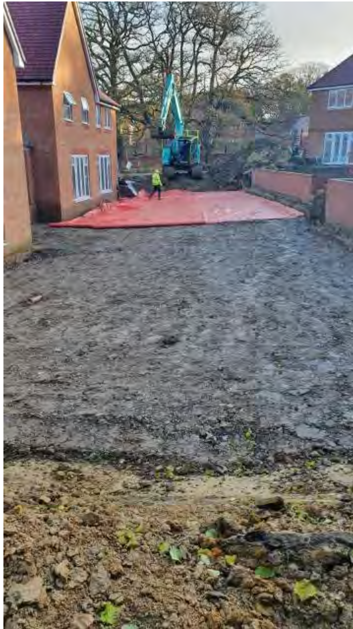
Plate 33 – View of the high visibility membrane being installed above crushed concrete layer in Plots 104-107
