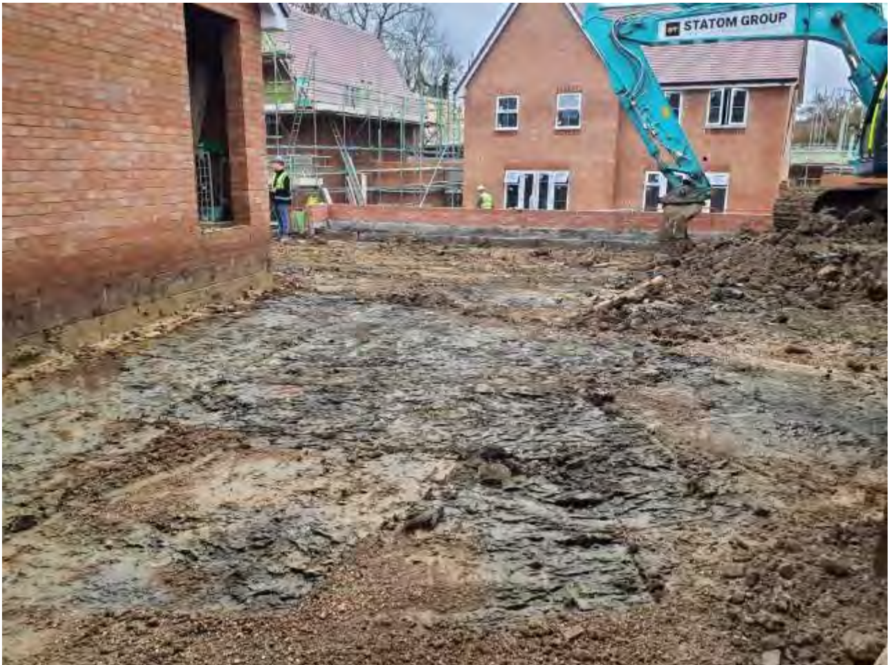
Plate 8 – View of reduced dig in Plot 102
