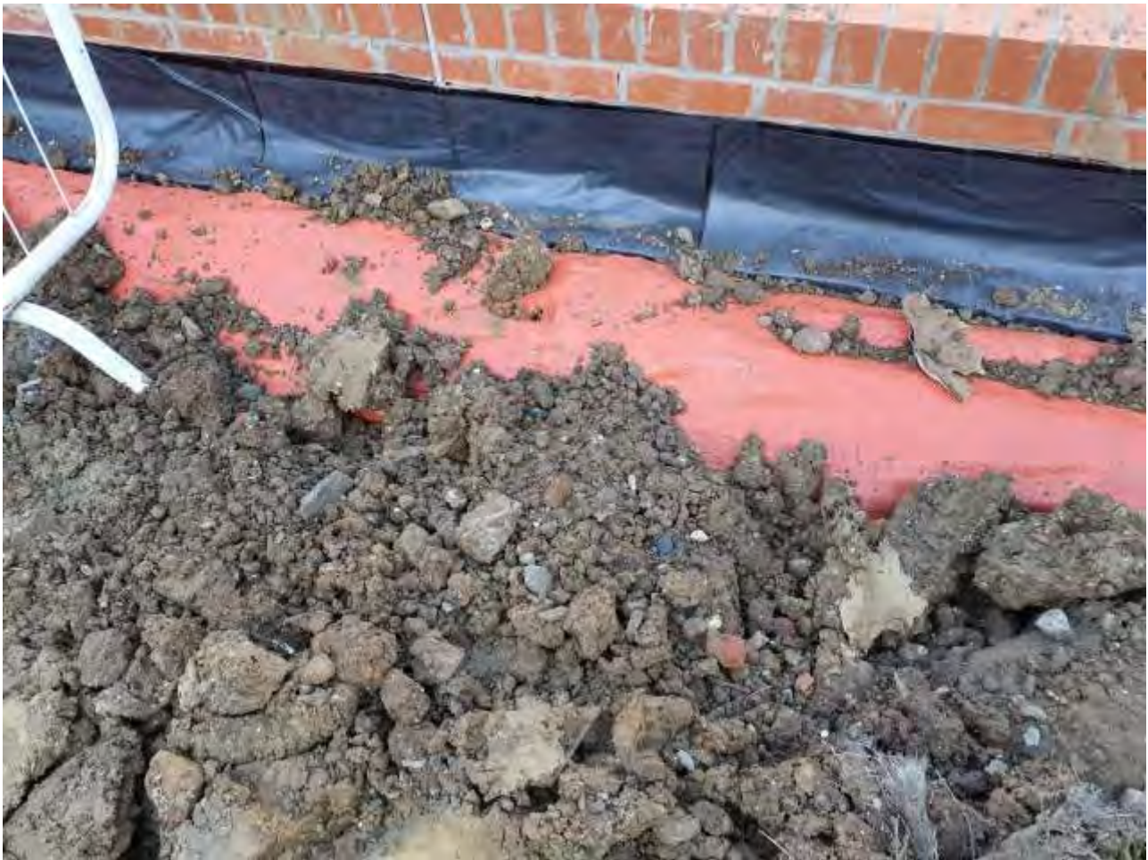
Plate 19 – View of high visible membrane installed beneath subsoil in Plot 102
