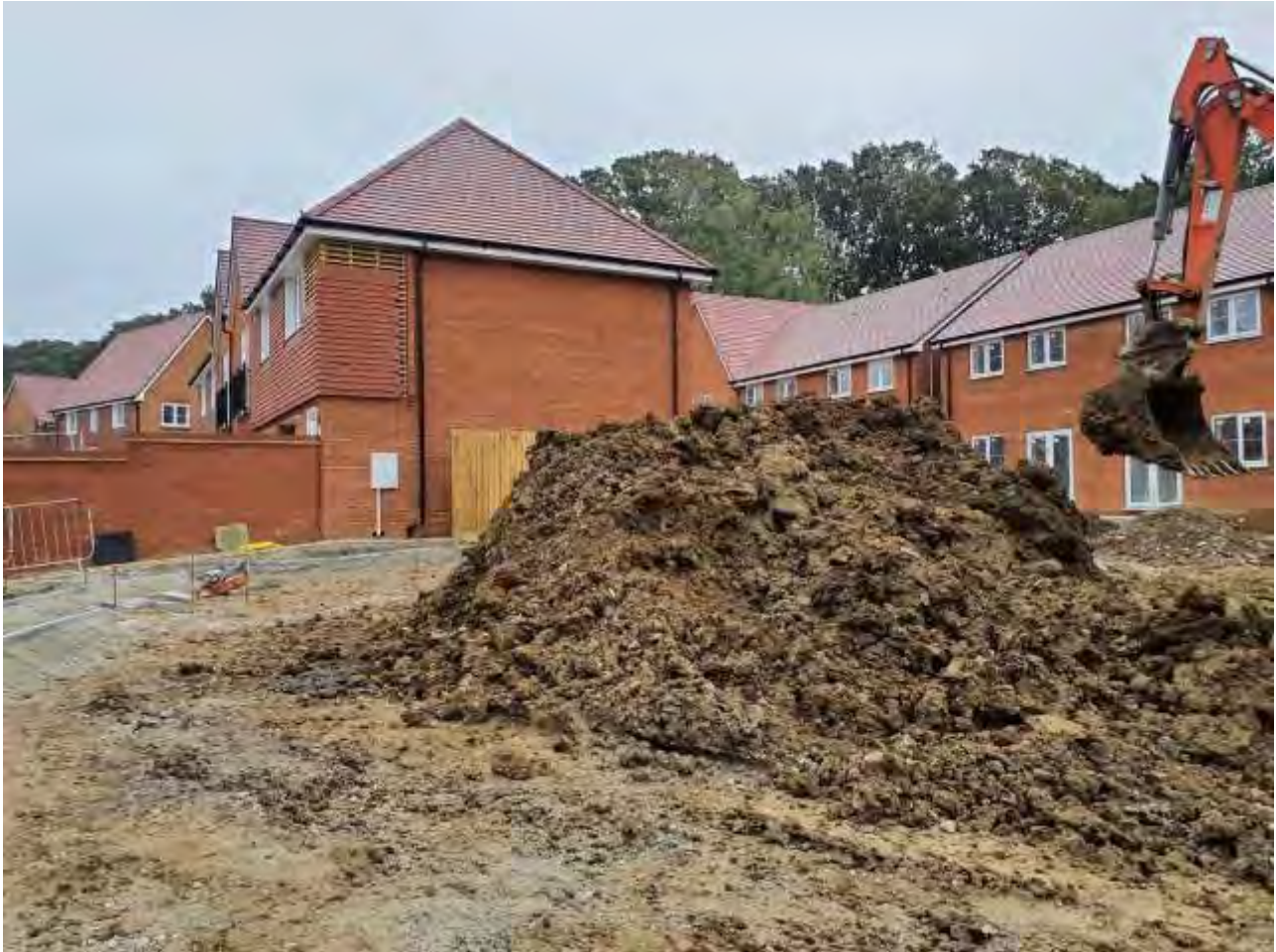
Plate 28 – View of the stockpile of site-won subsoil to be reused in rear garden areas
