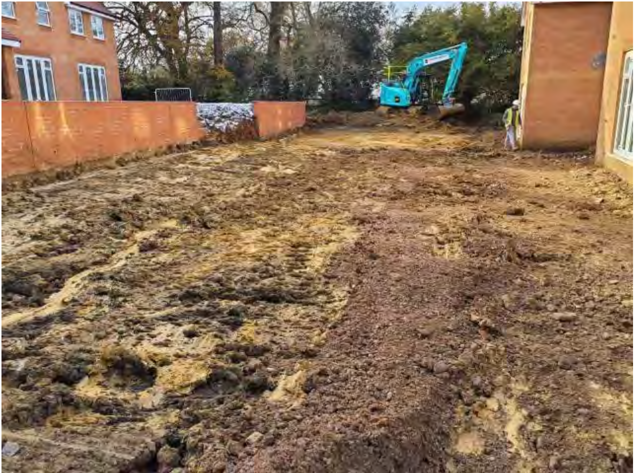
Plate 30 – View of the reduced dig in progress across Plots 104-107
