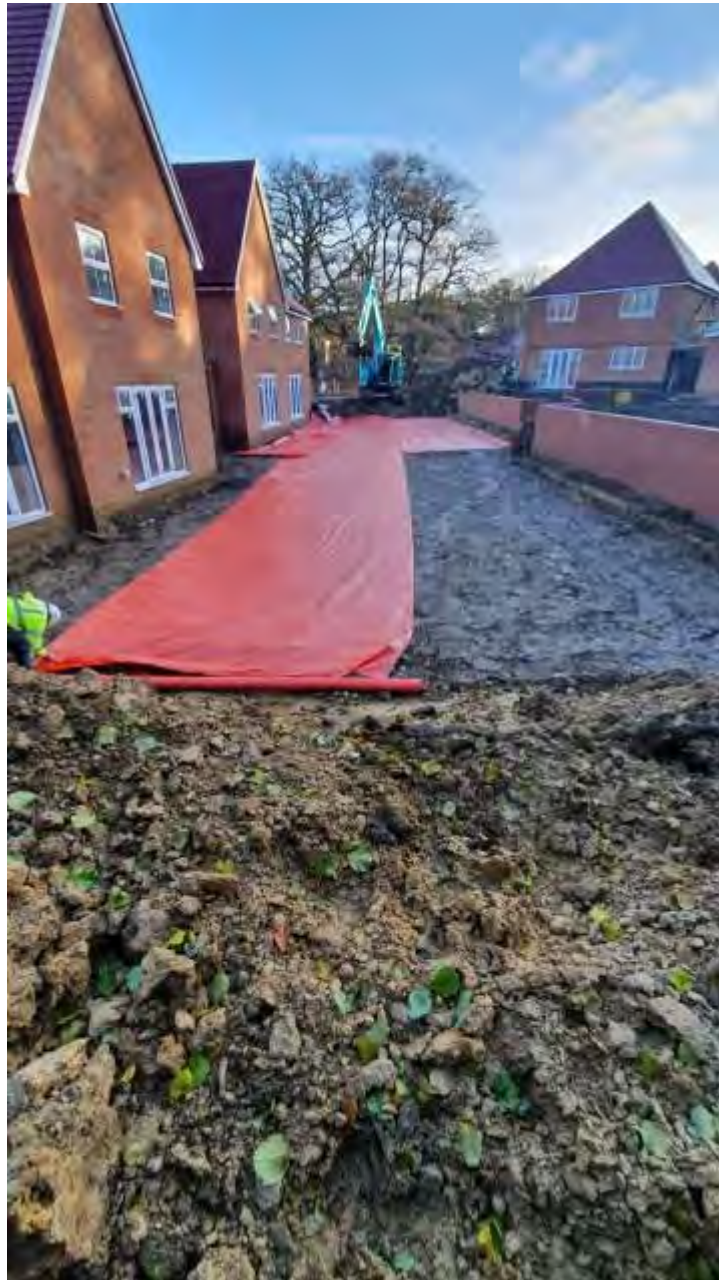
Plate 34 – View of the high visibility membrane being installed above crushed concrete layer in Plots 104-107
