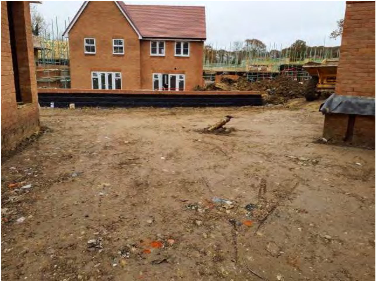
Plate 11 – View of crushed concrete in Plots 102-103
