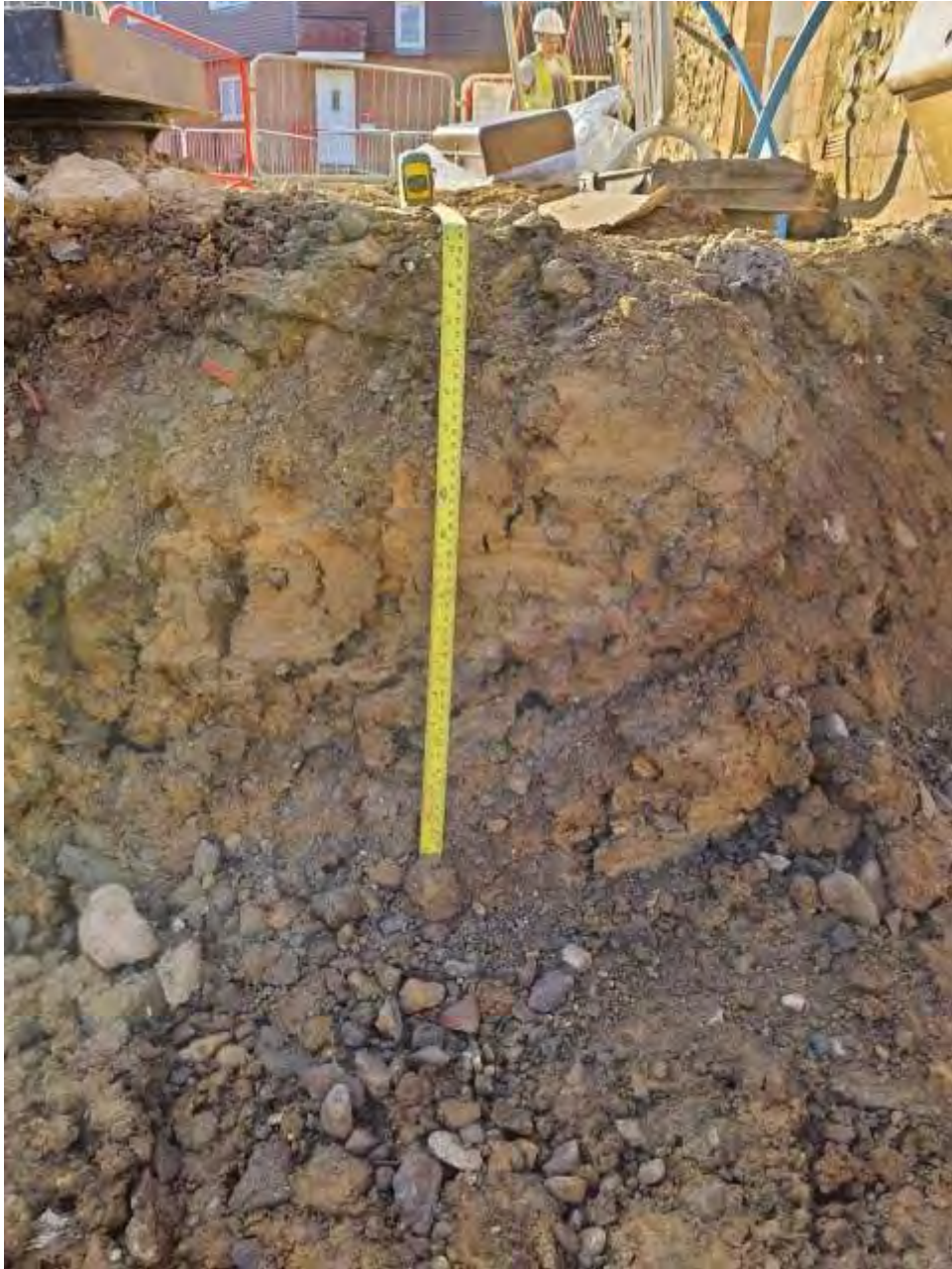
Plate 6 – Depth of reduced dig across Plots 119-120
