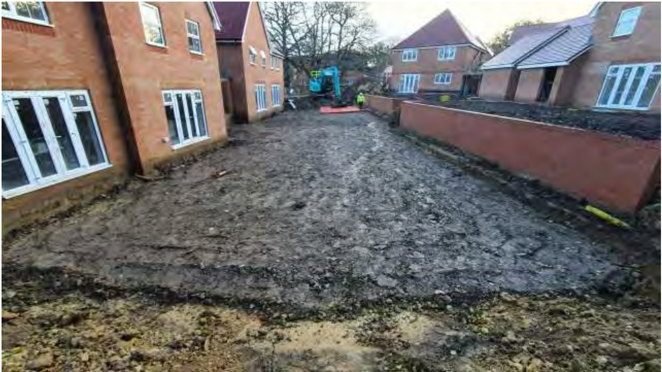
Plate 32 – View of the crushed concrete layer across Plots 104-107
