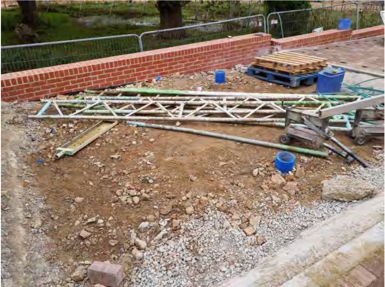
Plate 17 – View of soft landscaped area to west of Plot 120 with crushed concrete layer
