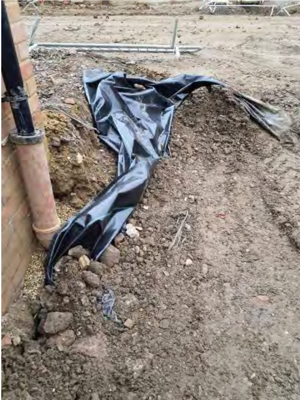
Plate 23 – View of membrane edge beneath crushed concrete
