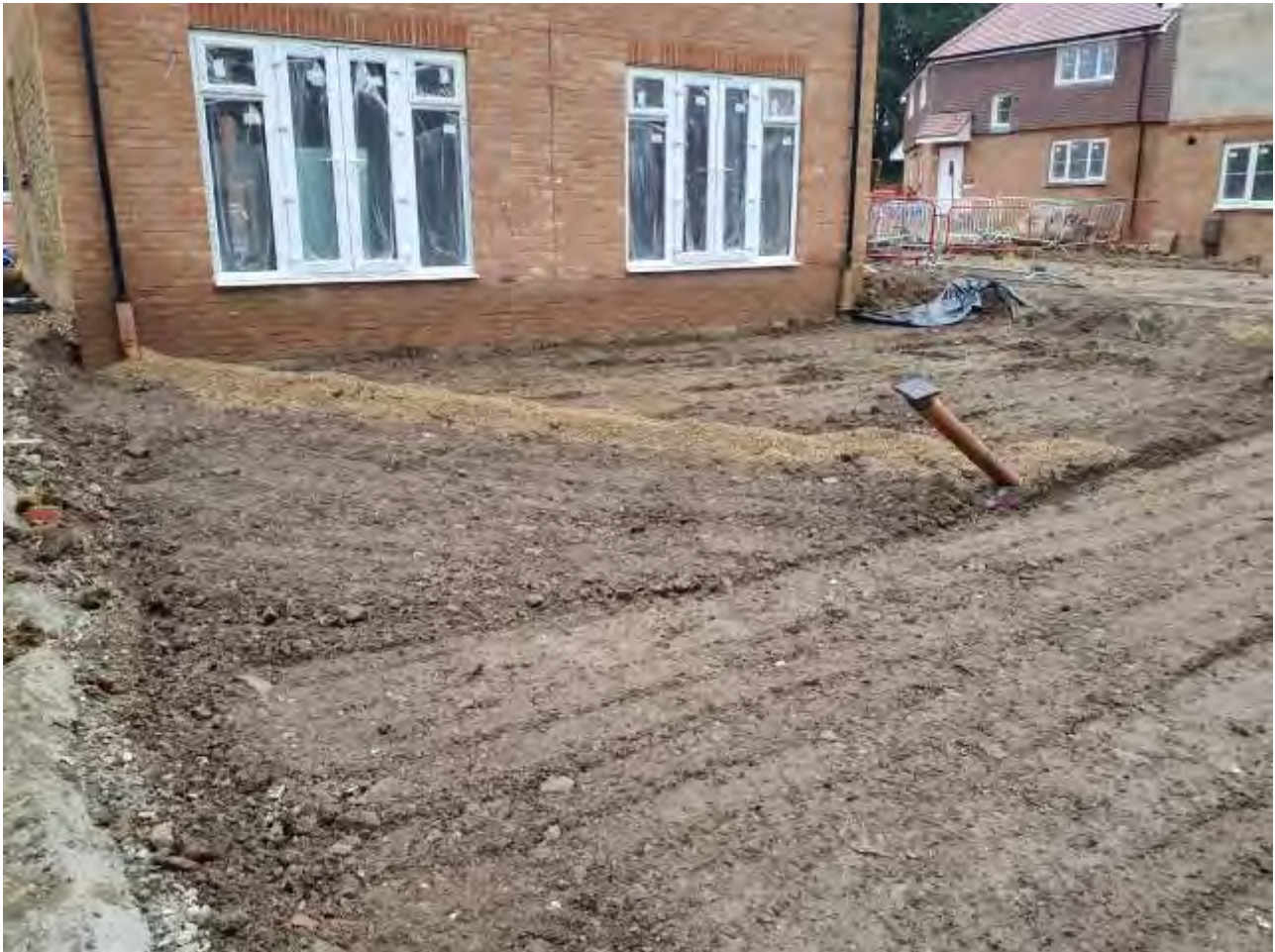
Plate 20 – View of crushed concrete layer installed in Plots 121-122
