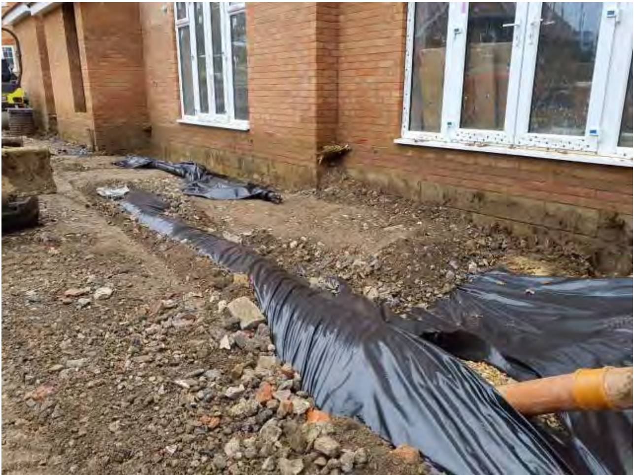
Plate 9 – View of crushed concrete in Plots 100-101
