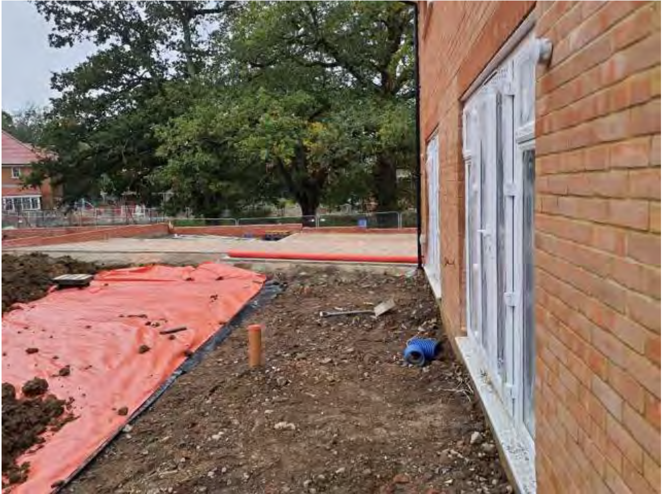
Plate 27 – View across Plots 119-120 of the ongoing installation of membranes and subsoil
