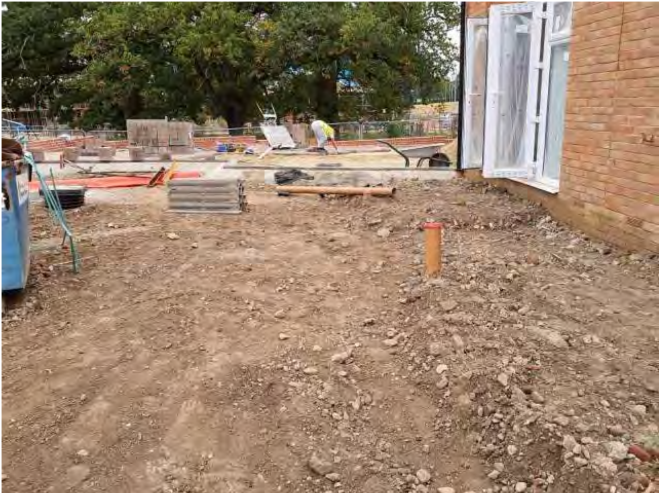
Plate 13 – View across crushed concrete layer installed in Plots 119-120
