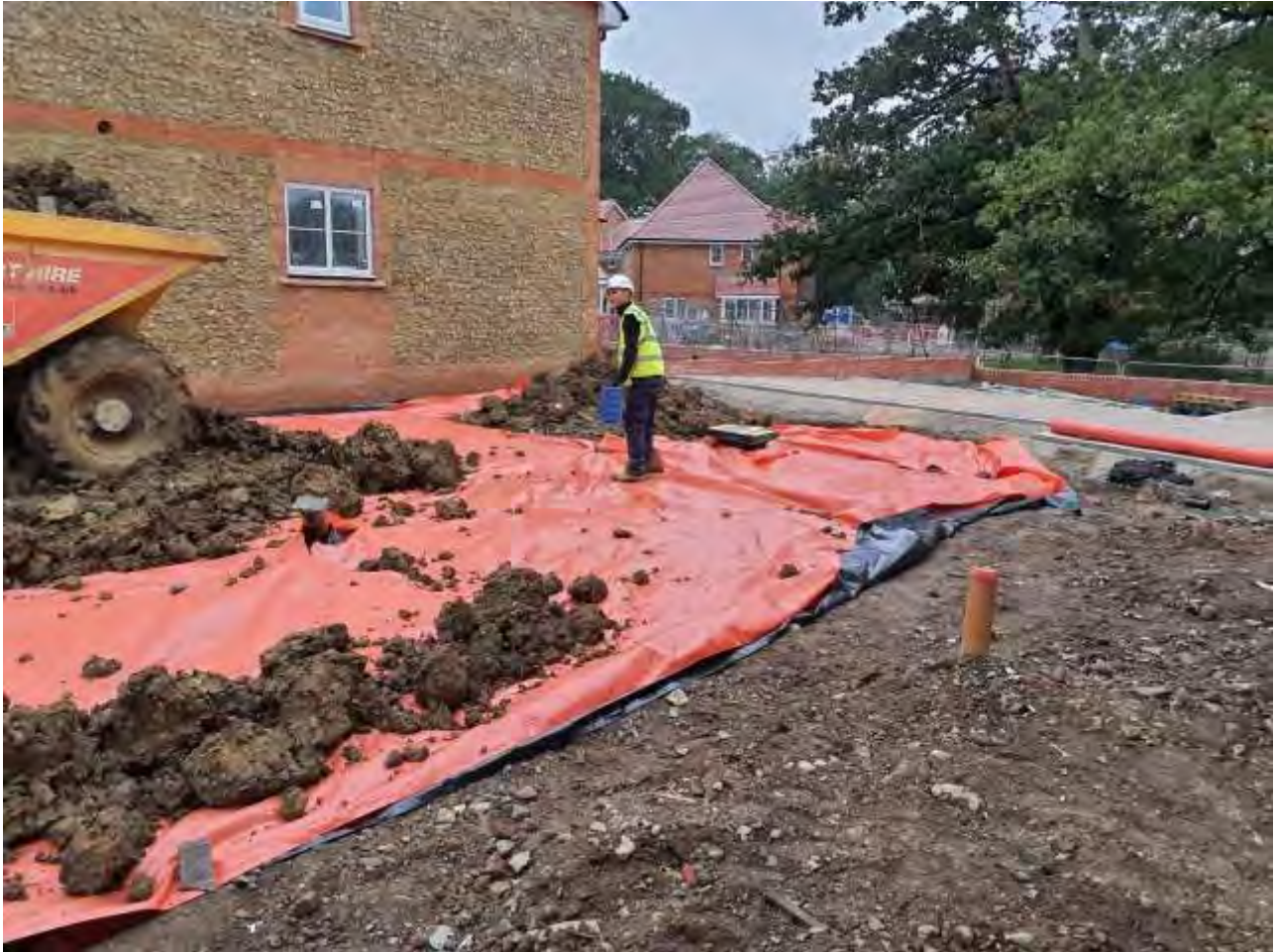
Plate 24 – View of the installation of membranes and subsoil in Plots 119-120 above crushed concrete
