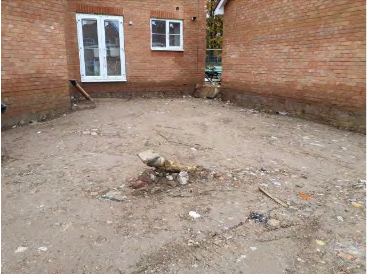
Plate 18 – View of crushed concrete installed in Plot 102
