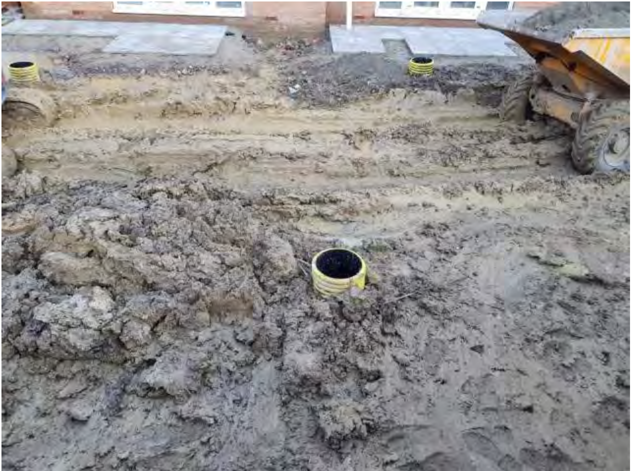
Plate 37 –View of the subsoil installation in Plots 106-107
