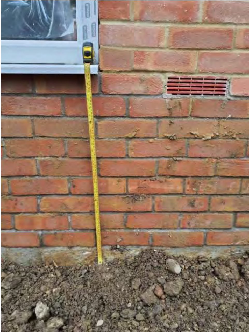
Plate 21 – Depth to crushed concrete layer in Plots 121-122
