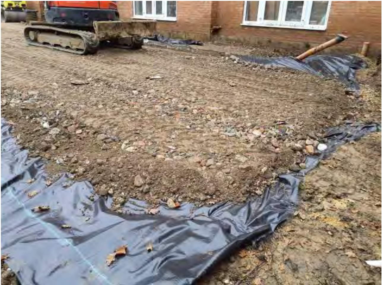
Plate 13 – View of crushed concrete installed in Plot 100
