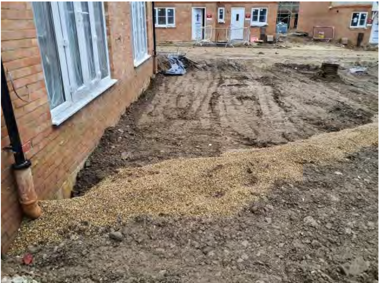
Plate 19 – View of crushed concrete layer installed in Plots 121-122 along with gravel drainage run
