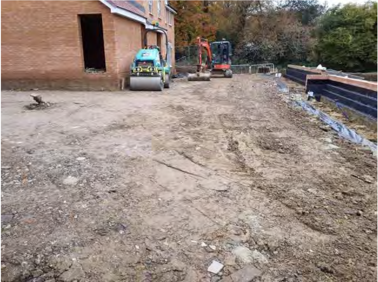
Plate 14 – View of crushed concrete installed across Plot 100-103
