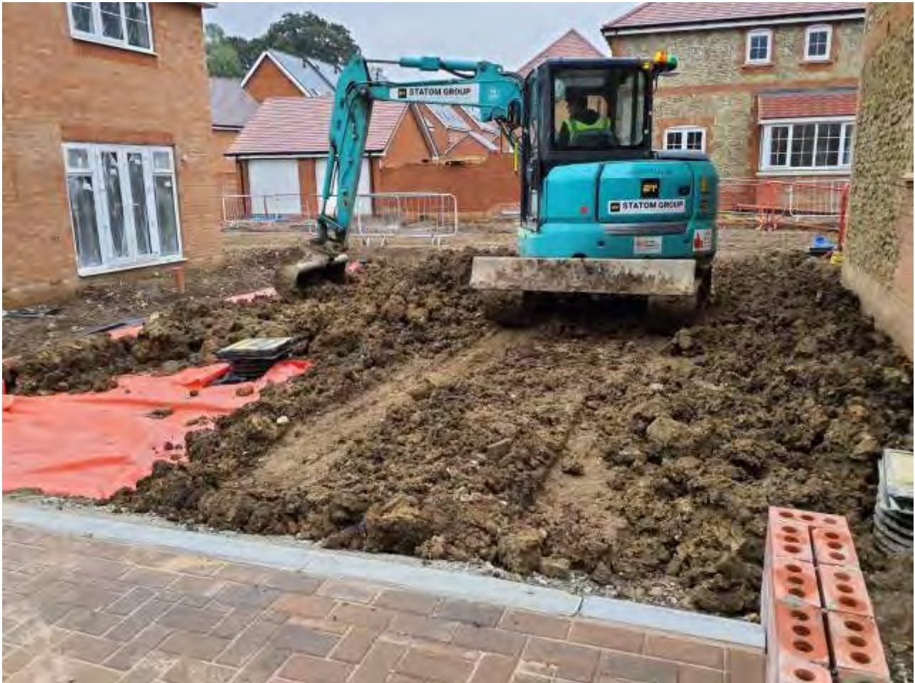
Plate 25 – View of the installation of membranes and subsoil in Plots 119-120
