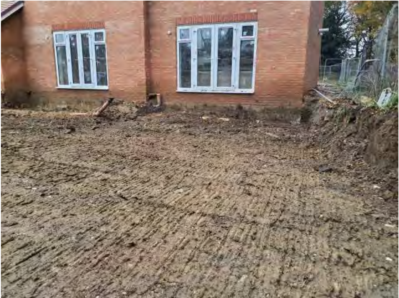
Plate 1 – View of reduced dig in Plot 100
