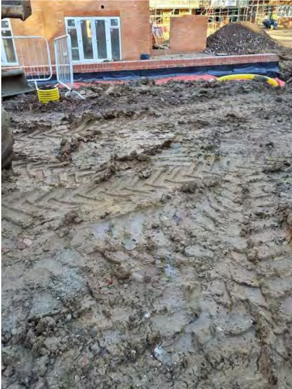
Plate 20 – View of subsoil installed in Plot 102
