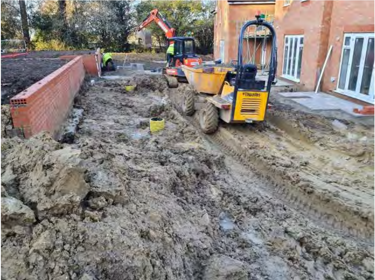
Plate 38 –View of the installation of subsoil in progress in Plots 106-107
