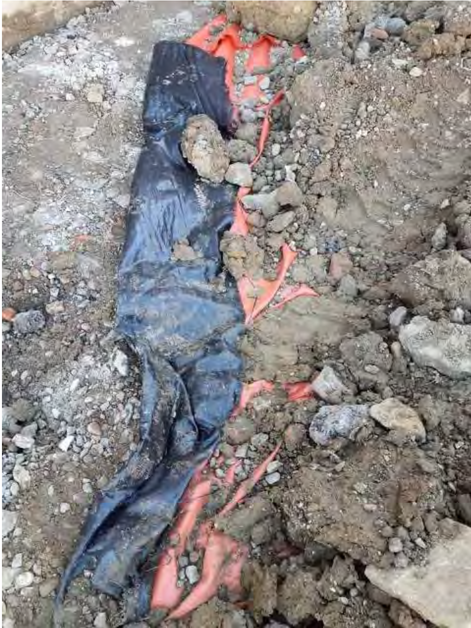
Plate 22 – View of membrane edge beneath subsoil in Plot 103
