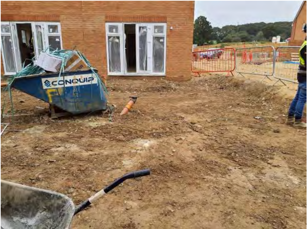
Plate 14 – View of crushed concrete installed in Plot 119
