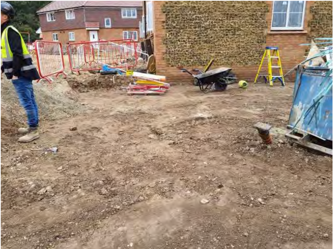
Plate 12 – View of crushed concrete layer installed in Plot 119
