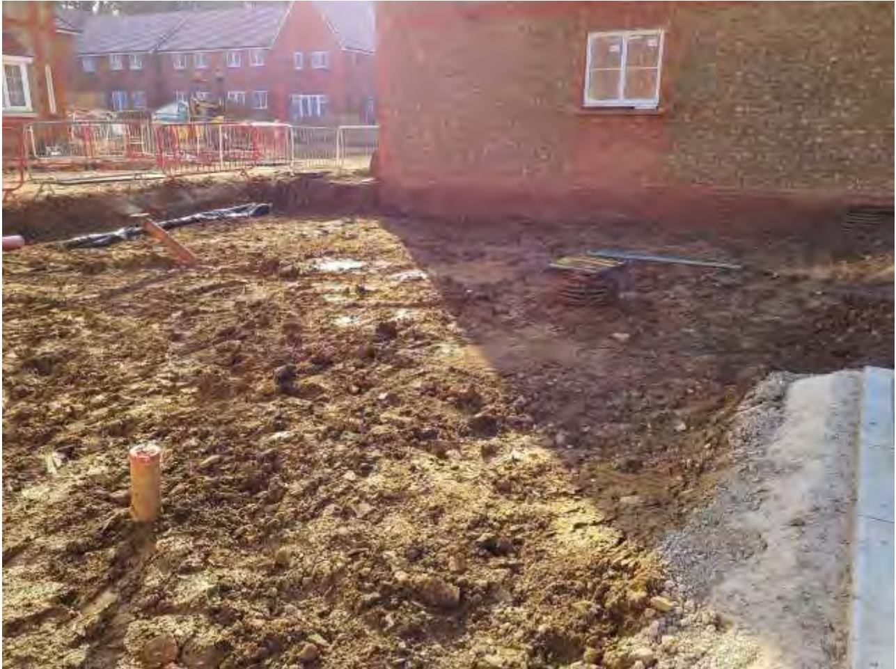
Plate 7 – View south across reduced dig in rear gardens of Plots 119-120
