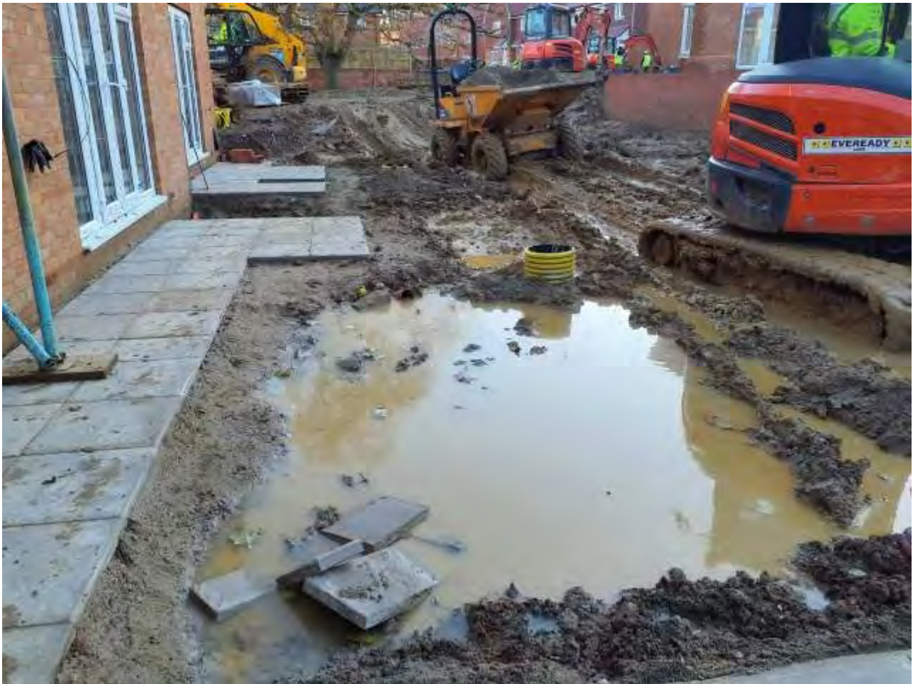
Plate 36 –View of the subsoil being installed within Plots 106-107
