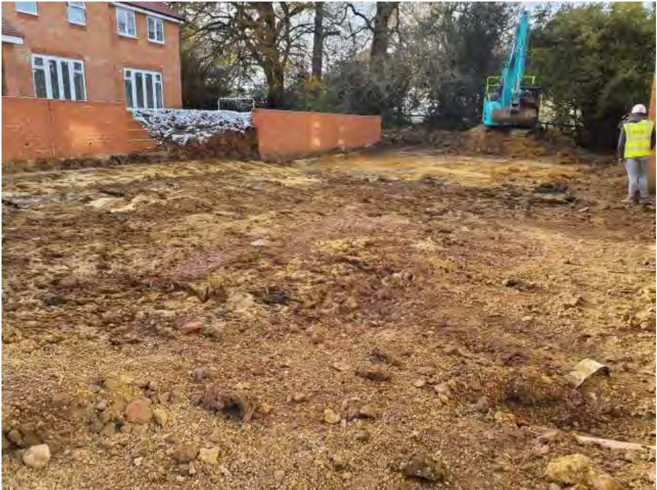
Plate 28 – View of reduced dig in progress in Plot 106
