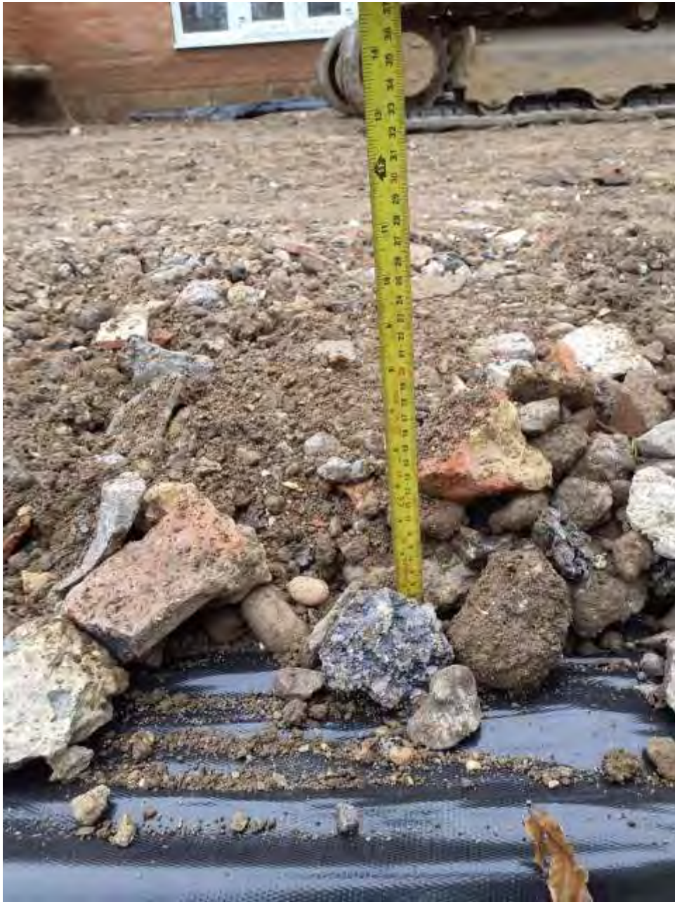
Plate 17 – Depth of crushed concrete
