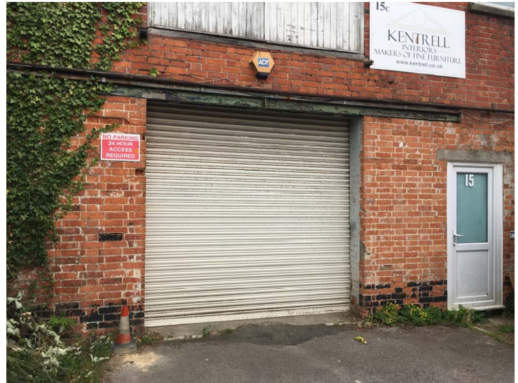
Main access to unit
