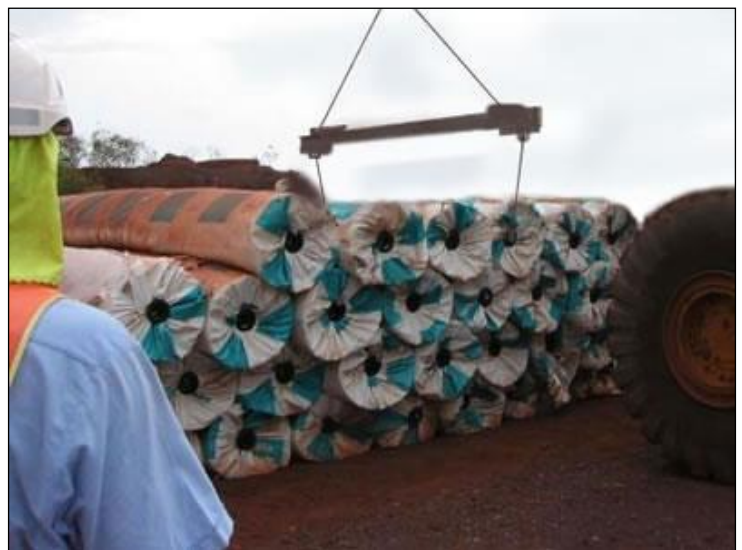
Figure 4 Tensar Basetex rolls stacked on site (Max 4 rolls high)
