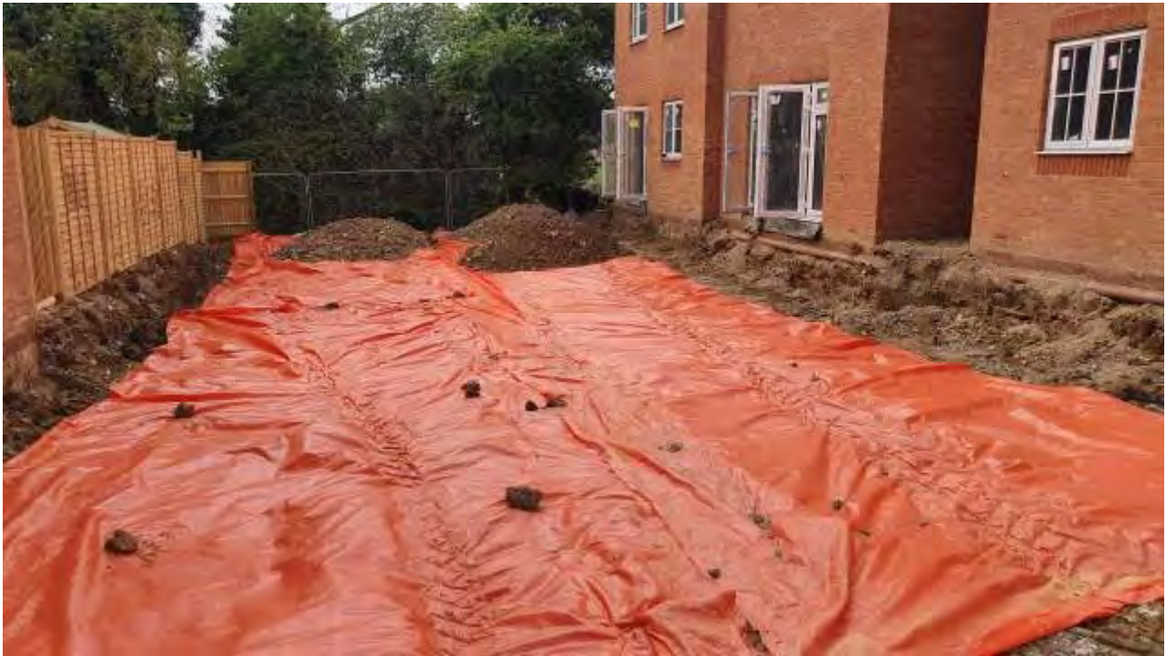
Plate 4 – View of membrane installed above crushed concrete layer across Plots 141-144
