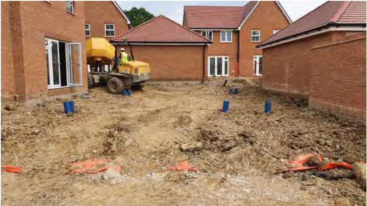
Plate 2 – View of subsoil installed within Plot 129-130
