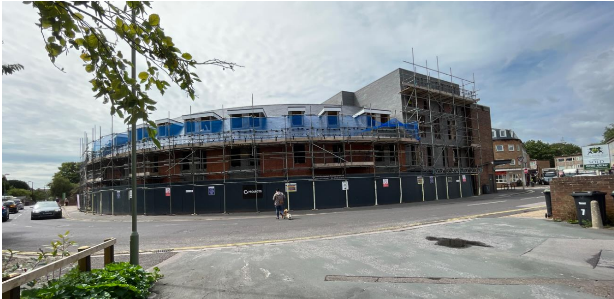
Figure 5 North Street Arcade Site – To east of Warner House – Currently being Redeveloped with 29 Flats – View from North-East
