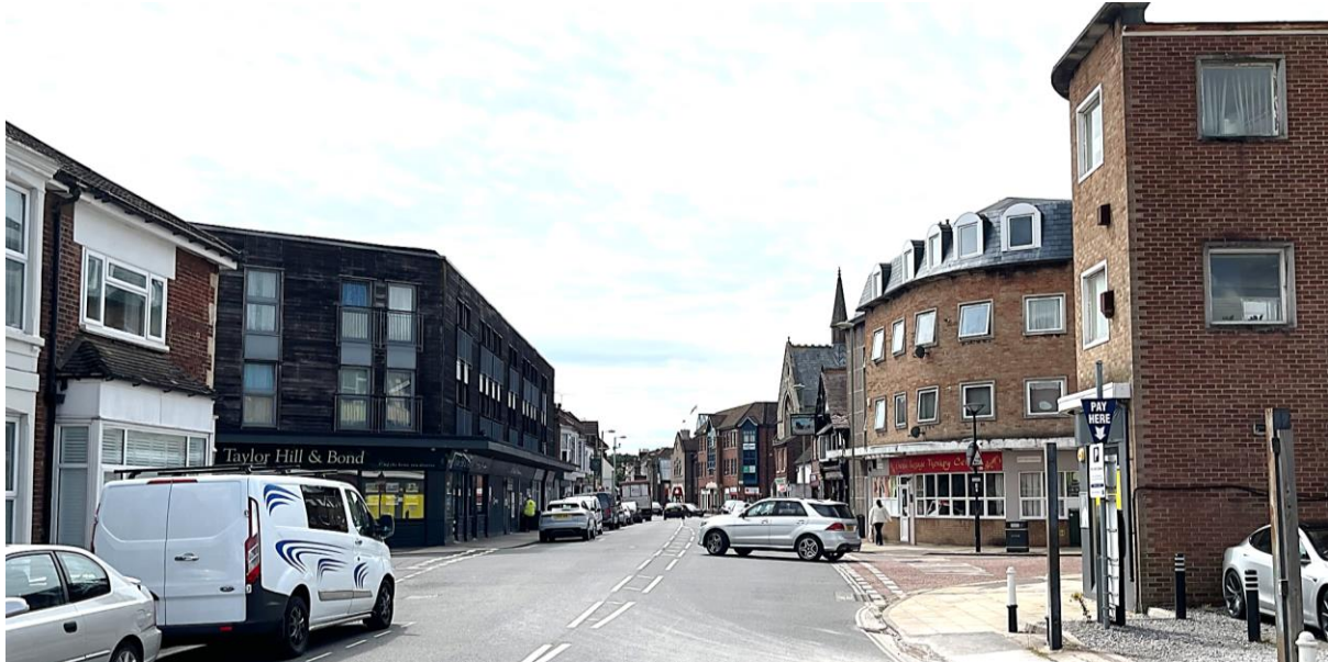
Figure 3 Warner House on Corner of North Street & Prince George Street – 4-Story Block of Flats on Opposite Corner with Market Parade
