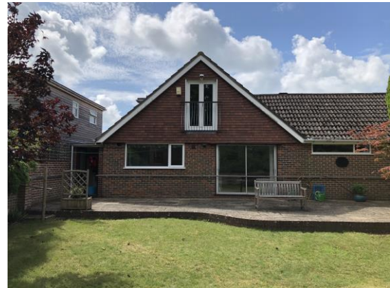
Figure 7: View of north elevation
