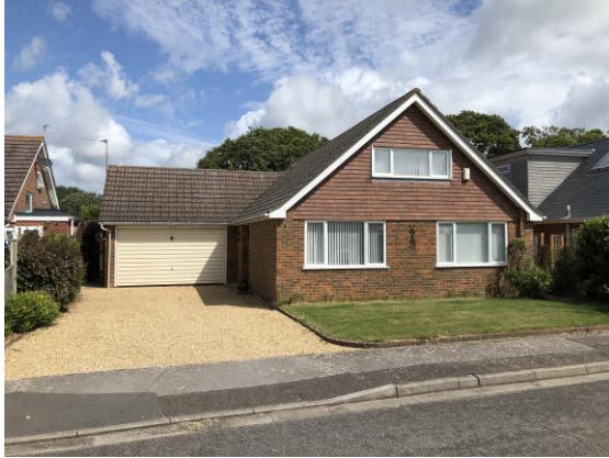
Figure 4: front view of the south elevation.
