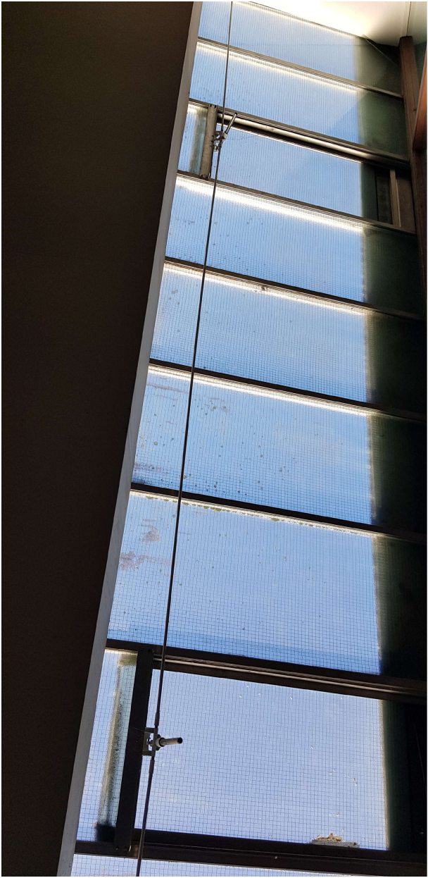
1 Interior photograph of existing patent glazing
