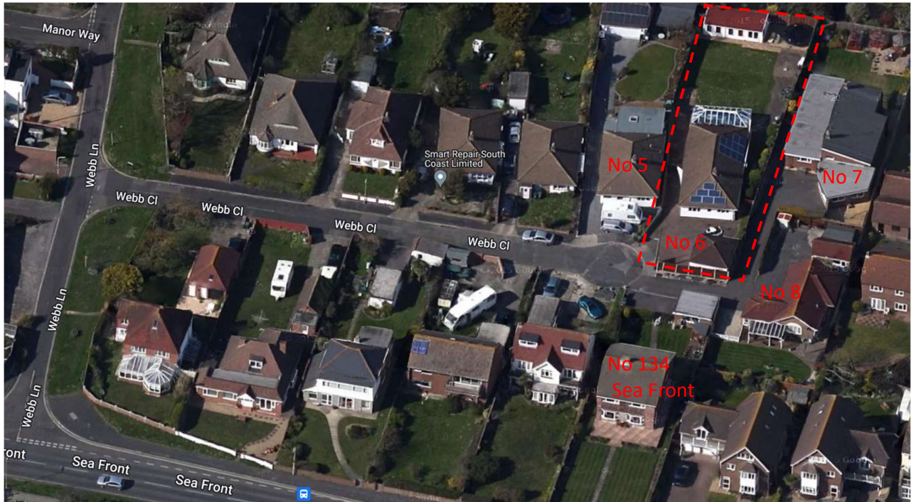
Aerial View of Webb Close with subject site at No. 6
