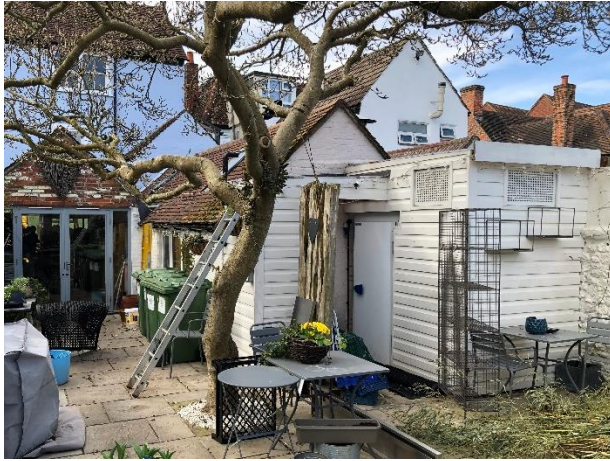
Figure 2: Old upvc storage spaces at the back of the building [to be demolished]
