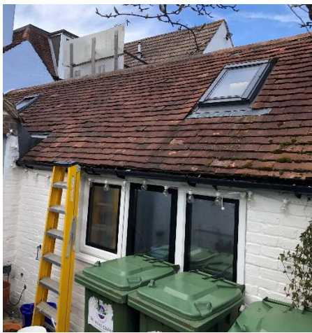
Figure 3: Existing clay roof element [to be extended]
