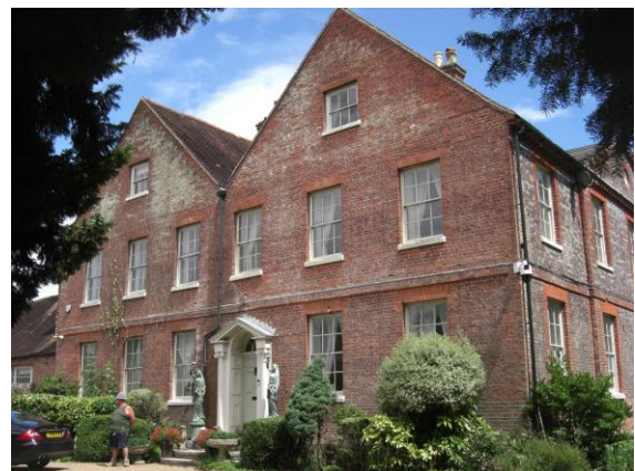
The Manor House west facade
