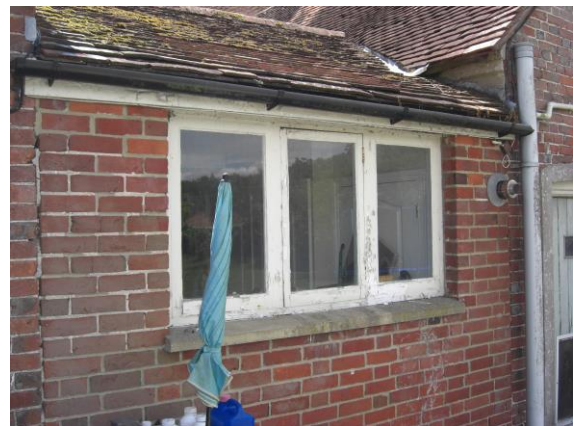
Casement on the north elevation
