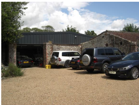
Approach to the service yard and outbuildings
