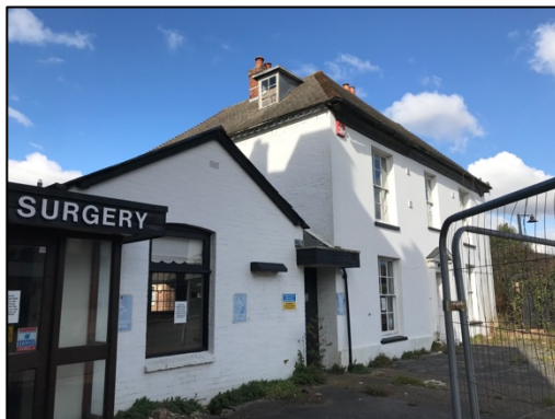
Figure 8 – eastern elevation, with the southern pitched and flat roof extensions
