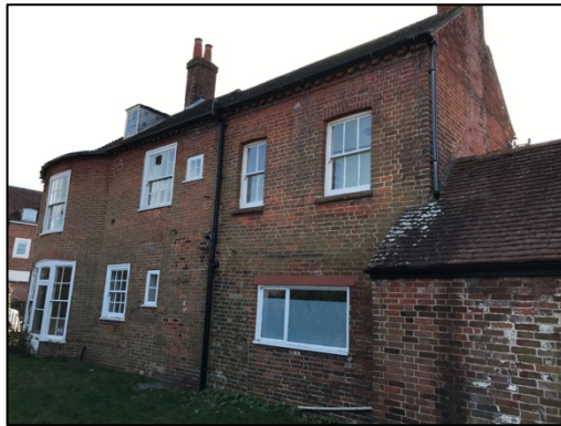
Figure 6 – northern elevation of the main building
