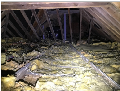
Figure 10 – main roof void
