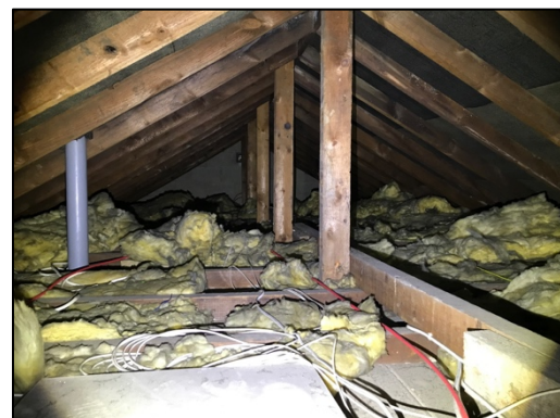
Figure 11 – southern roof void
