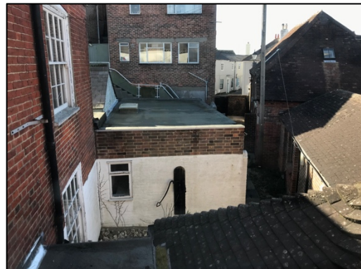
Figure 9 – westernmost flat roof extension
