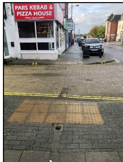
Photograph 4: Tactile Paving on Victoria Road
