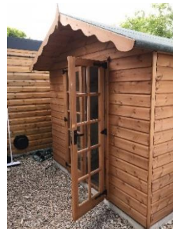
Figure 4: Timber office shed at the rear
