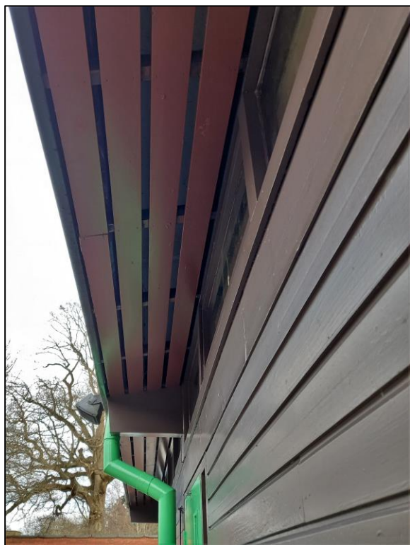
Photo 4 Cavity within the eaves, lined with smooth metal.
