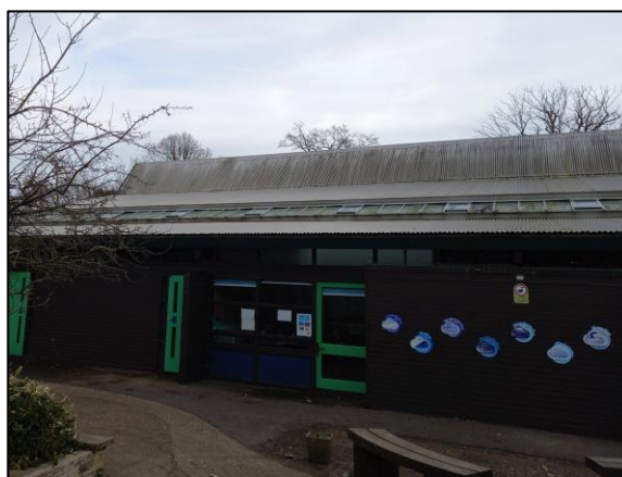
Photo 7 General view of the roof from the north.
