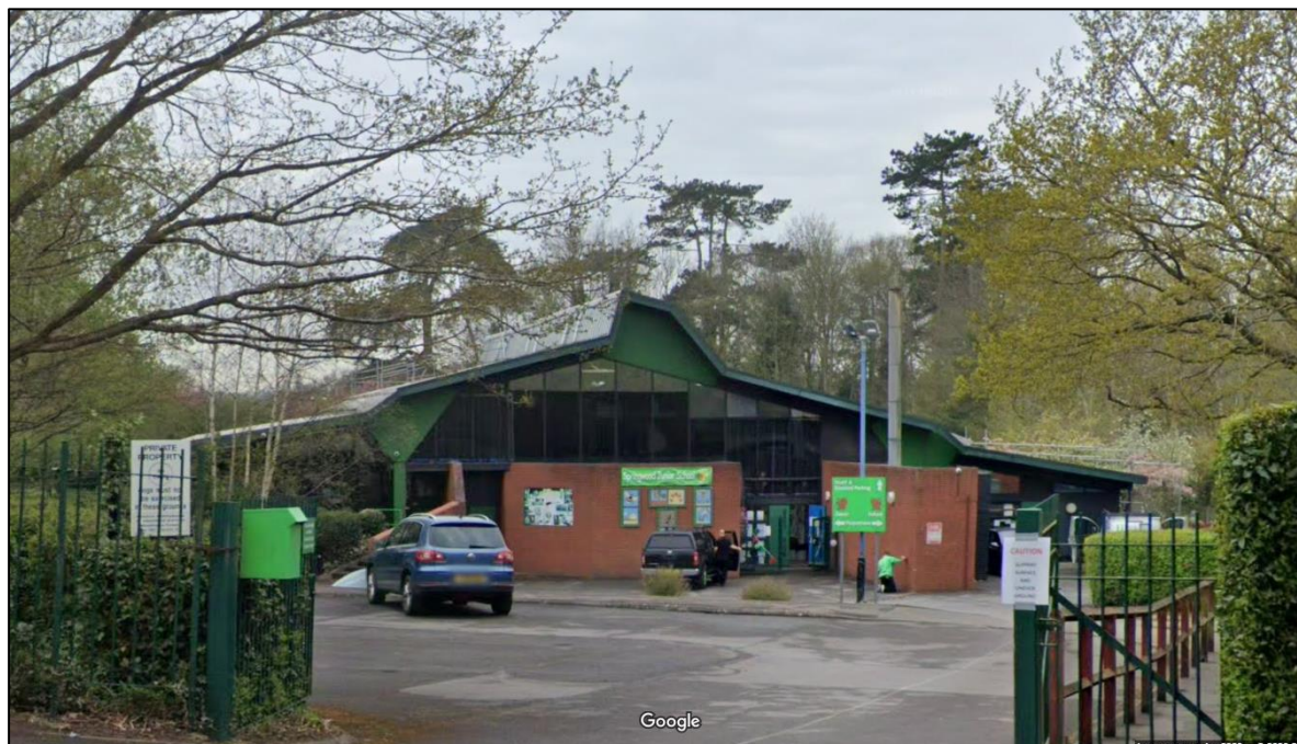
Photo 1 General view of the main school building from the east, showing expansive roof of unusual shape.
