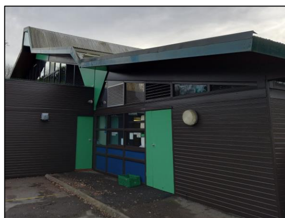
Photo 3 View from the north-east, showing tightly-fitting wall components and two large vents into the kitchen.
