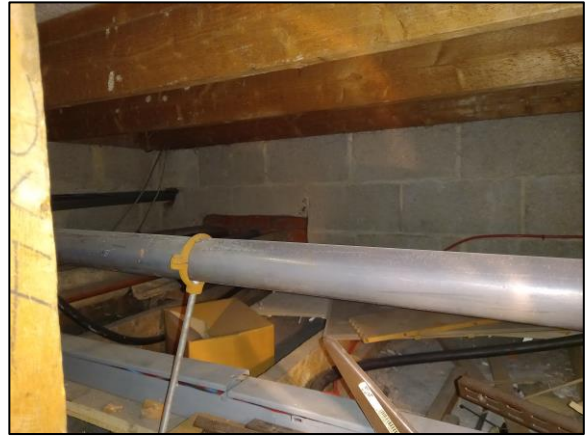
Photo 9 Inside the loft space above the caretaker's office.
