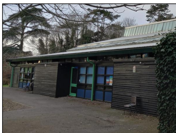
Photo 2 View from the south, showing typical wall construction, with a mix of boarding and glazing.
