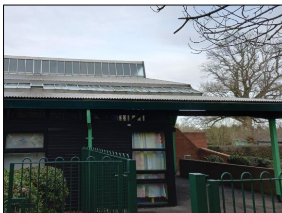
Photo 6 General view of the roof from the south.
