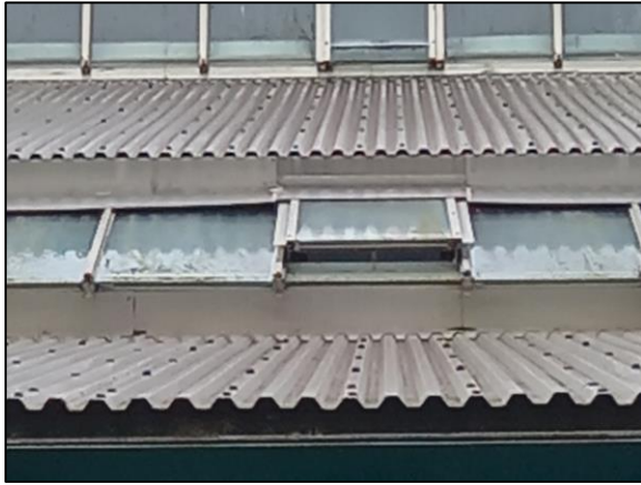
Photo 8 Detail of corrugated metal roof, glazing and flashing.
