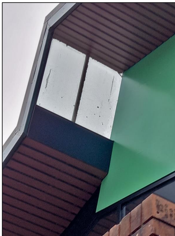
Photo 5 Large overhang at the ends of the building, same construction as the eaves.
