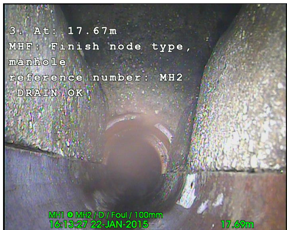
Photo: 150122_1613A-Survey.jpg 17.69m, Finish node type, manhole reference number: MH2 DRAIN OK
