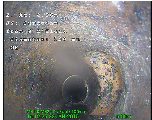
Photo: 150122_1612A-Survey.jpg 5m, Junction from 9 O'Clock diameter: 100 mm OK
