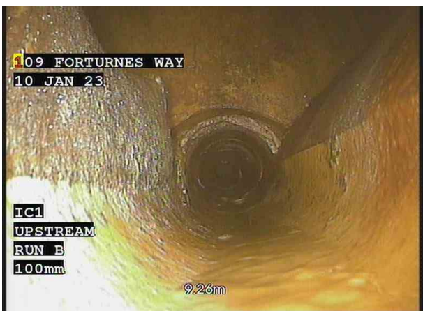
005.jpg, 00:01:44, 9.26 m Finish node type, manhole, reference number: IC2
