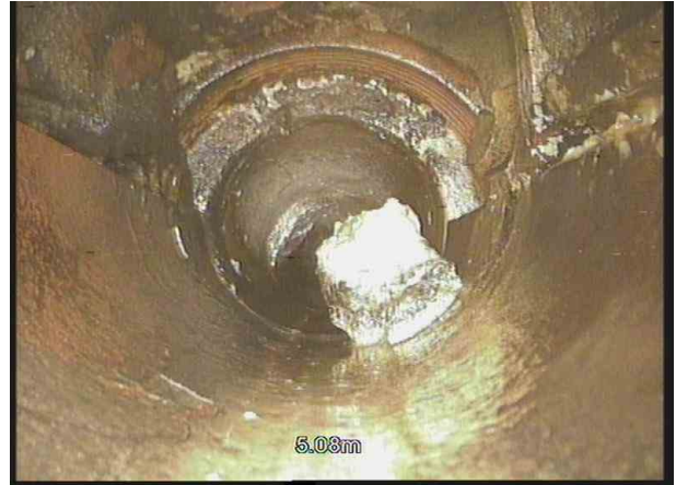
007.jpg, 00:00:40, 5.08 m Finish node type, manhole, reference number: IC3
