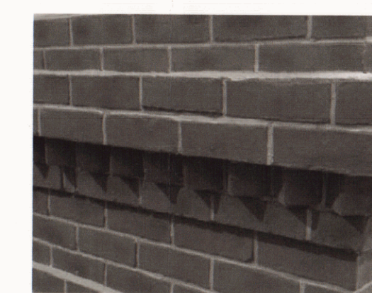
11 PROPOSED DENTAL BRICK DETAILS N.T.S.
