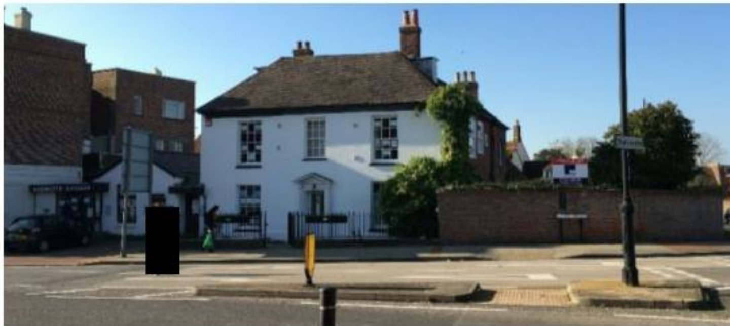
Plate 6: 6 North Street, principal east elevation.
