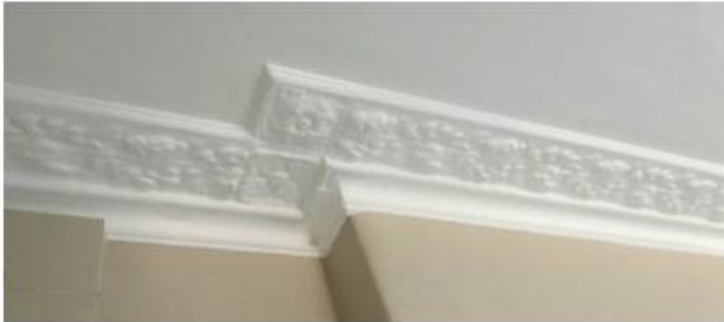
Plate 29: Decorative cornice, Room 3a.
