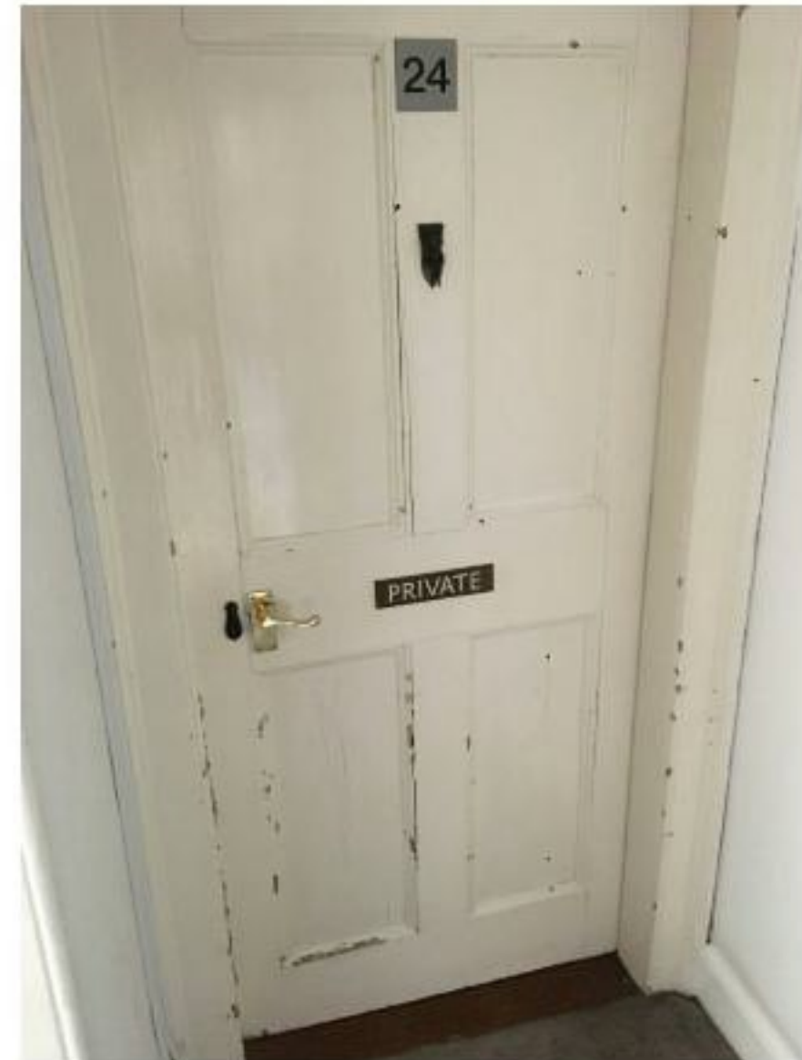
Plate 31: Door to Room 15 (labelled 24) from Room 11.
