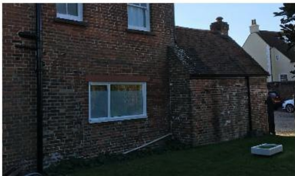
Plate 19: Single-storey extension at the west end of the north elevation and ground-floor window with concrete lintel.
