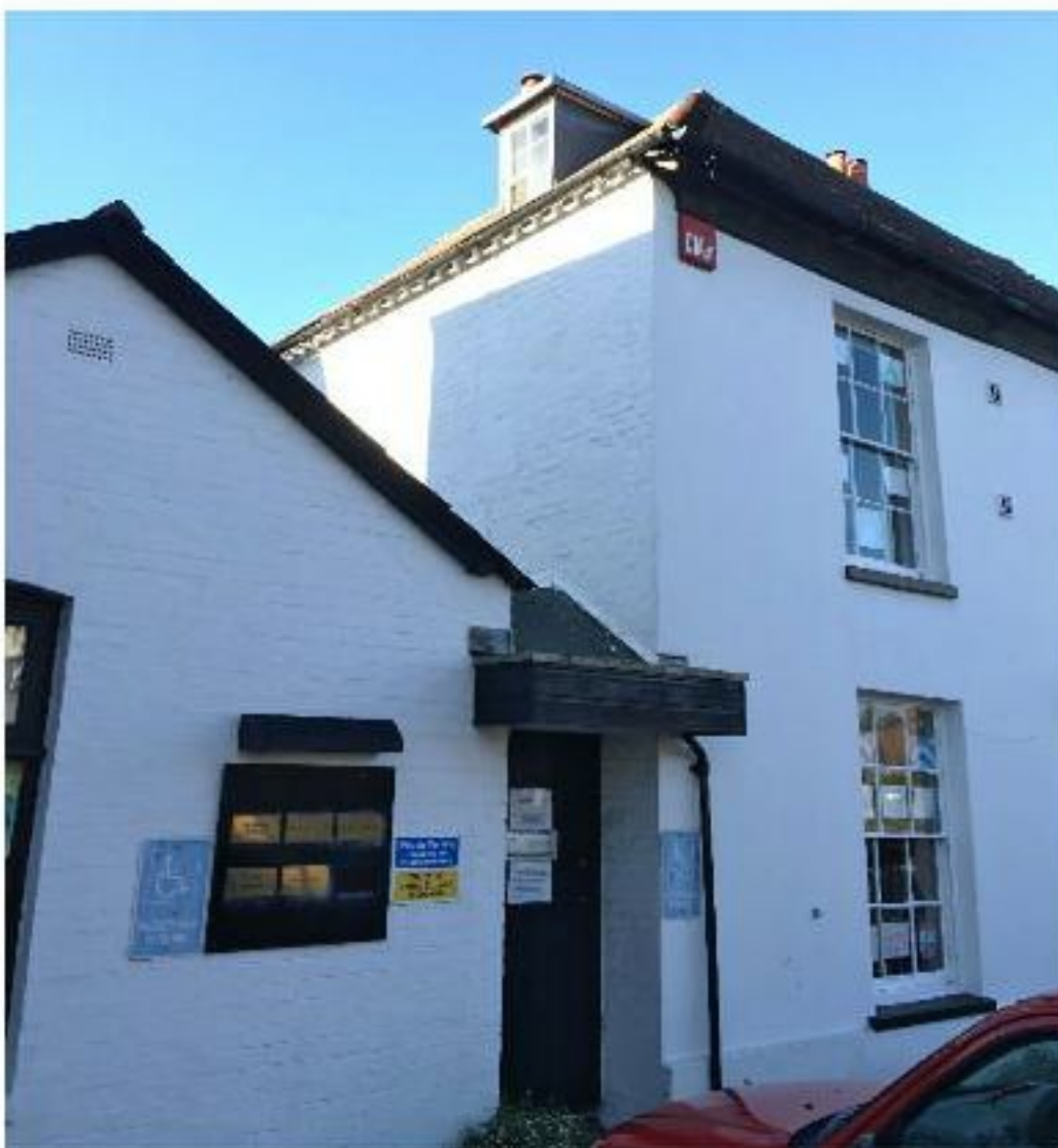
Plate 17: Detail of the join between the two-storey east façade and the single-storey extension.
