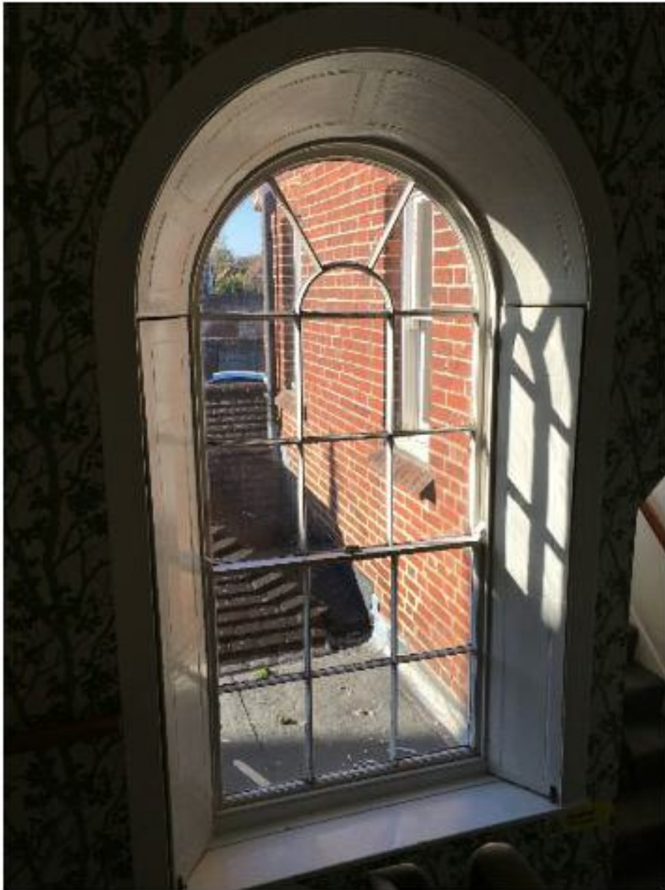
Plate 32: Window above the main staircase (Room 10).
