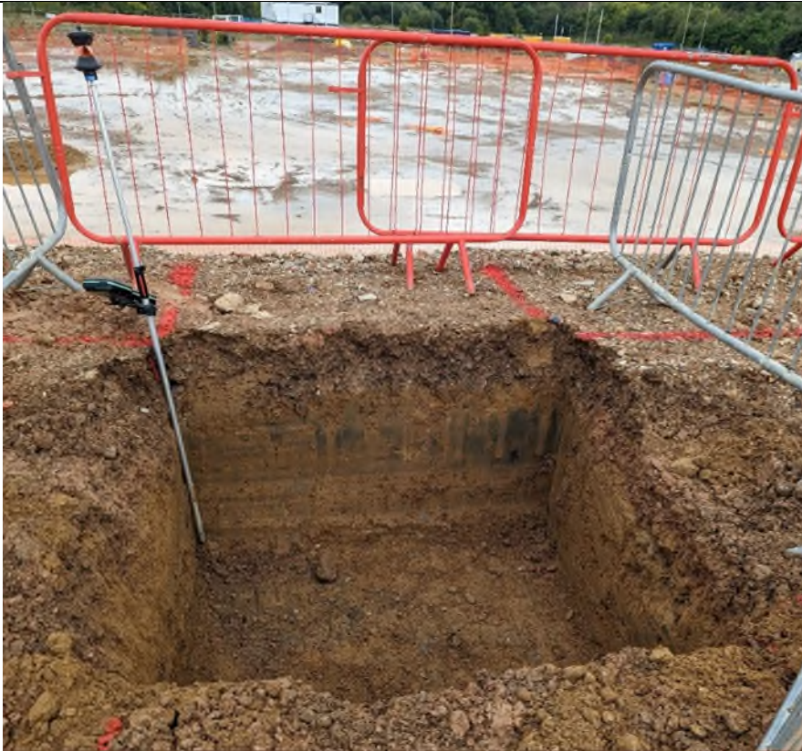
Photograph 8: Looking South over crest of 501
