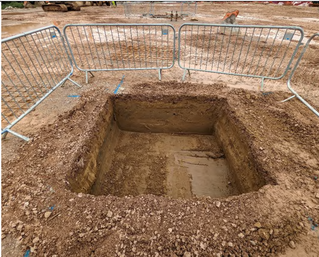
Photograph 4: Looking south along boundary over plot 501 towards 500
