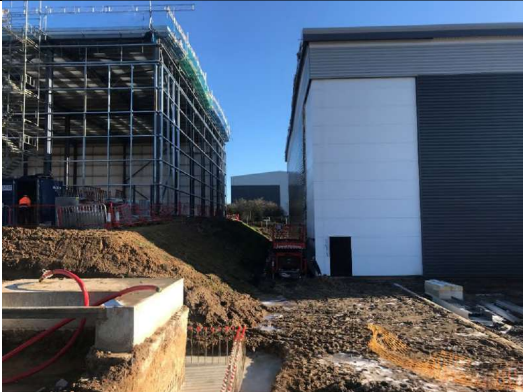
Photograph 1: Slope between Plot 500-501.
