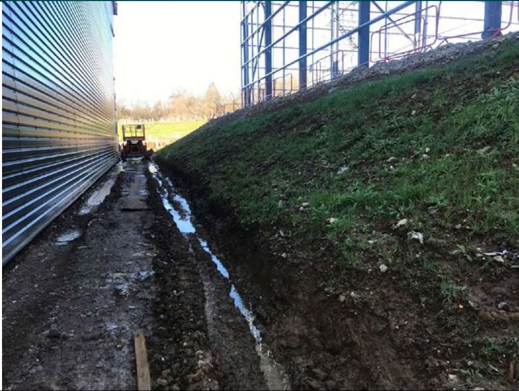
Photograph 3: Looking west across base of slope between Plot 500-501.
