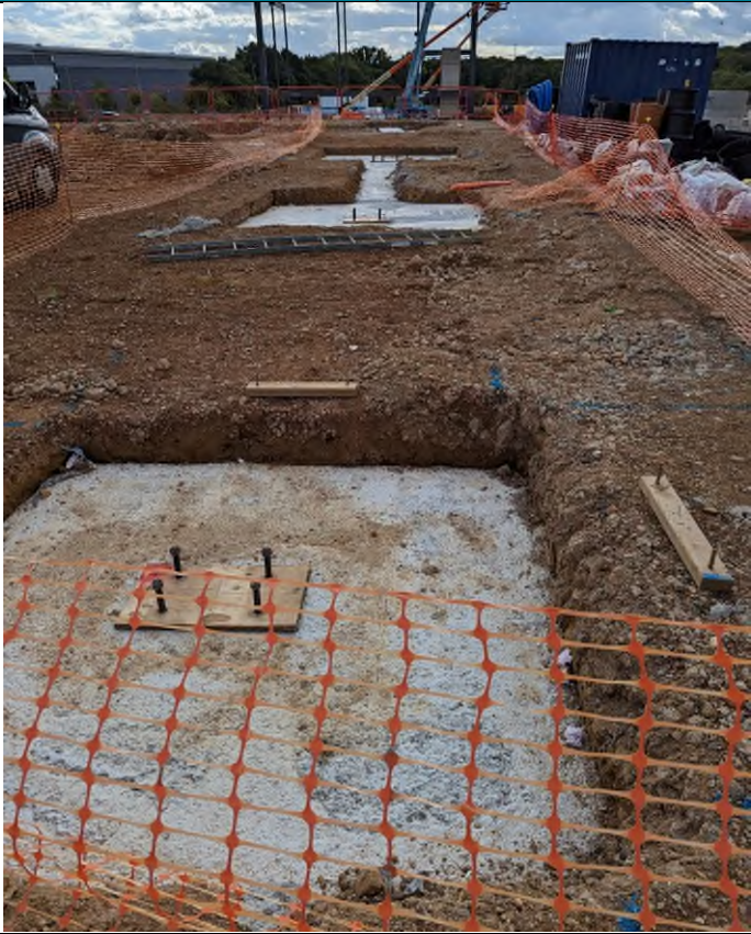
Photograph 3: Poured Footings along the western edge of Plot 501 and Looking South
