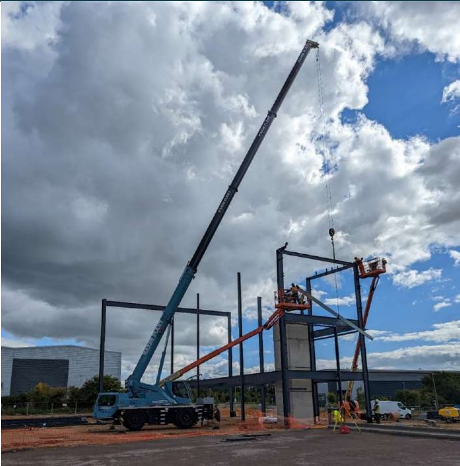
Photograph 1: Steel frame starting to be constructed on Plot 500
