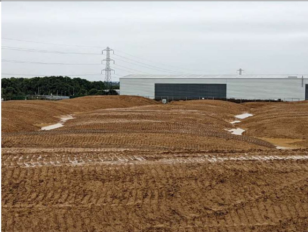
Photograph 13: Stockpile area looking south
