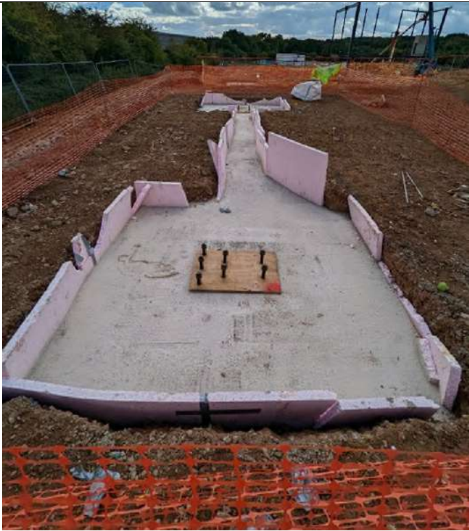
Photograph 4: Looking south along the eastern edge of Plot 501. Poured footings showing heave protection
