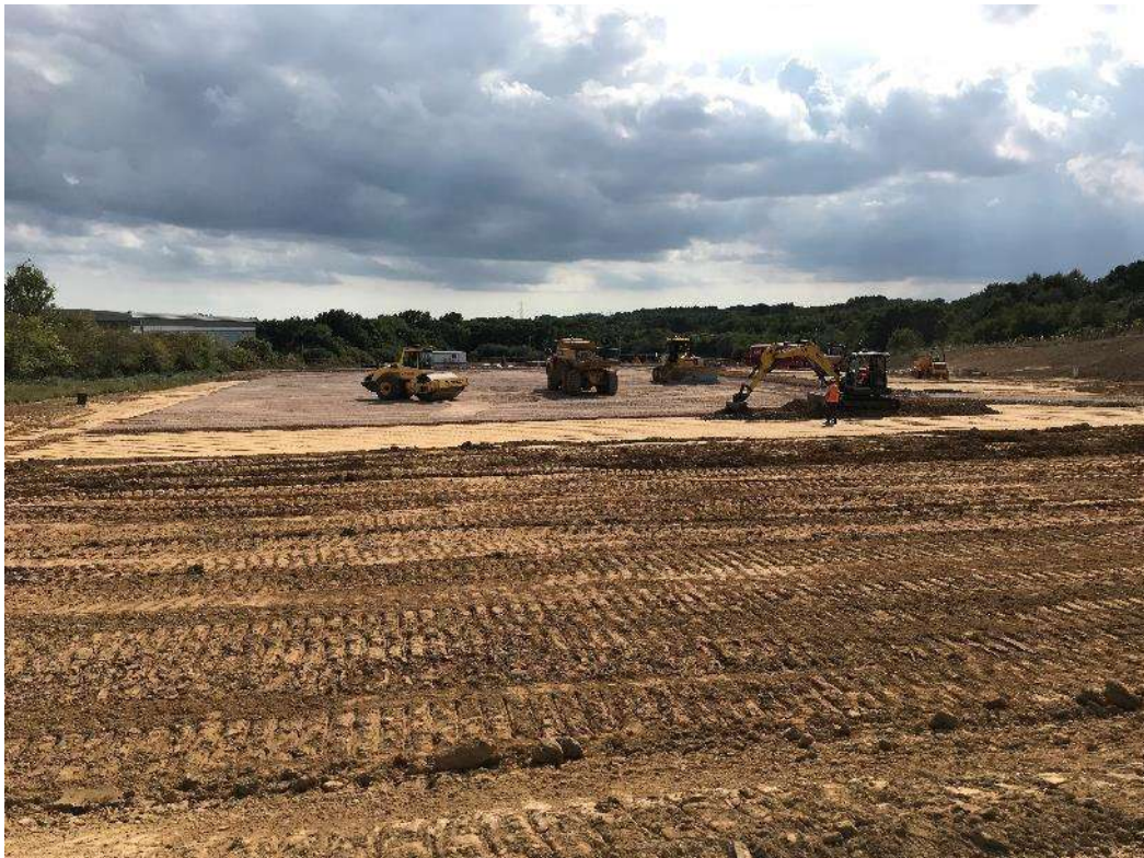
Photograph 2: Looking north across Plot 501 with fill being placed.
