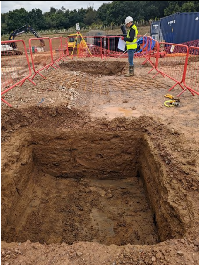
Photograph 9: Site surveyor confirming pad depths
