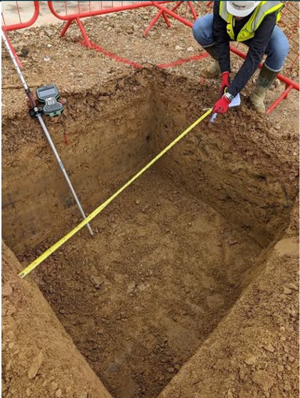
Photograph 7: Site surveyor checking pad depths on 501
