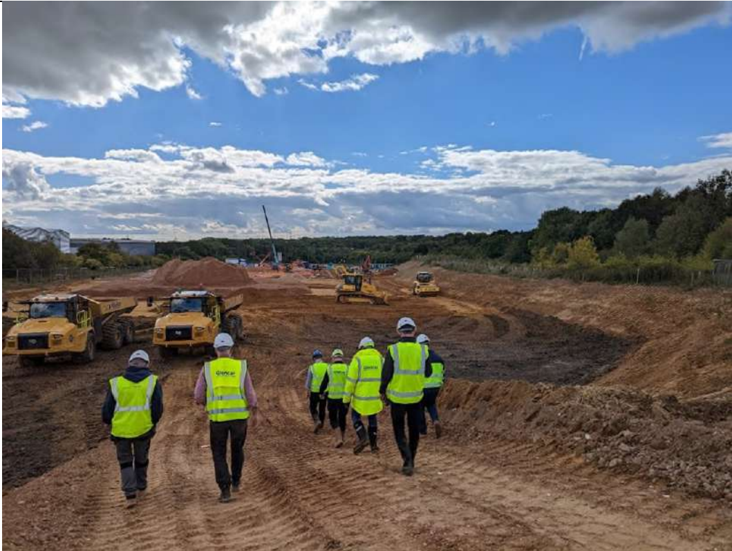
Photograph 8: Looking south from the access ramp to Plot 400
