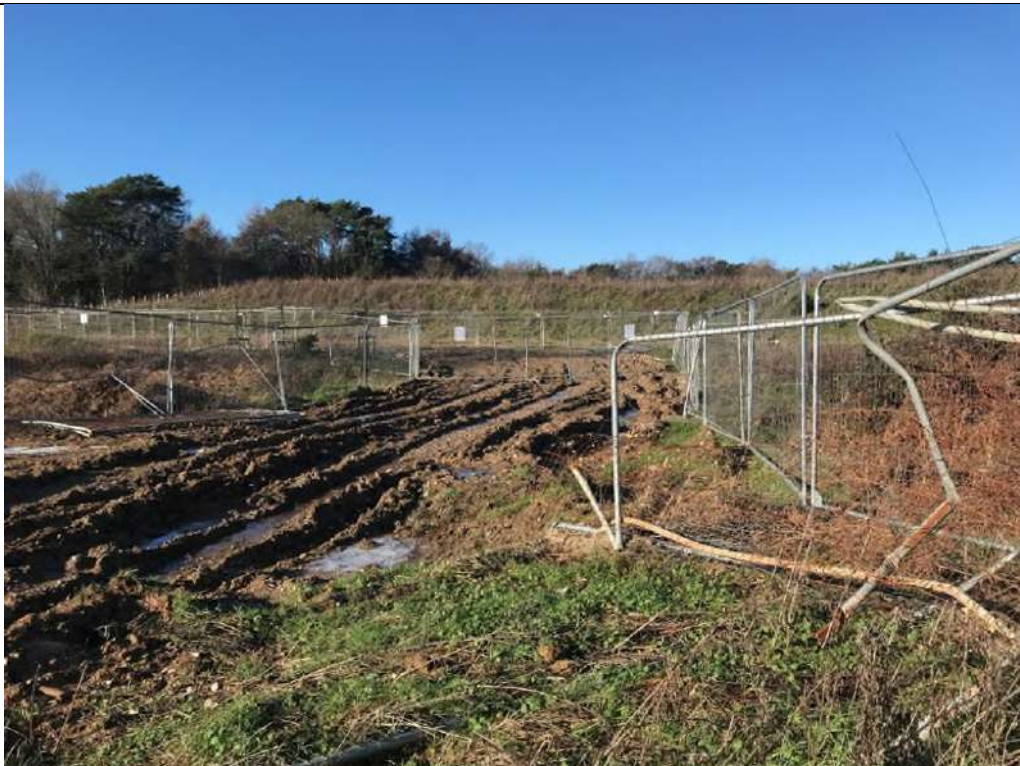
Photograph 6: Access to Plot 400 – very wet and soft ground.
