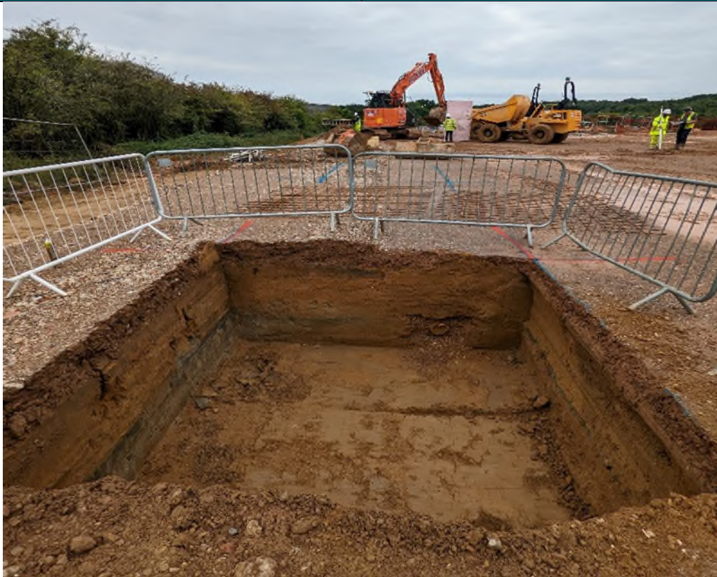
Photograph 3: Looking south along boundary over plot 501 towards 500
