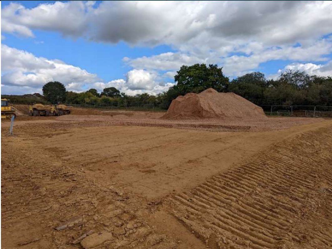
Photograph 11: Plot 501 – starting to place capping layer material
