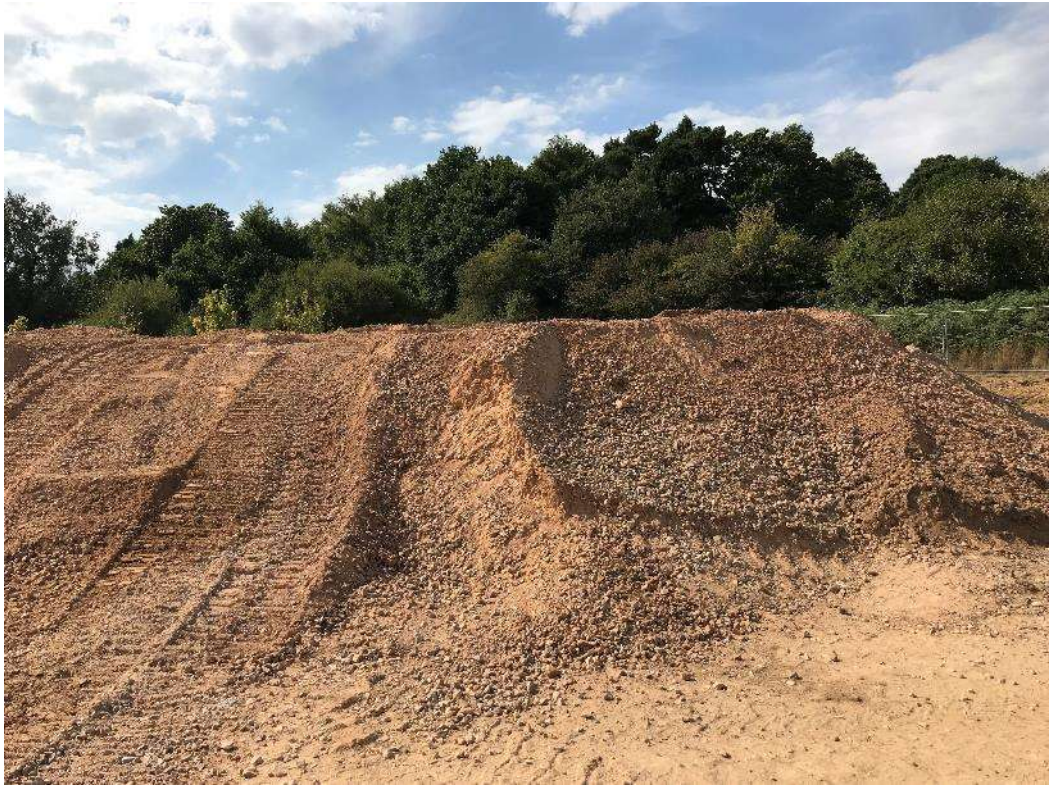
Photograph 4: Stockpile of site won aggregate in NW of Plot 502.
