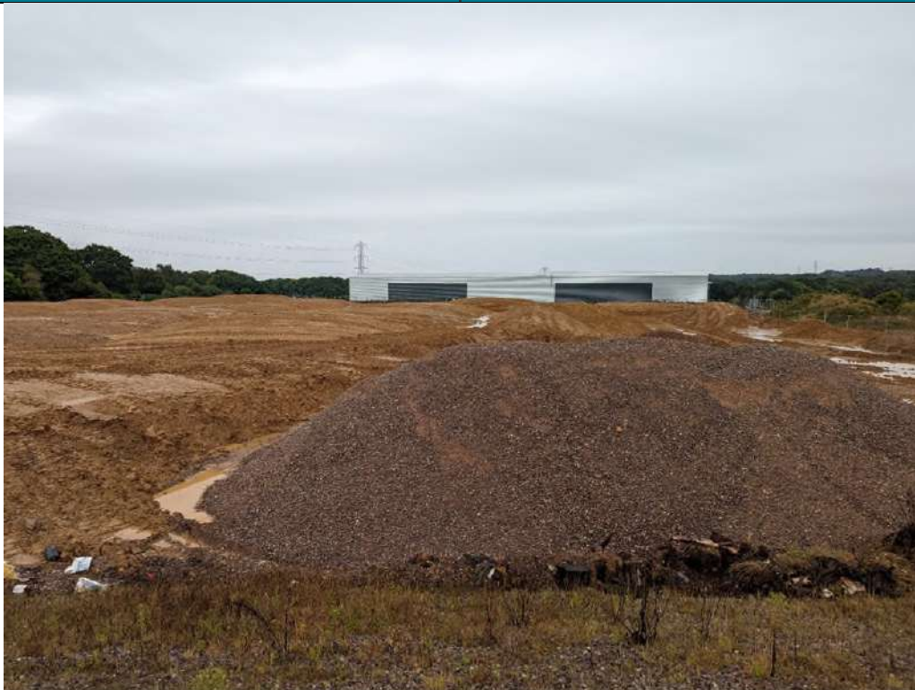
Photograph 12: Stockpile area looking south – Type 1 / Class 6 material in foreground:
