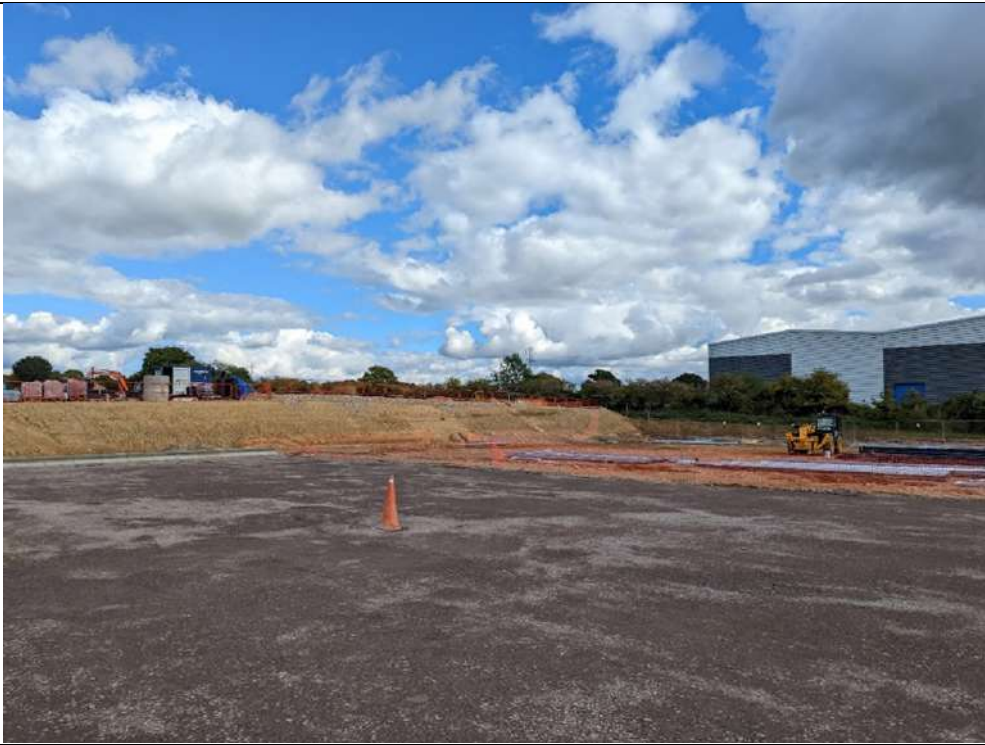
Photograph 2: Looking NE across the top of plot 500 and towards the Plot 501 berm
