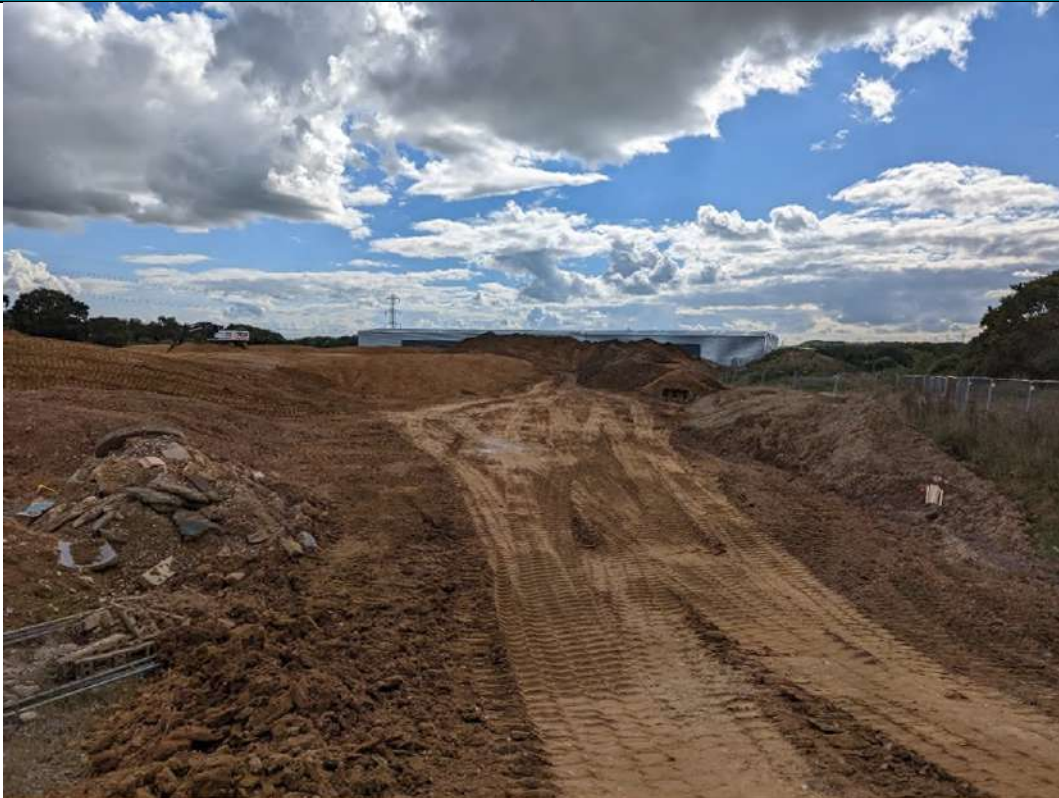
Photograph 9: Plot 400 Looking from access road entrance and south
