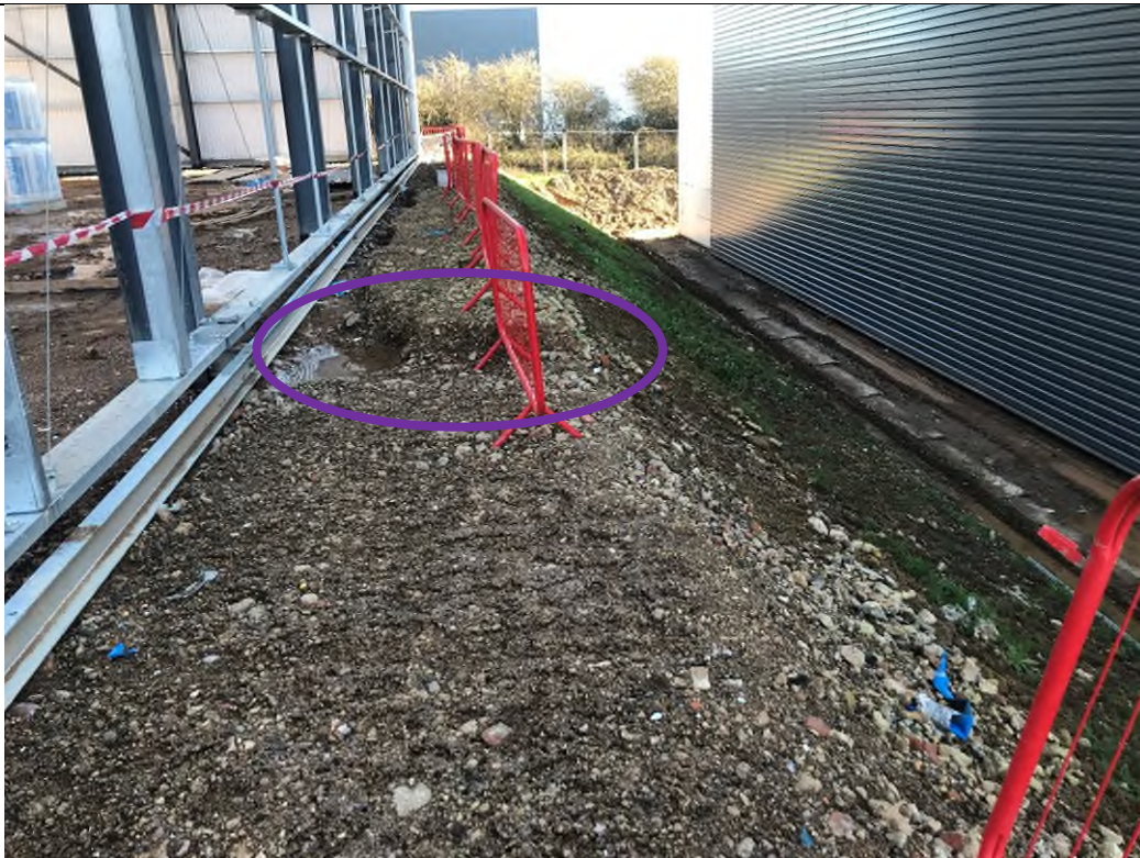
Photograph 2: Looking east across the top of slope between Plot 500-501. Dewatering trench circled.
