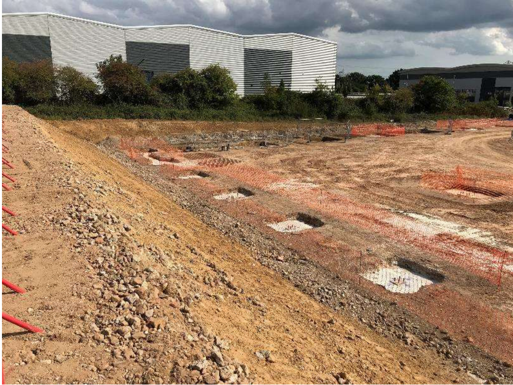
Photograph 1: Looking south east across Plot 500 with new pad foundations.
