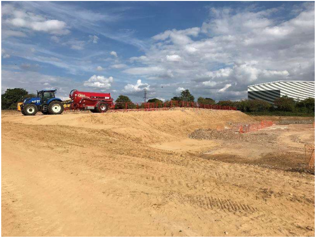
Photograph 3: Tractor and bowser for dust mitigation.
