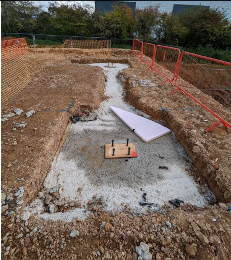
Photograph 5: SE Corner Plot 501 with berm to the right – note closeness of footings to berm edge
