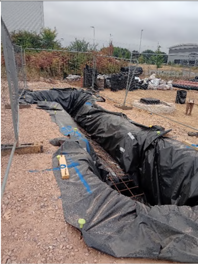
Photograph 2: Plot 500 footing inspection
