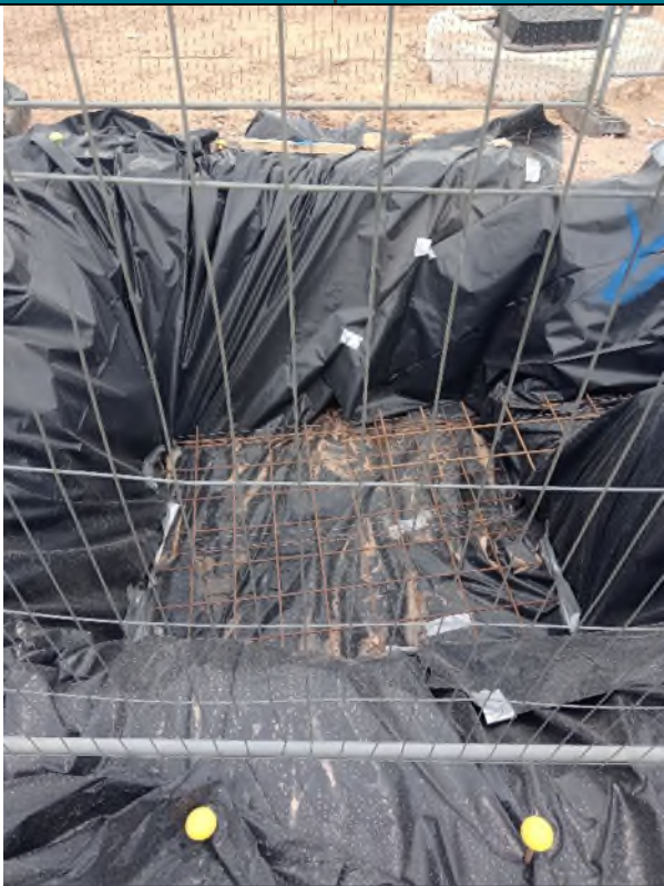
Photograph 3: Plot 500 footing showing protection
