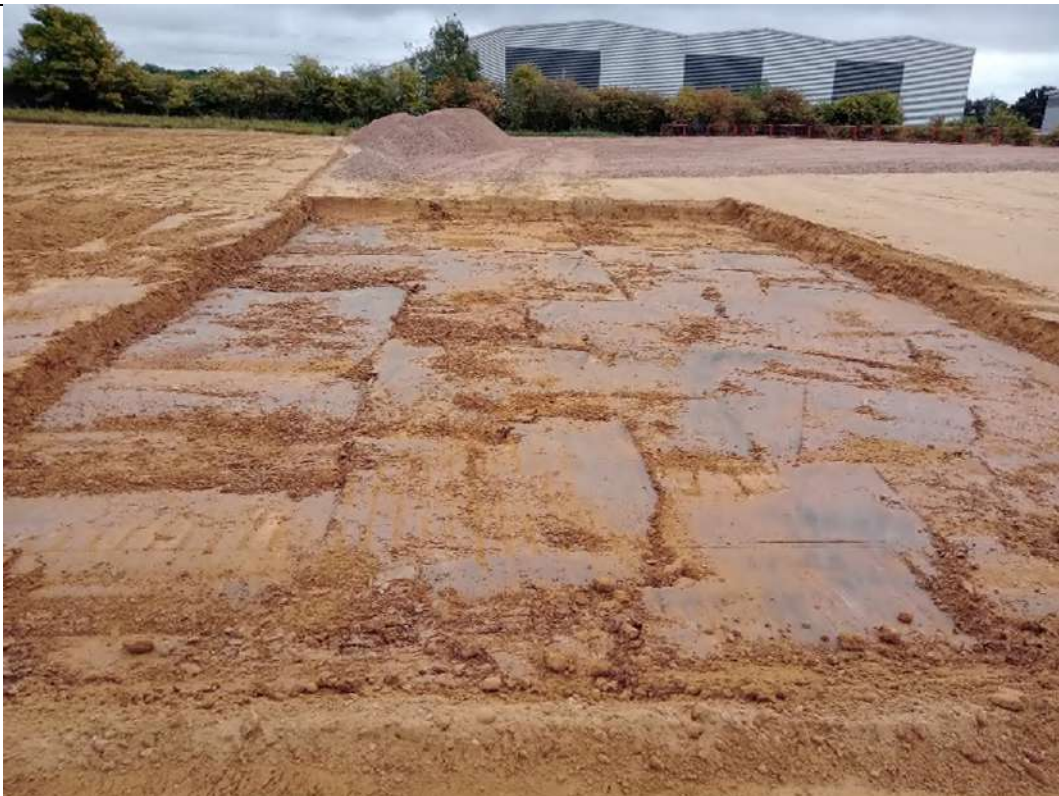
Photograph 16: Plot 501 - Clay prior to being tested before fill placement – looking towards eastern boundary
