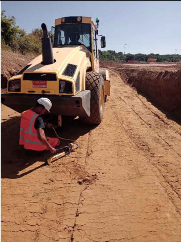
Photograph 7: Contact technician carrying out plate load tests
