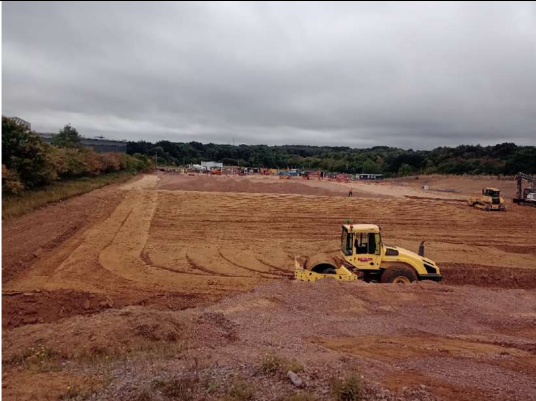
Photograph 15: Overall view looking over 502 towards 501 and 500 (South)
