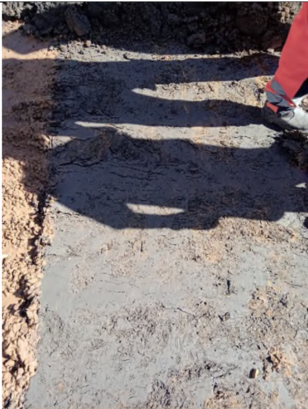
Photograph 2: Clay subgrade on proposed compaction trial area
