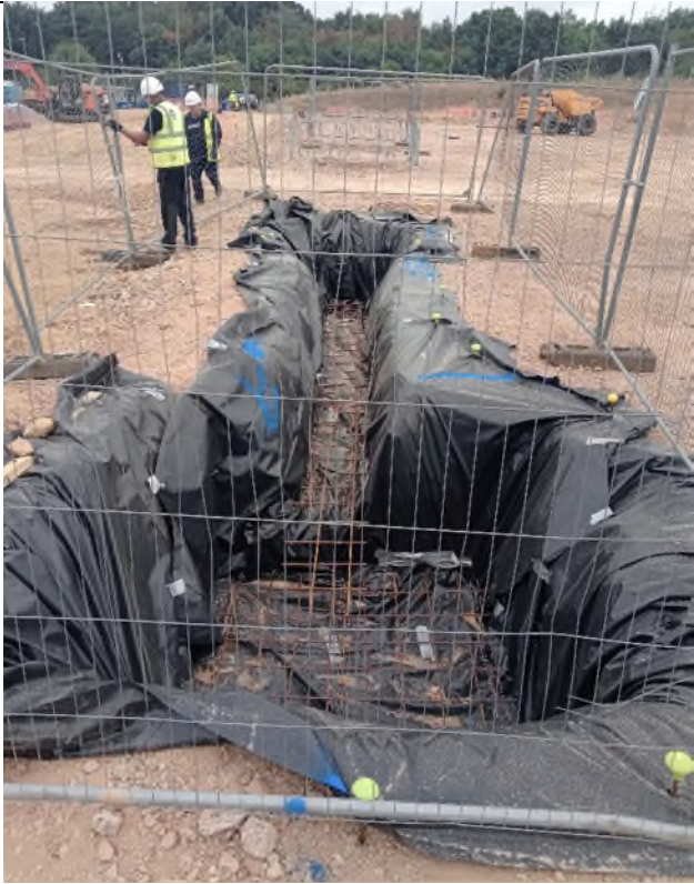
Photograph 4: Pre excavated and footing being protected from weather
