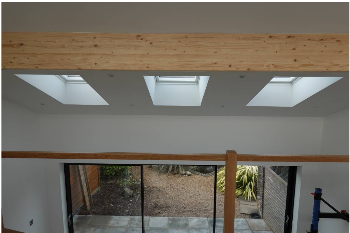
Photo 6 – View with back to south-east wall of mezzanine looking into the room. The only views into the building from outside would be the sloped ceiling and possibly the timber beam.
