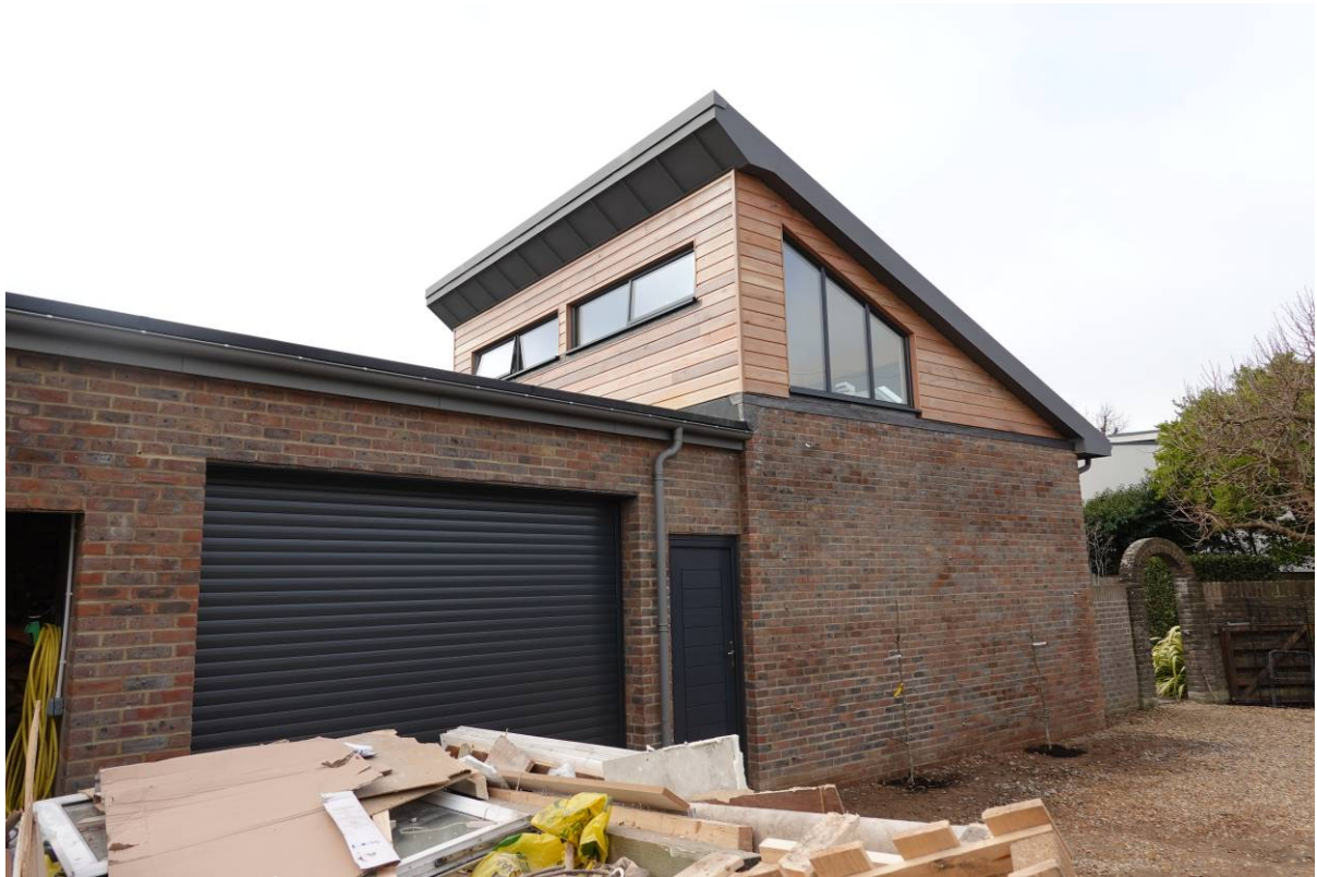
Photo 1 –View of gymnasium & garage nearing completion showing high level south-east facing windows to the mezzanine floor.
