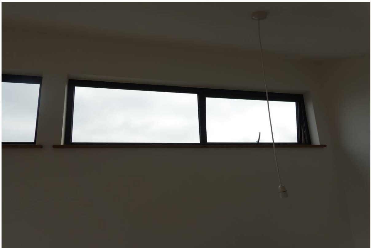
Photo 2 – View through windows standing at the far edge of the mezzanine floor (by 6ft adult). It should be noted that only the sky can be seen with no view whatsoever of the adjoining properties.
