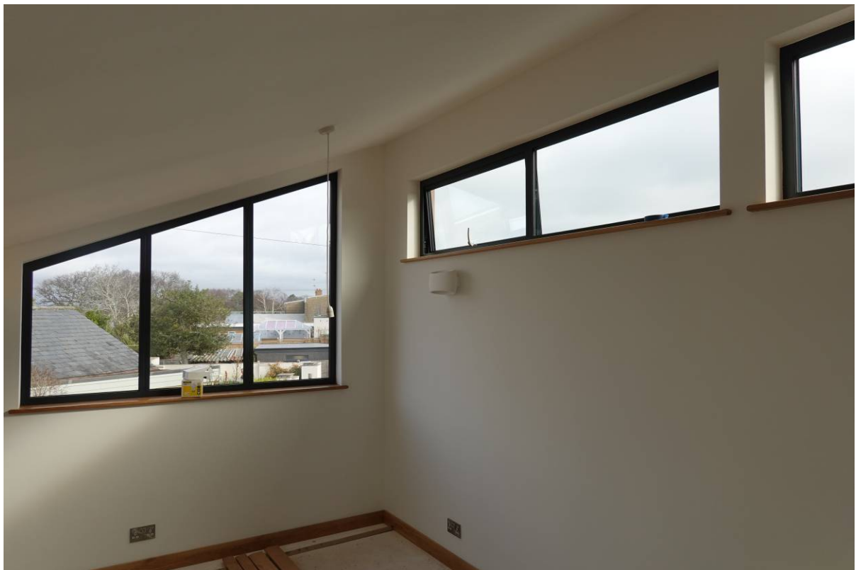
Photo 4 – View of mezzanine windows looking north-east and south east respectively.
