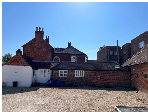
The rear elevation of the subject premises and parking area.
