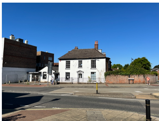
The site viewed from the east, on High Street.
