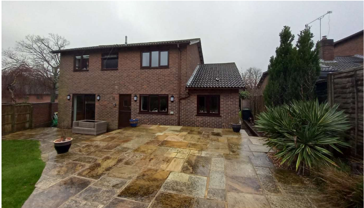
Photograph showing rear of 3 Riverdale Avenue
