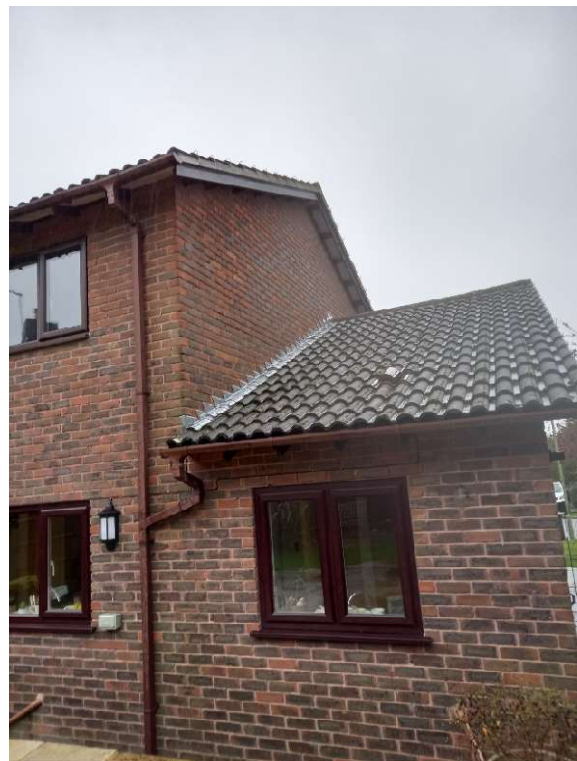
Rear view of footprint to be extended
