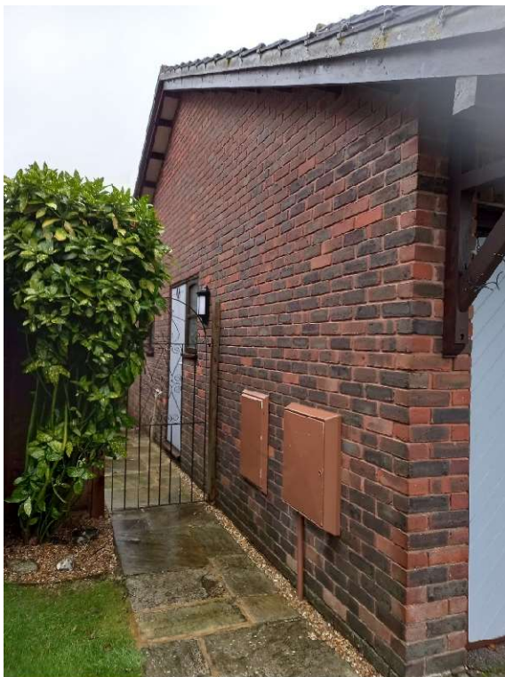
Side view of existing garage from front
