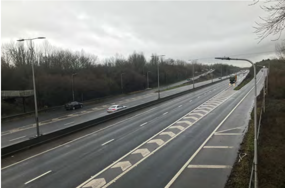
Figure 16: View south west from pedestrian bridge over A27 looking toward northern boundary of the Site
