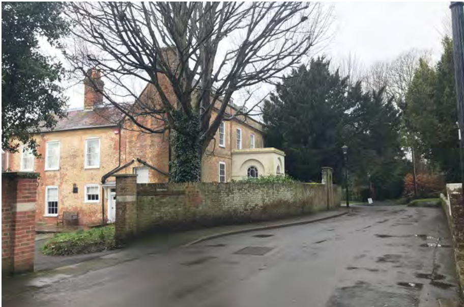
Figure 18: View west on Bidbury Lane to Grade II Old Rectory (NHLE ref.1091648) positioned opposite church of St Thomas.
