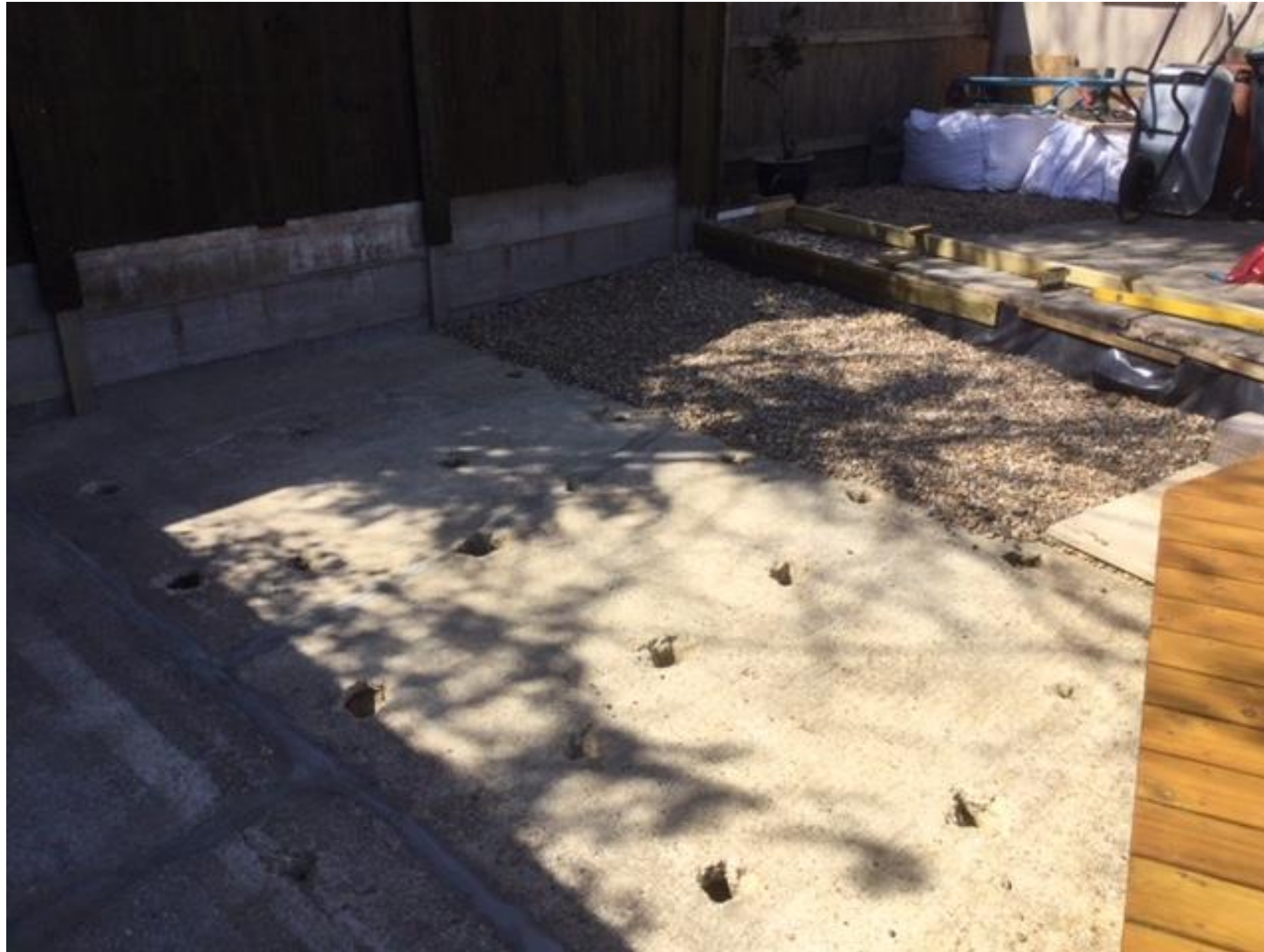
Figure 1. Showing rear garden once uncovered by Mr Wragg, found concrete slab when investigating newly bought land.
