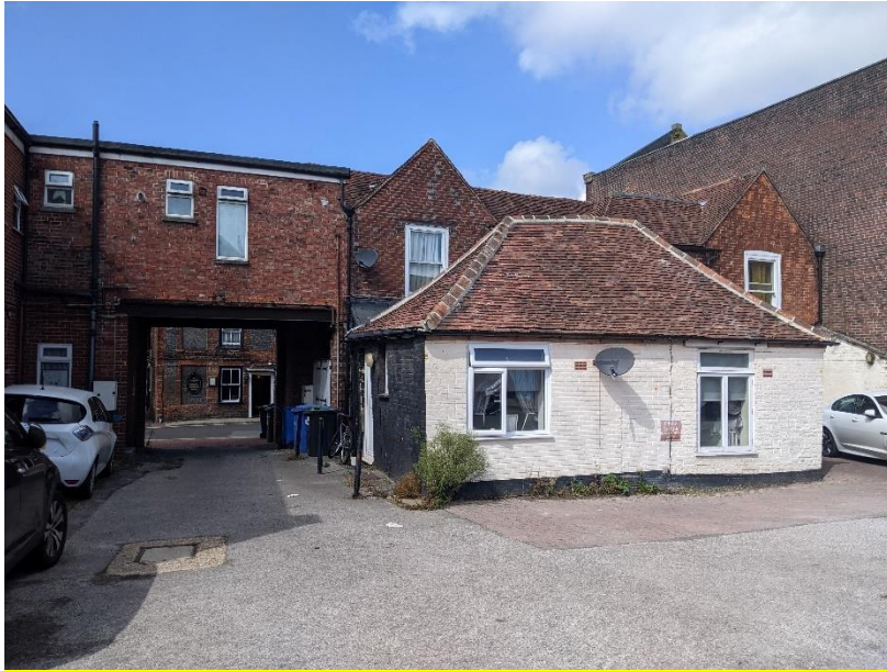
Figure 11: Rear of no.13 South Street as seen from the courtyard area. Here the rear gable ends of the original part of the building are still visible behind a rear extension.
