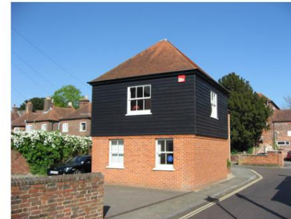
Figure 58: Weatherboarding used effectively in new building in the conservation area (Homewell)
