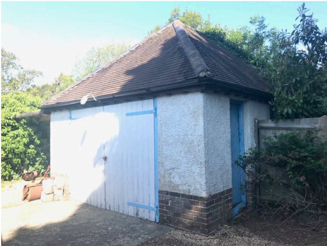
Figure 6. Garage set for demolition.
