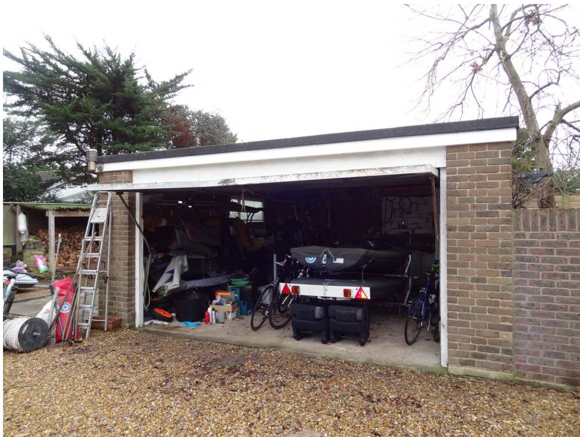
Photo 1 –View of existing garage to be demolished.
