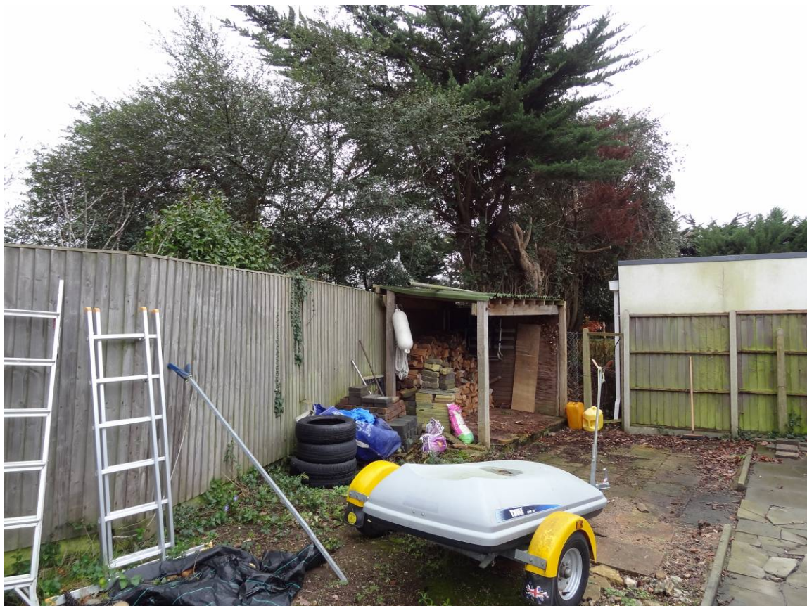
Photo 4 – View of south-east boundary on left with existing log store to be removed..
