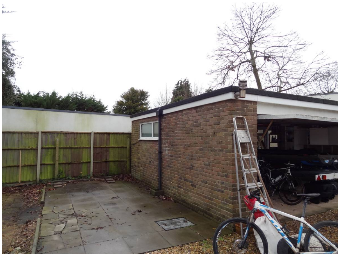
Photo 3 – View of south-east end of existing garage. Adjoining garage to no. 13 beyond.
