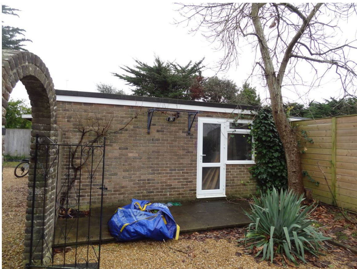
Photo 2 – View of existing garage north-west elevation from courtyard.
