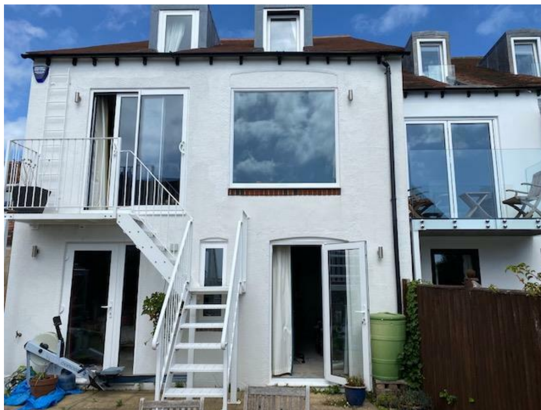
Image 2 Rear: Number 4 to the east of the site (right) with recently approved first floor balcony overlooking number 5's rear garden.
