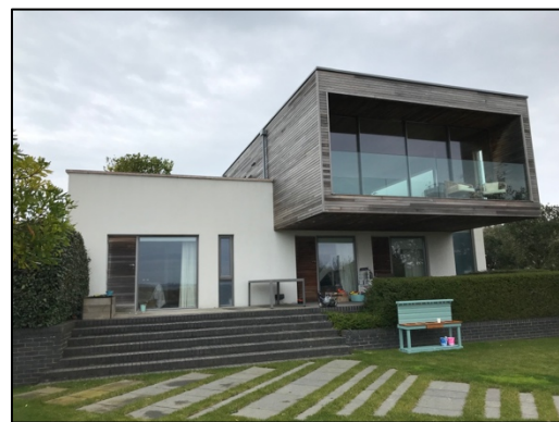
Figure 6 – eastern elevation of the house
