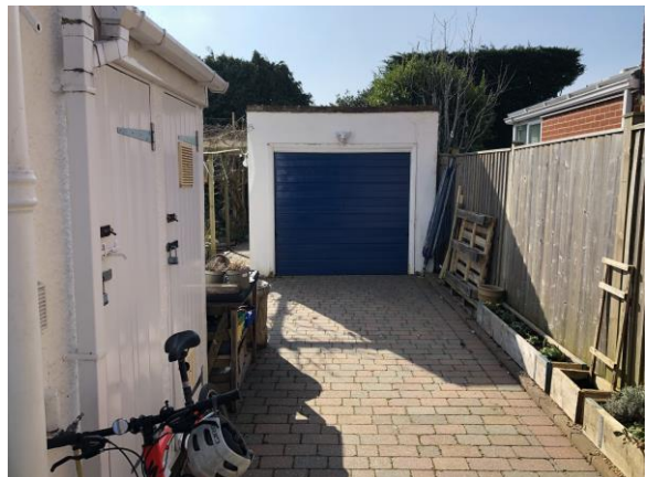
Figure 9: North elevation of garage
