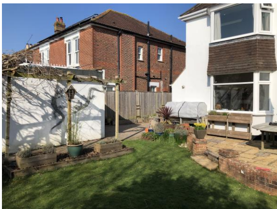
Figure 8: Side view of rear elevation and garage
