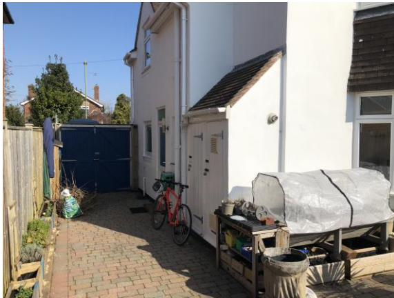
Figure 6: Side access to garden
