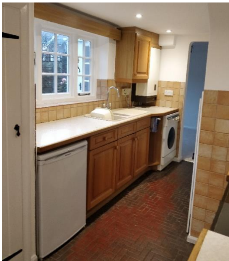
Existing kitchen and rear wall
