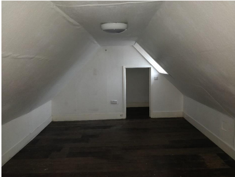
Second floor loft room – flat section of fibre board ceiling to be removed.
