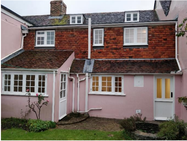
Figure 4: Rear Elevation of dwelling
