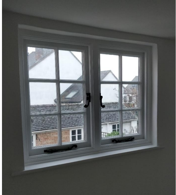
Existing landing window to be repositioned and replaced.
