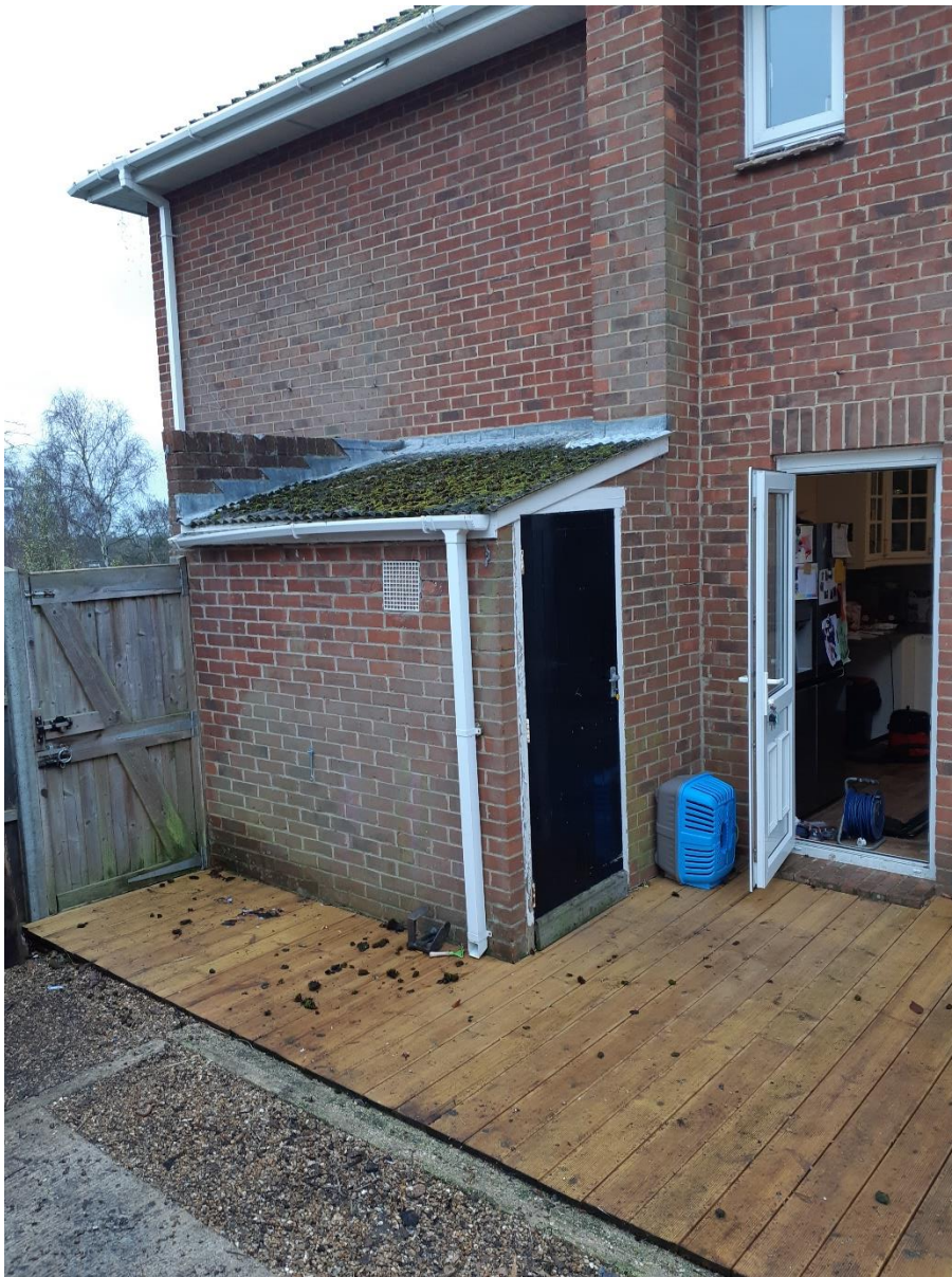
Photo 7: Rear of property
