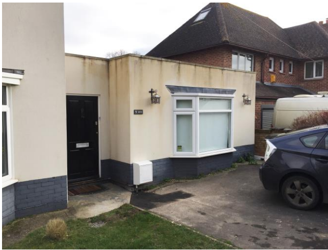
Figure 4: Existing flat roof extension
