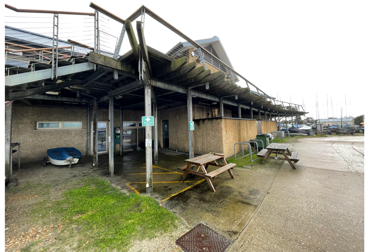
View onto existing unused space underneath balcony of main building on site.
