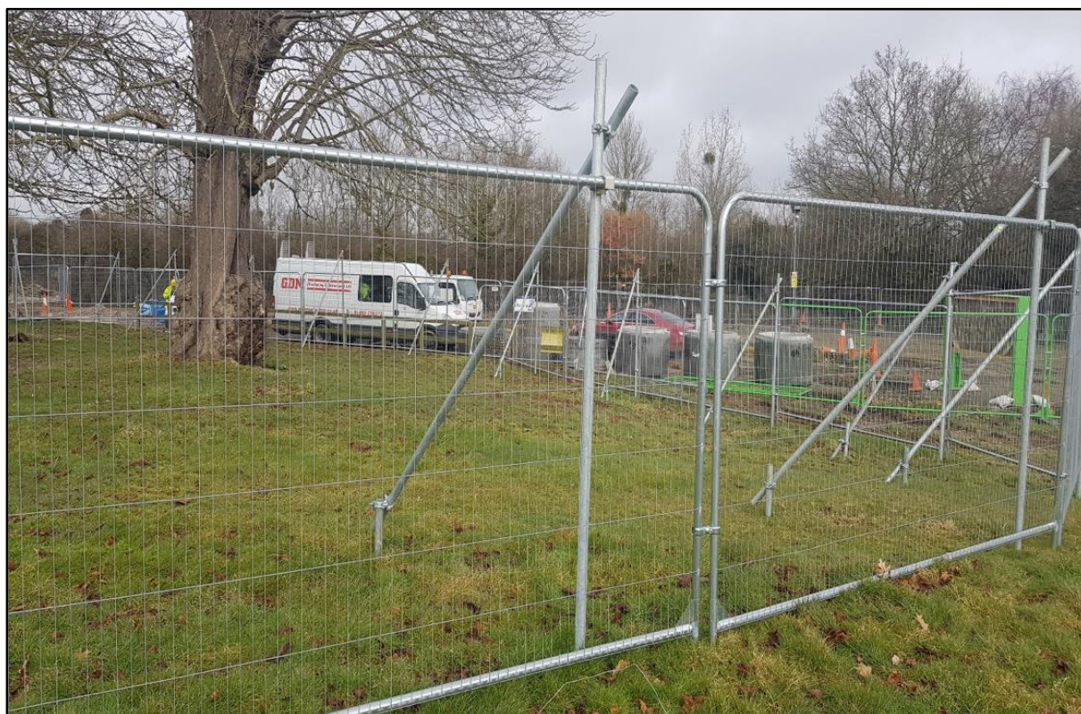
Specification agreed by LAP Tree Officer tree protection fencing
